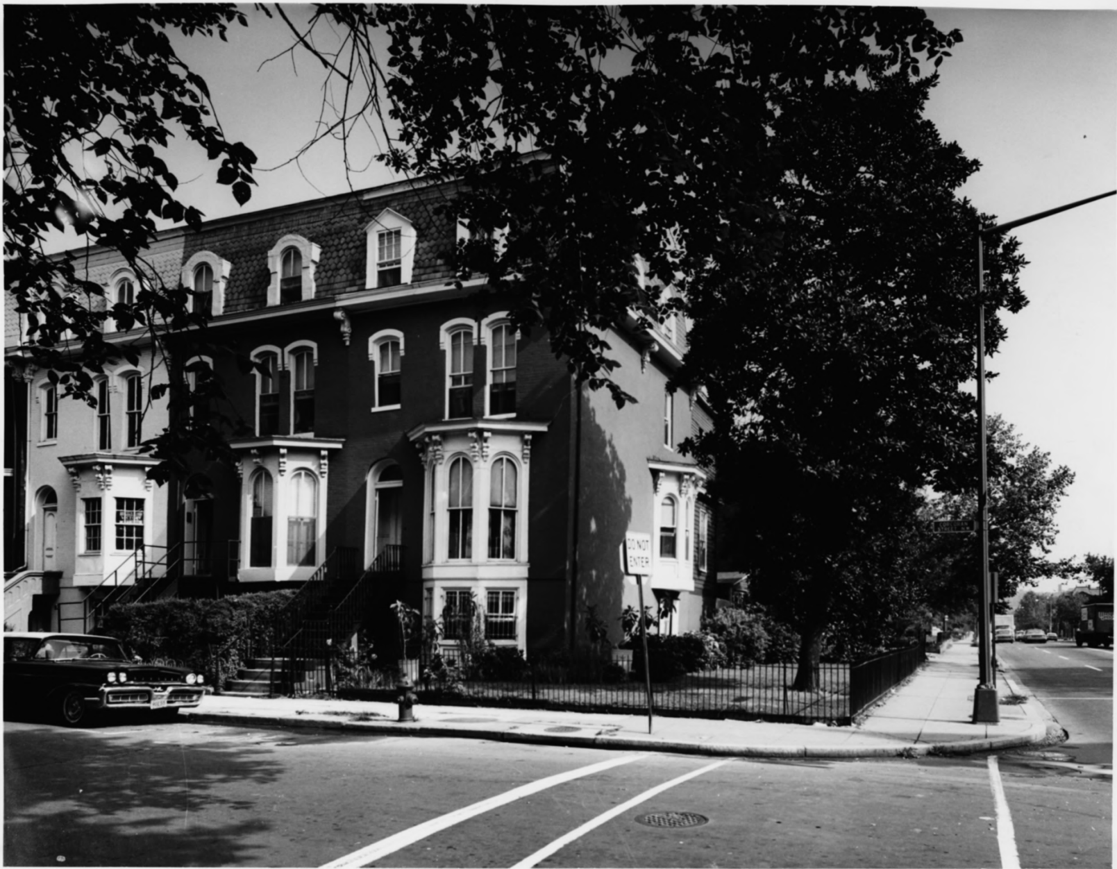
Zalmon Richards House - 1301 Corcoran Street, NW., - National Park Service Photo, 1965.
