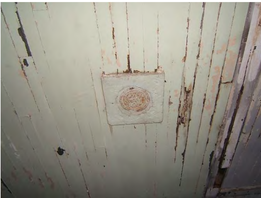
Photo 12a: Chimney thimble in ceiling
