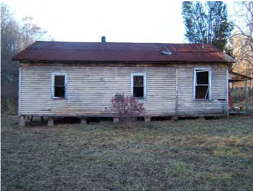
Photo 4: East Elevation, facing west.
