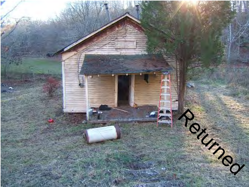
Photo 1: North Elevation, facing south.
