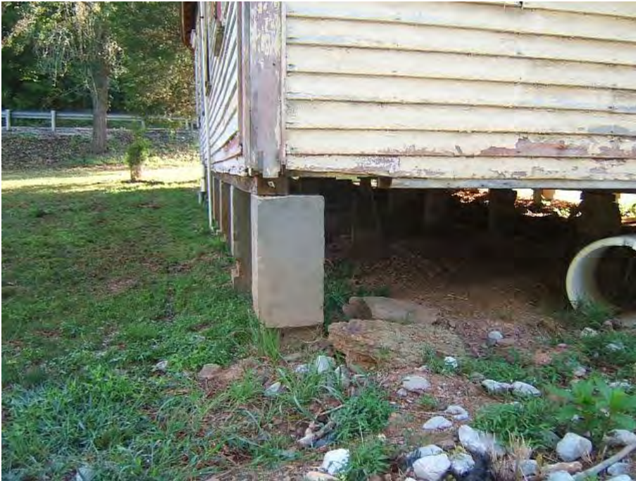
Photo 9: Pier detail south elevation, west elevation corner
