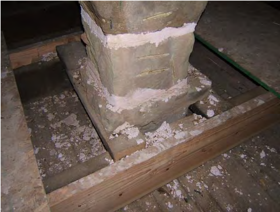
Photo 12b: Chimney thimble in attic
