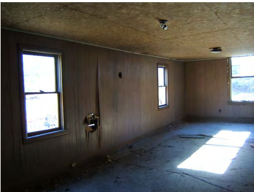
Photo 6: Interior, Classroom, southeast corner, facing southeast.
