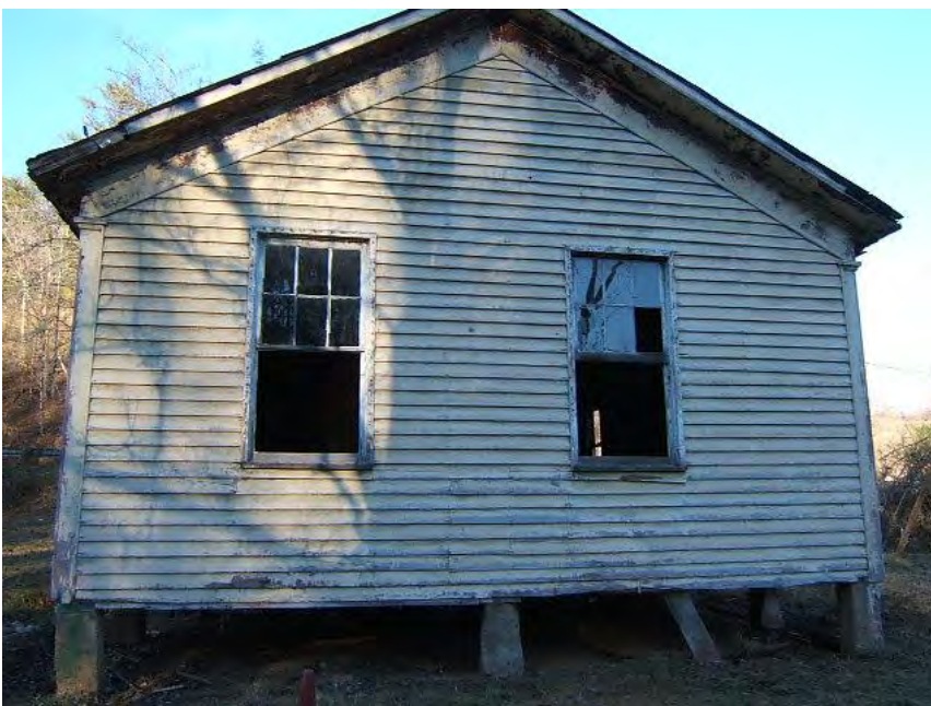
Photo 2: South Elevation, facing north.
