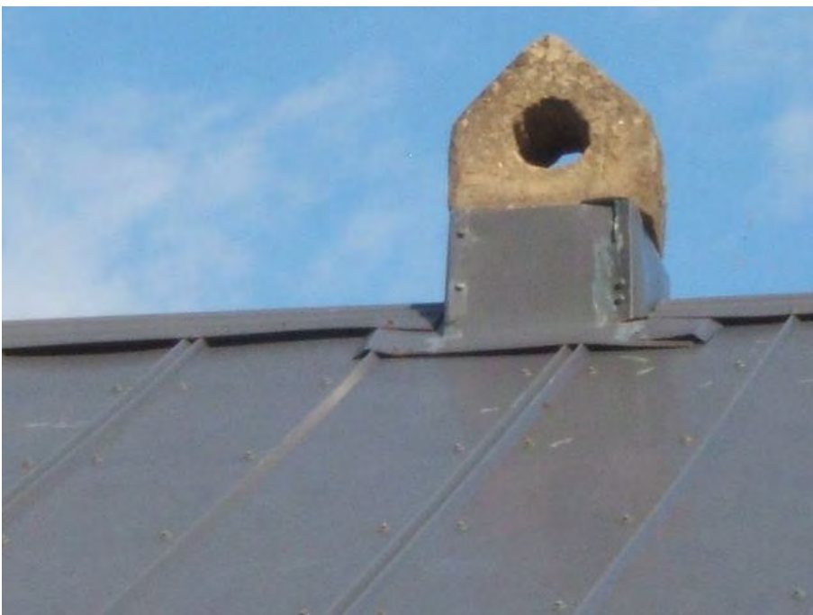
Photo 13: Chimney cap facing west
