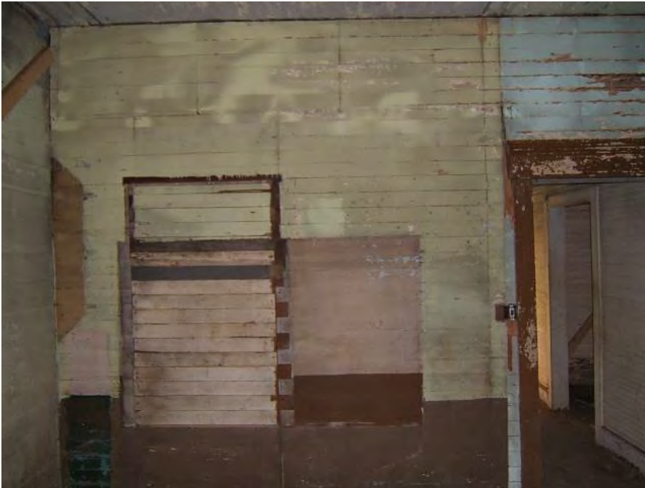
Photo 7: Original bead board/trim, corner at classroom/kitchen wall facing north
