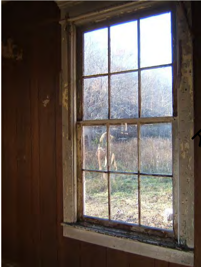
Photo 10: Interior, 6/6 double-hung window, facing west.
