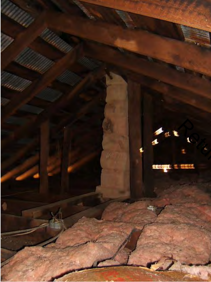
Photo 11: Interior, Attic, Chimney stack, facing south.
