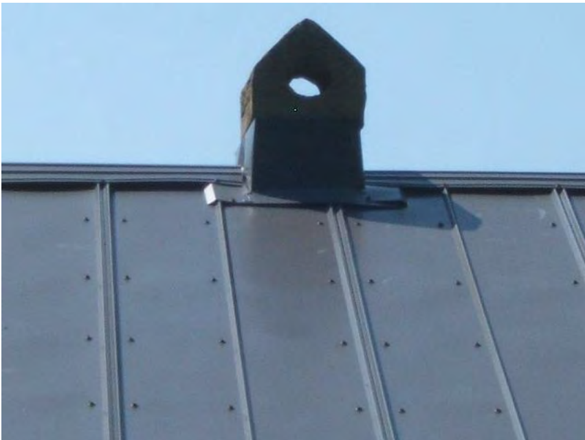
Photo 13: Exterior, Chimney Cap on Roof Ridge, facing west.
