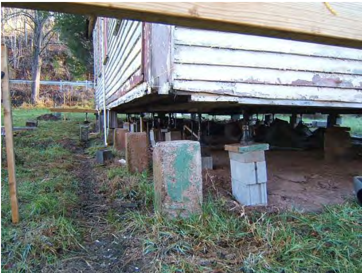
Photo 9: Pier, Detail, Southwest corner, facing northeast.
