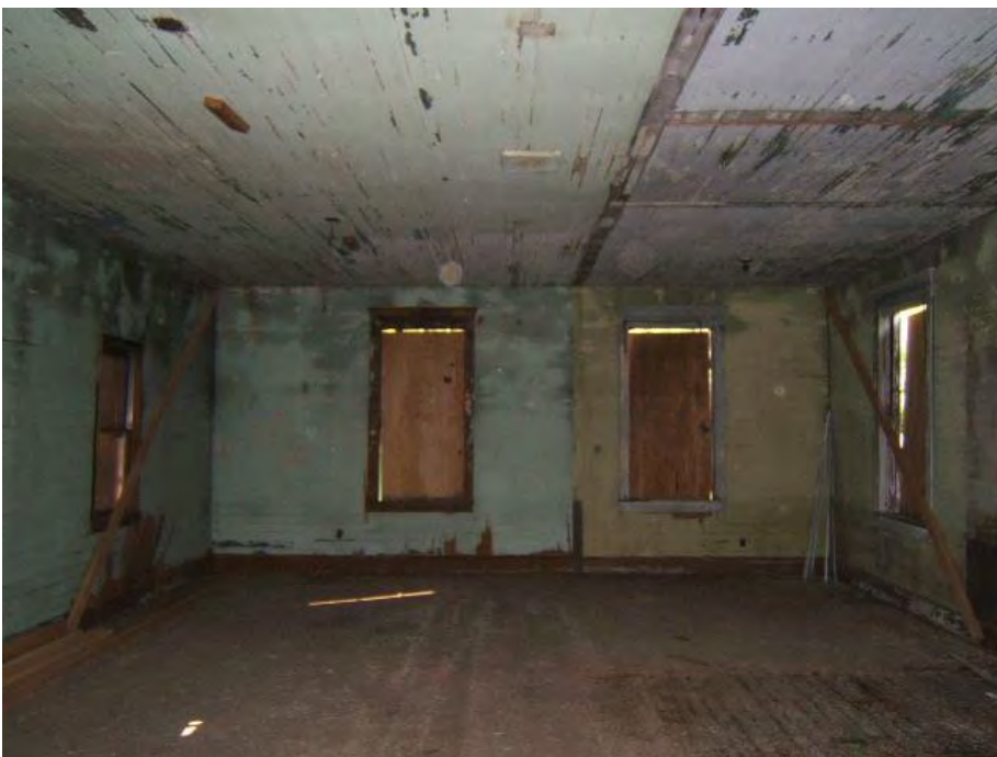
Photo 6: Classroom facing south elevation
