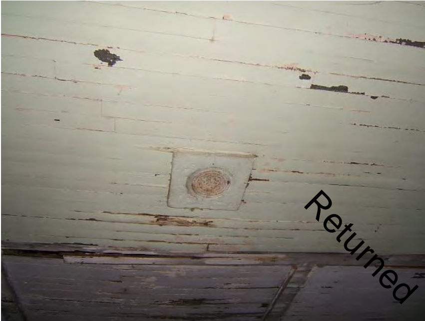
Photo 12: Interior, Ceiling detail, Chimney Thimble, facing skyward.
