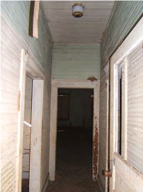
Photo 11: Foyer, front entry facing south elevation
