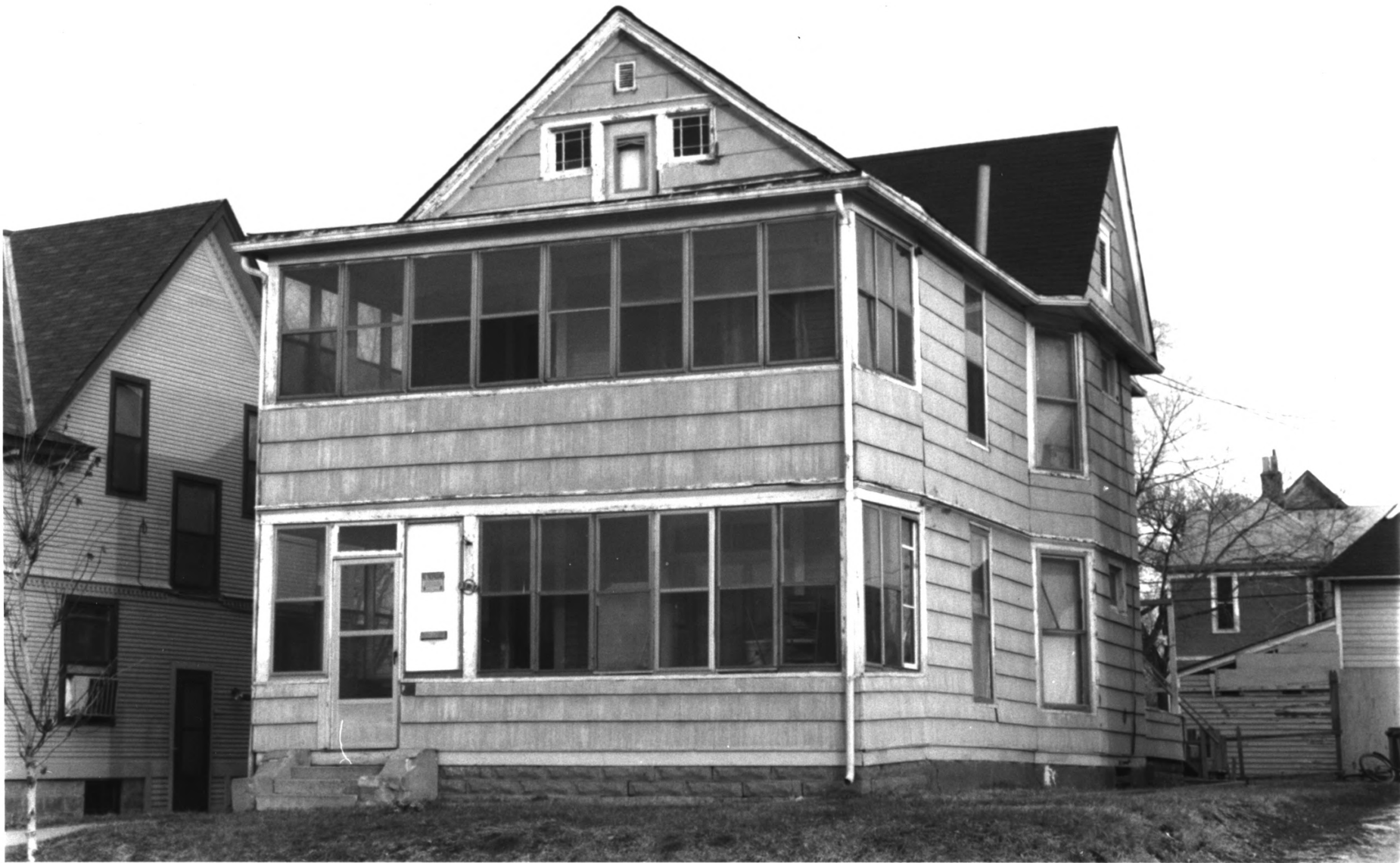
HEALY-FORBES HOUSE - 3137 2ND AVE. S. HEALY BLOCK HISTORIC DISTRICT MINNEAPOLIS, HENNEPIN CO., MINNESOTA #011476-22
