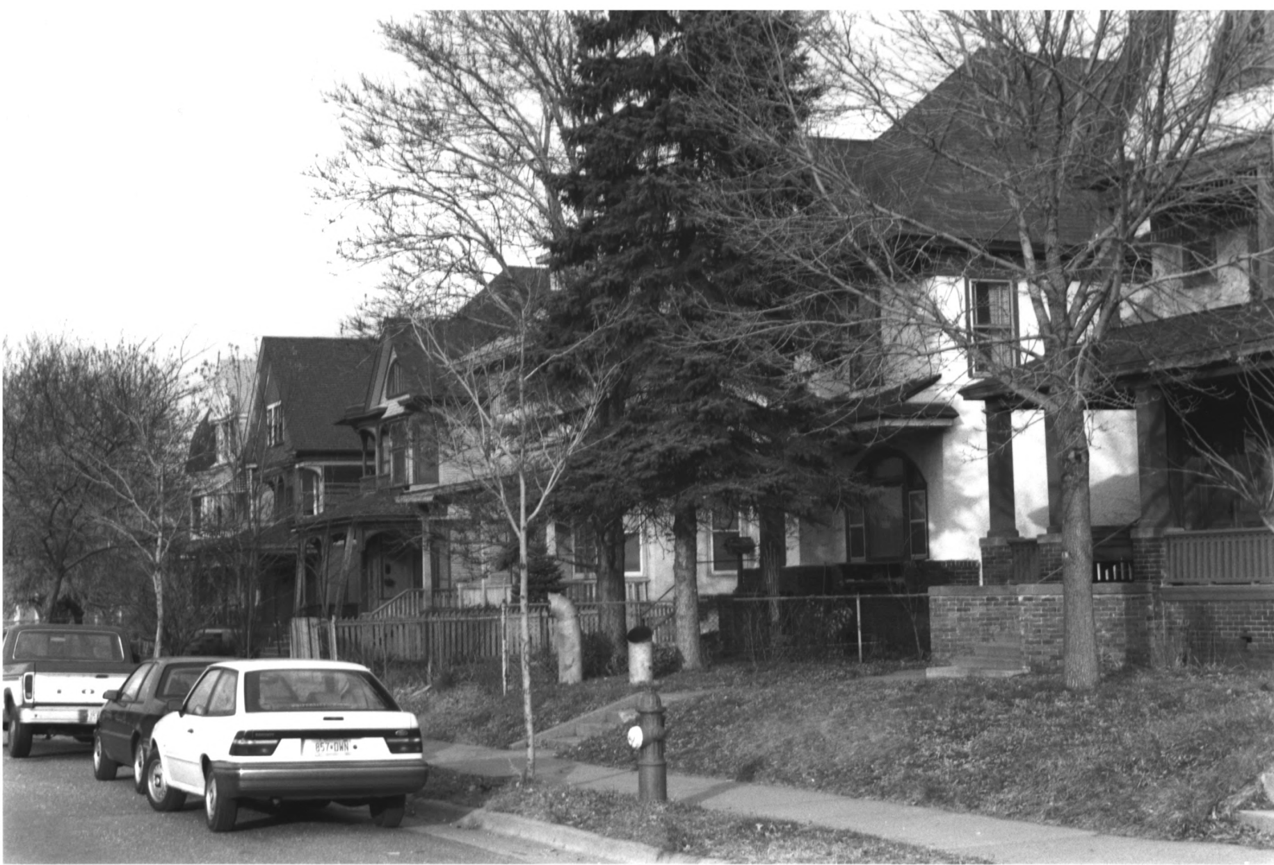
STREET SCAPE — 3111 - 3123 2ND AVE. S. HEALY BLOCK HISTORIC DISTRICT MINNEAPOLIS, HENNEPIN COUNTY, MINNESOTA # 011476-17
