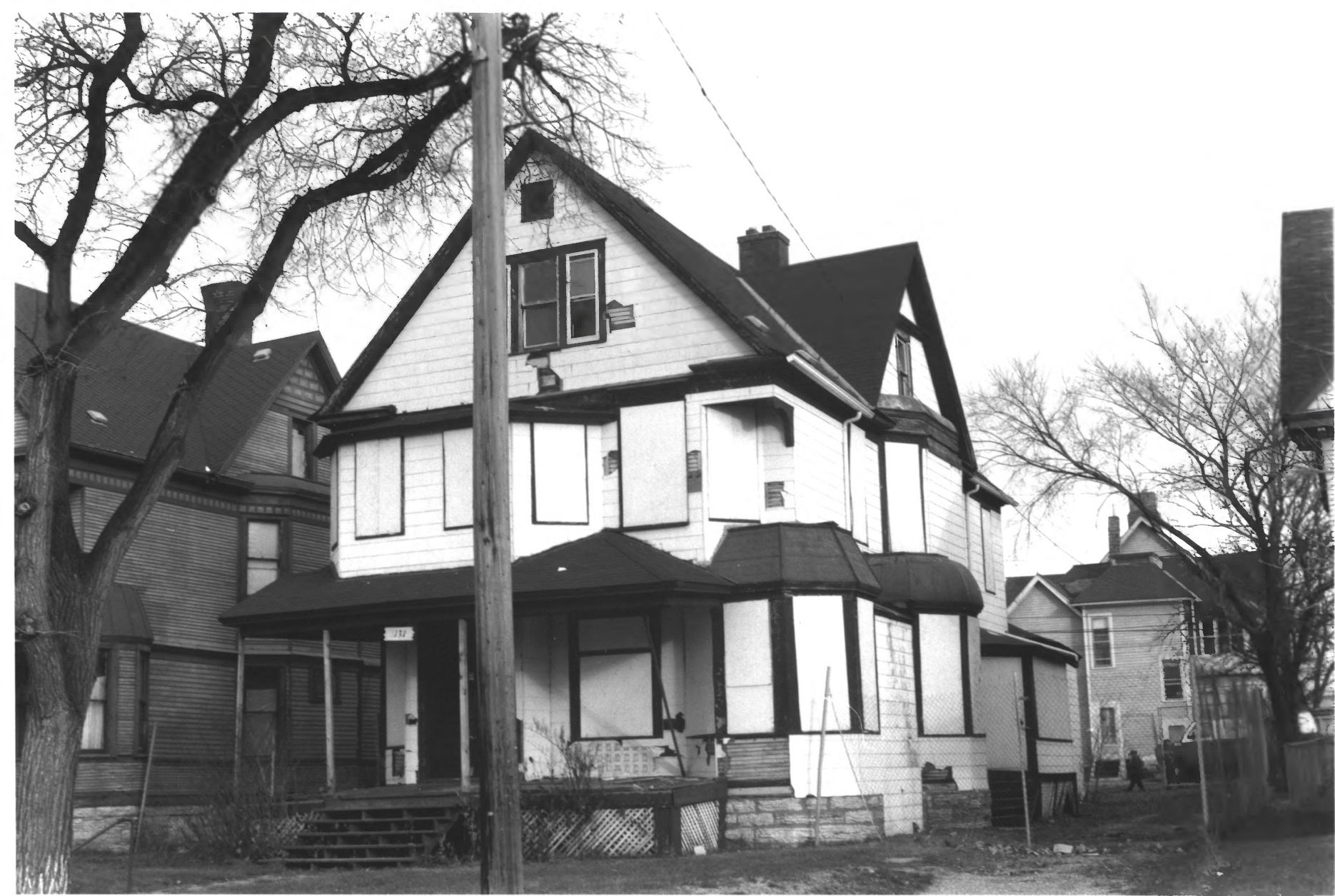
HEALY-REA HOUSE - 3131 2ND AVE. S. HEALY BLOCK HISTORIC DISTRICT MINNEAPOLIS, HENNEPIN COUNTY, MINNESOTA #011476-19
