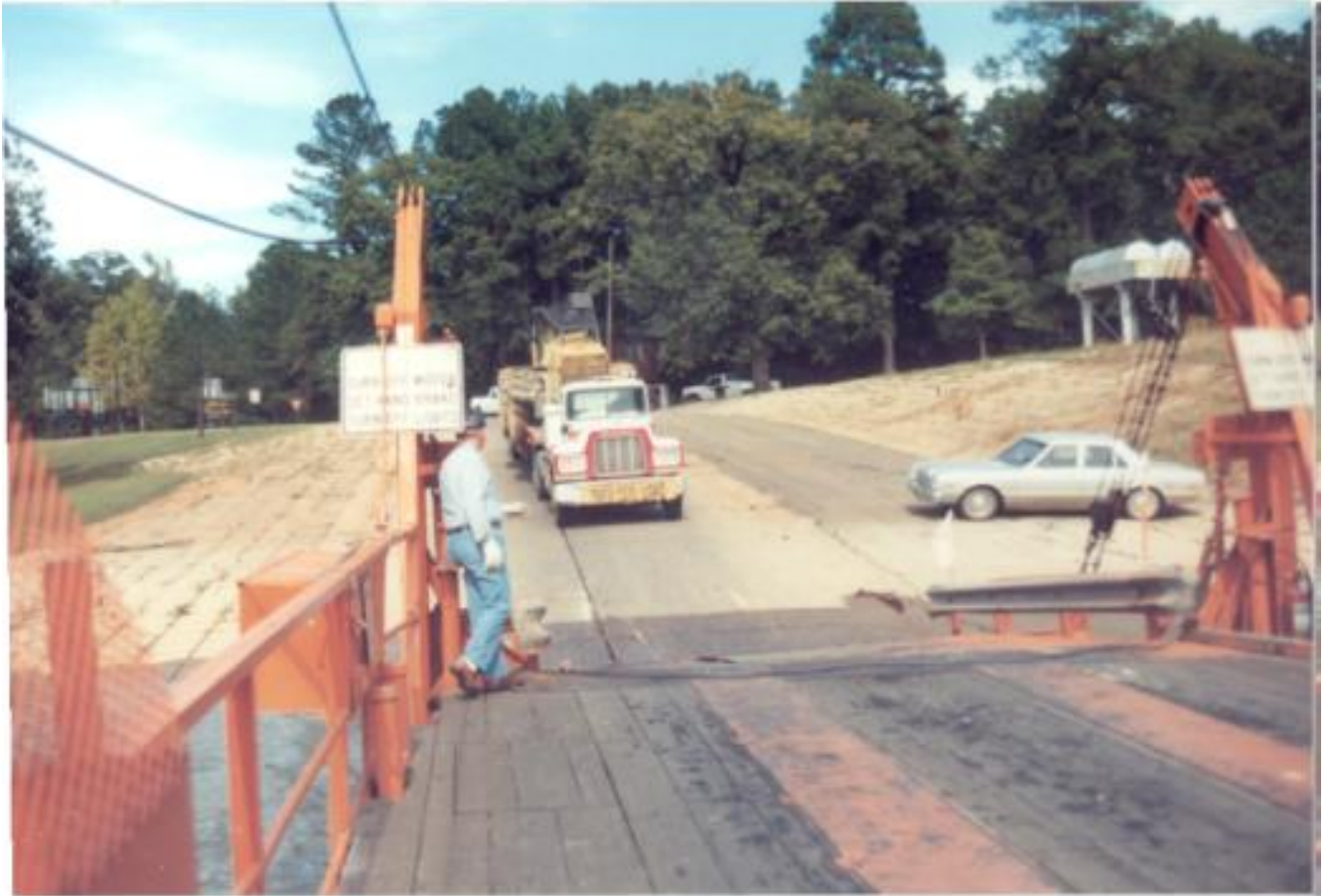
Figure 5: Photograph of a portion of the barge of the Moro Bay Ferry, c.1978. (From the files of Moro Bay State Park.)
