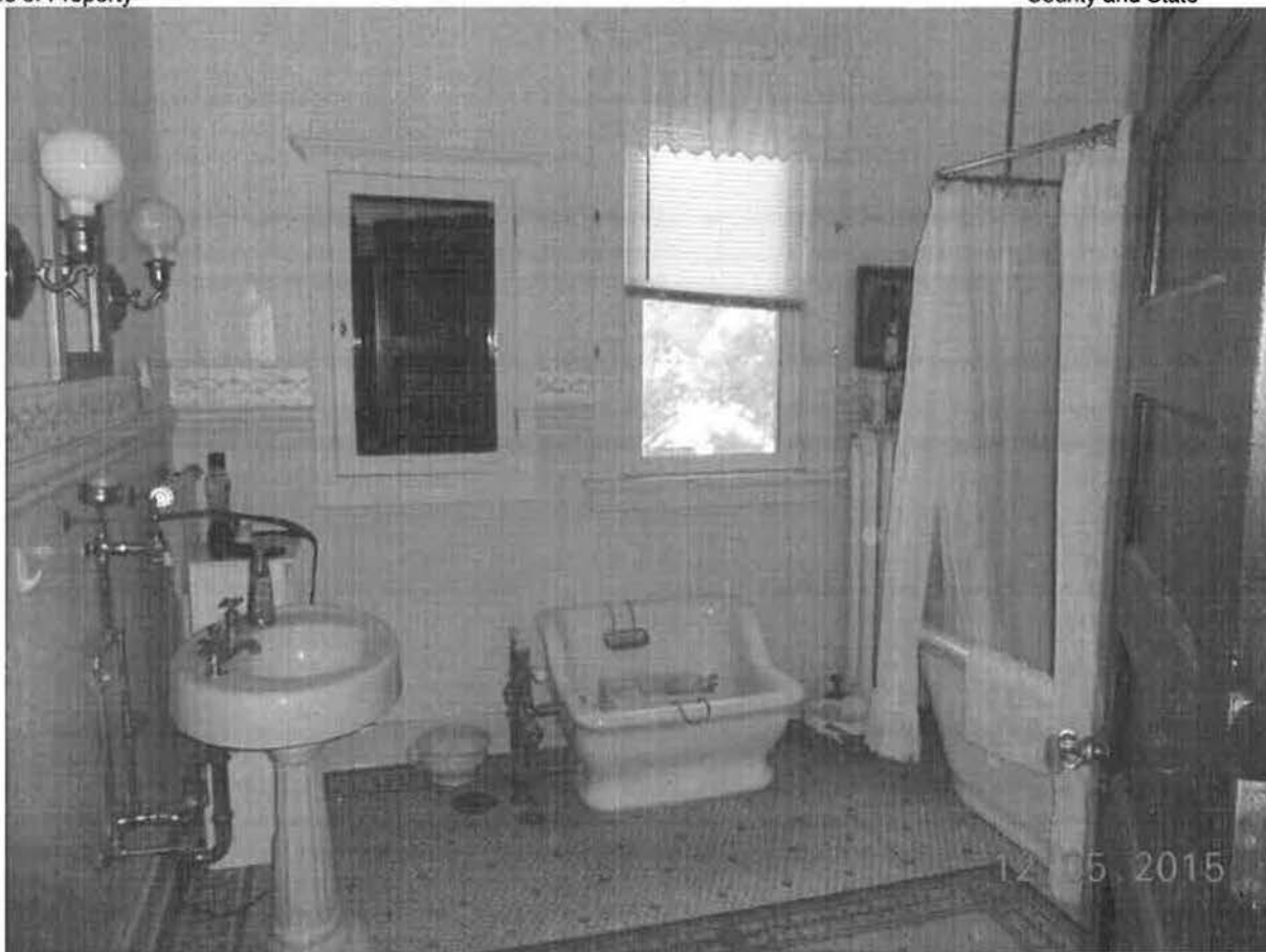
(Image 15) Second floor bathroom, showing original floor tile, sink, and sitz bath. Looking east. (Photo Roberta Wells) (2015)
