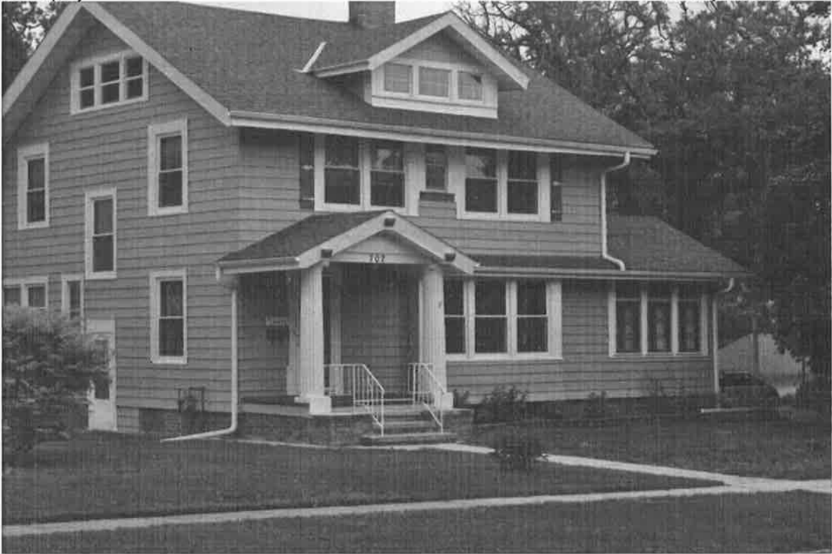
(Image 16) This 1913 house less than a block away from the Perkins residence bears little similarity to the Barber design. Nevertheless, the builder seems to have copied the column design from the much more elaborate Perkins residence. (photo Bruce Perry) (2015)
