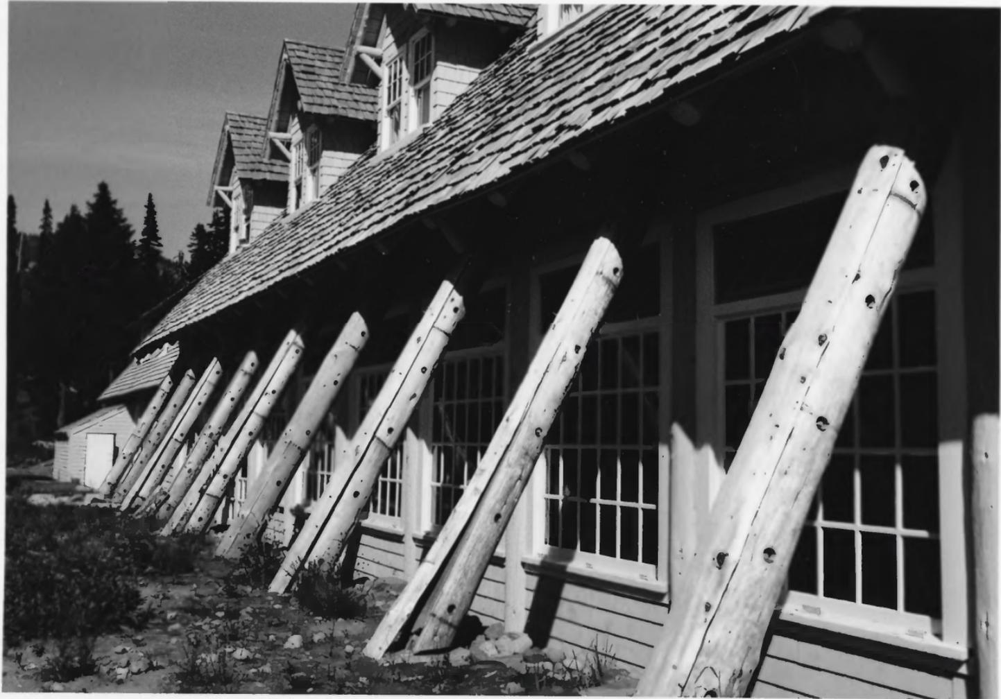
Steel Buttresses Encased in logs, dining
