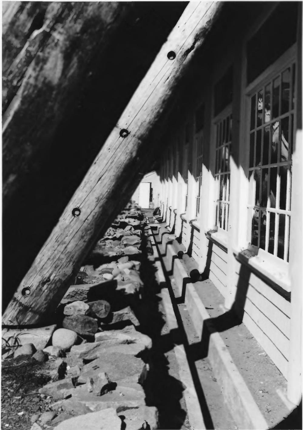
Steel Buttress Encase in Log Sheathing
