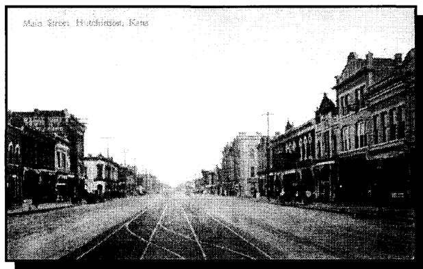
Looking north on Main from Avenue A, prior to storefront rehabilitation.
