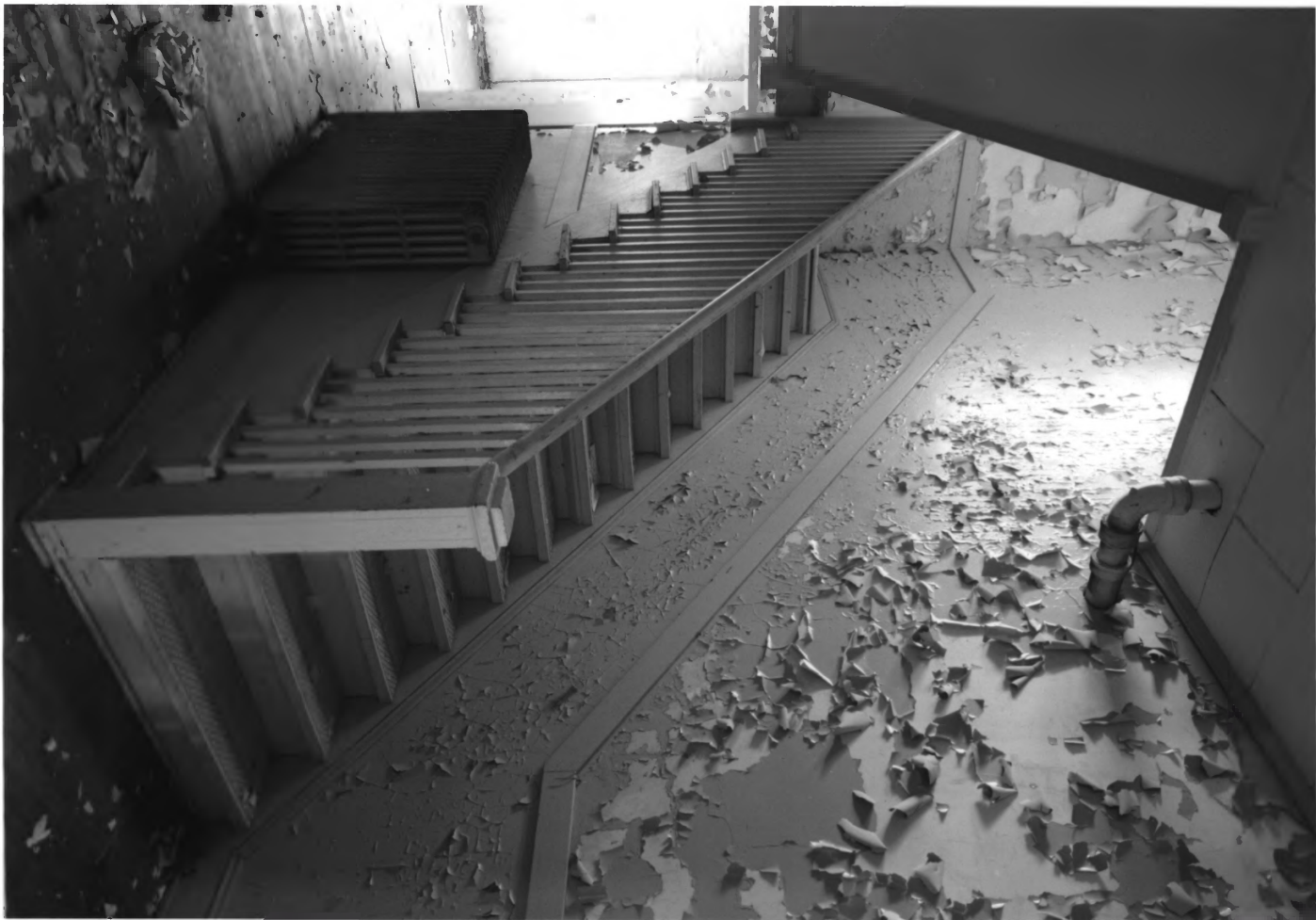
MILLEN HIGH SCHOOL MILLEN, JENKINS COUNTY, GEORGIA PHOTOGRAPH 9 OF 27
