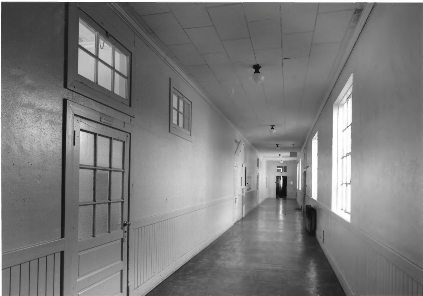
MILLEN HIGH SCHOOL MILLEN, JENKINS COUNTY, GEORGIA PHOTOGRAPH 22 OF 27
