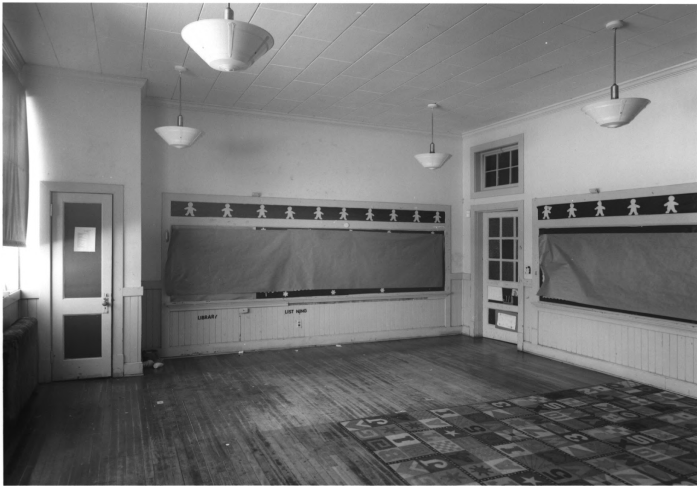
MILLEN HIGH SCHOOL MILLEN, JENKINS COUNTY, GEORGIA PHOTOGRAPH 20 OF 27
