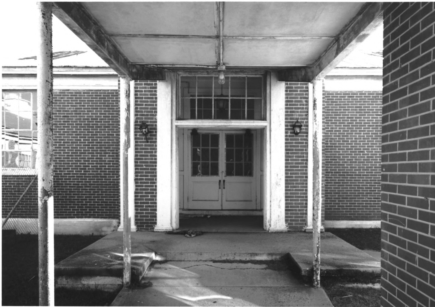
MILLEN HIGH SCHOOL MILLEN, JENKINS COUNTY, GEORGIA PHOTOGRAPH 26 OF 27
