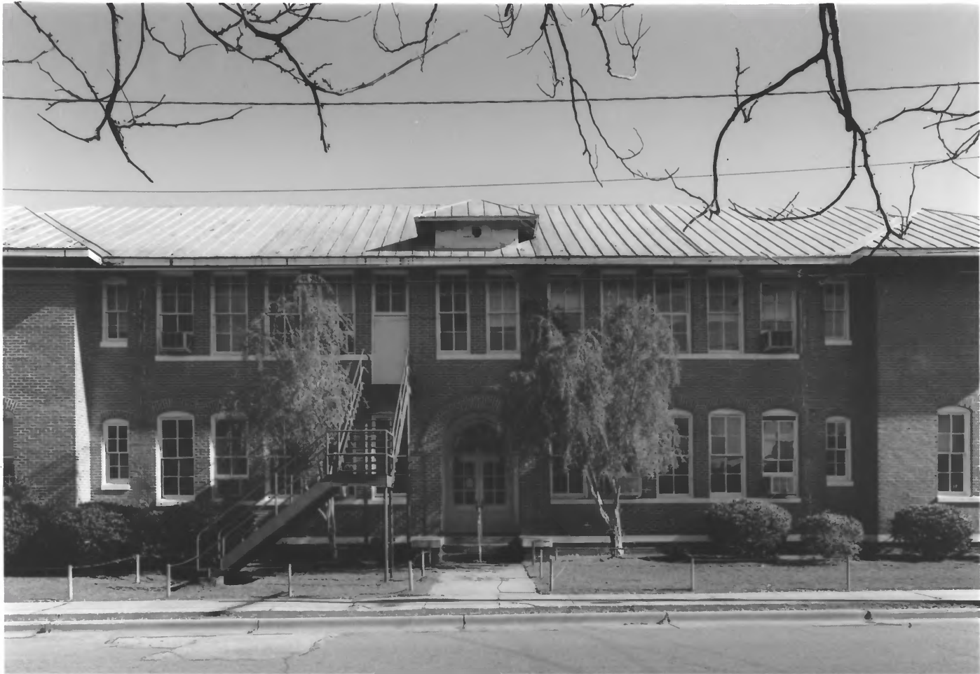
MILLEN HIGH SCHOOL MILLEN, JENKINS COUNTY, GEORGIA PHOTOGRAPH 3 OF 27
