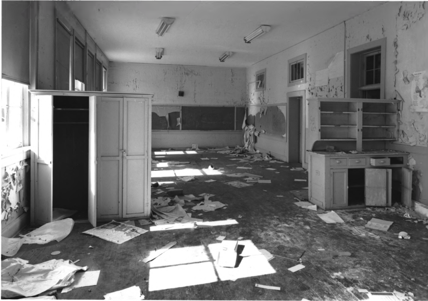
MILLEN HIGH SCHOOL MILLEN, JENKINS COUNTY, GEORGIA PHOTOGRAPH 10 of 27
