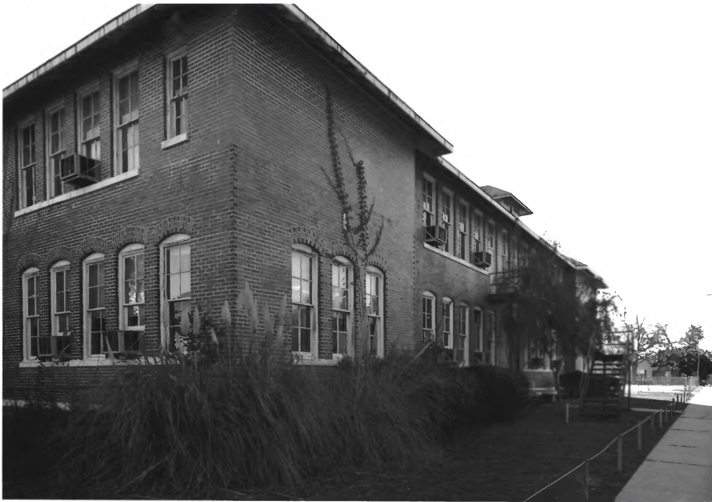
MILLEN HIGH SCHOOL MILLEN, JENKINS COUNTY, GEORGIA PHOTOGRAPH 2 OF 27
