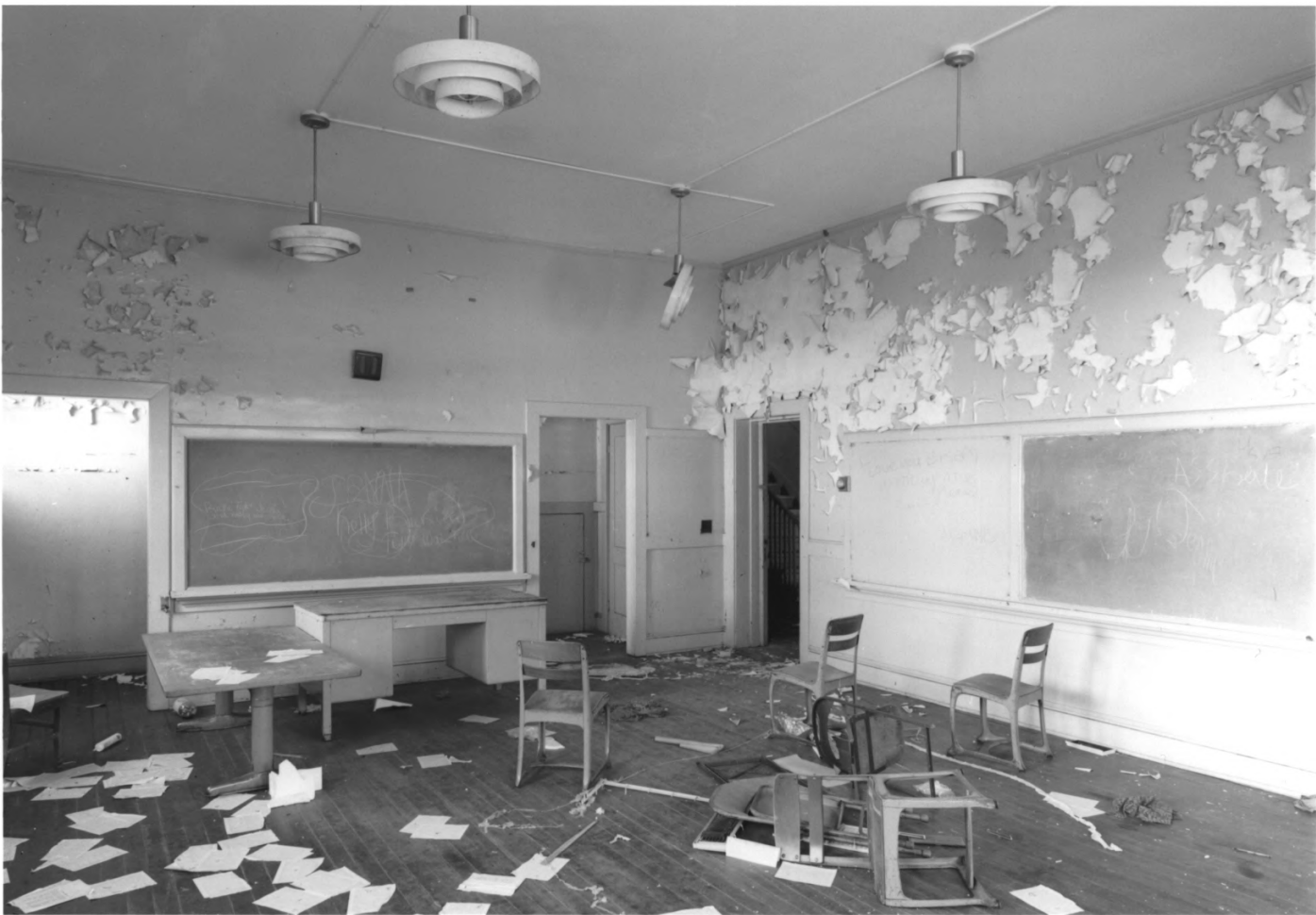
MILLEN HIGH SCHOOL MILLEN, JENKINS COUNTY, GEORGIA PHOTOGRAPH 8 OF 27
