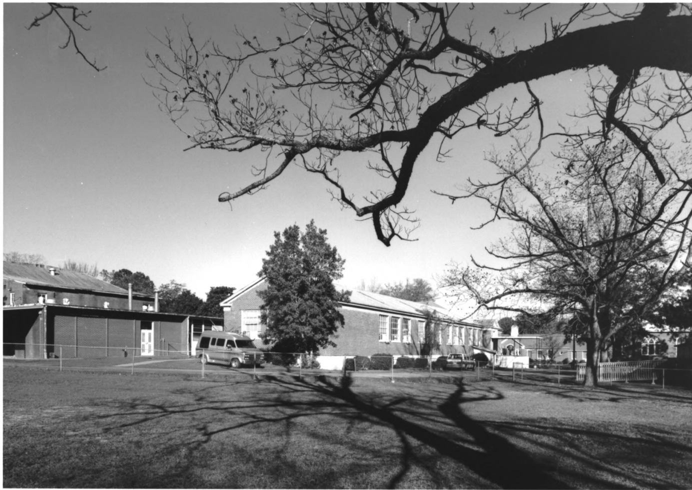
MILLEN HIGH SCHOOL MILLEN, JENKINS COUNTY, GEORGIA PHOTOGRAPH 24 OF 27
