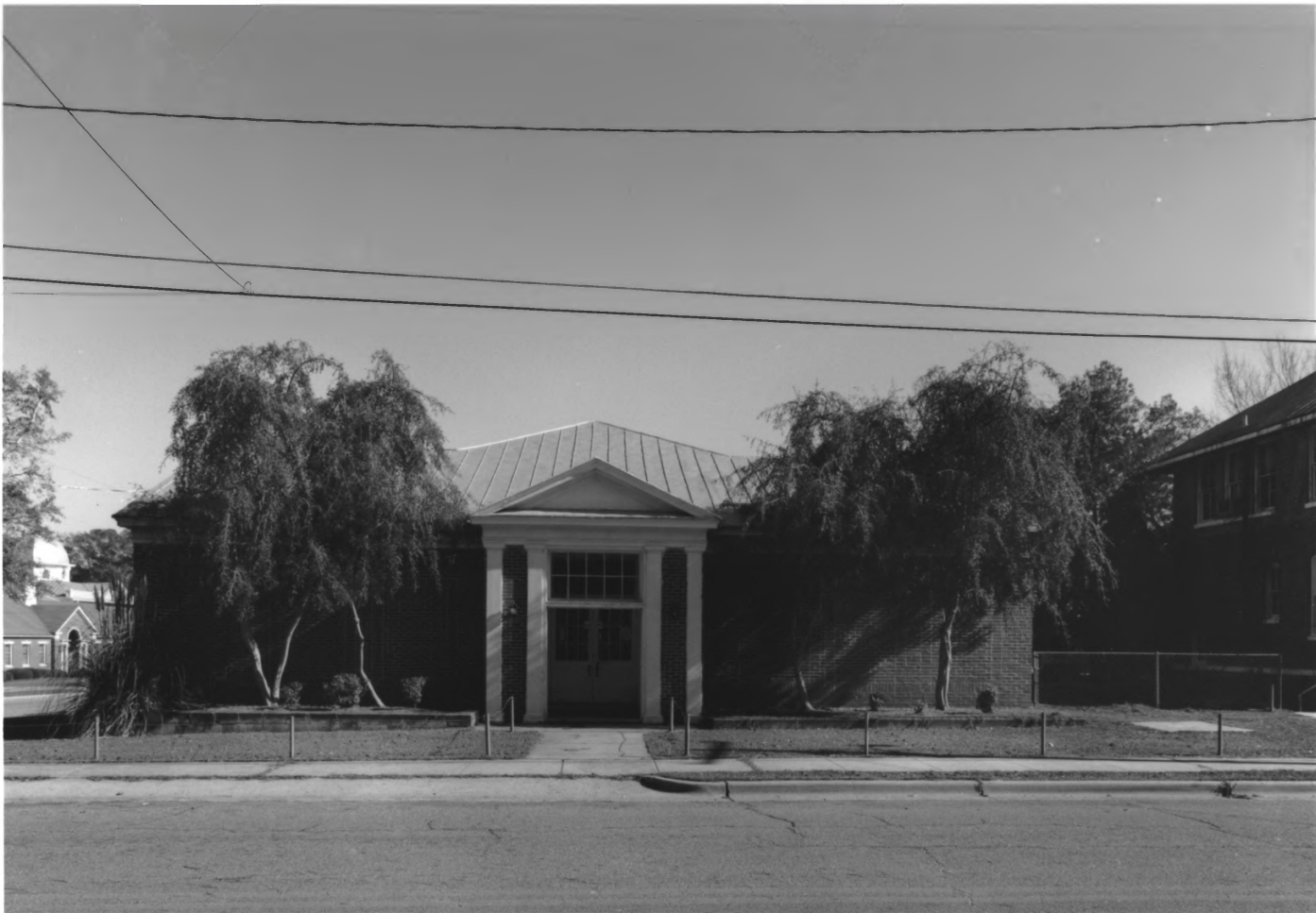
MILLEN HIGH SCHOOL MILLEN, JENKINS COUNTY, GEORGIA PHOTOGRAPH 17 OF 27
