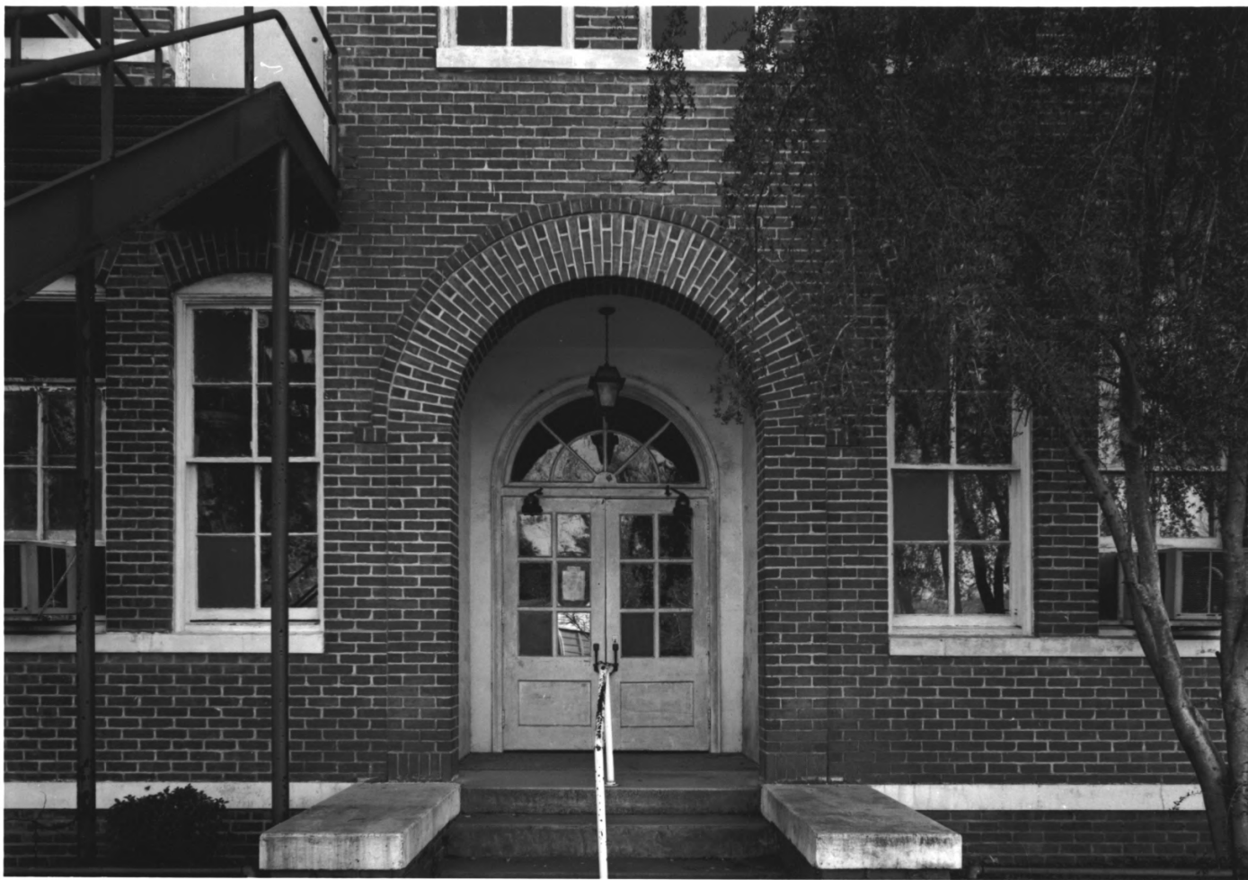
MILLEN HIGH SCHOOL MILLEN, JENKINS COUNTY, GEORGIA PHOTOGRAPH 4 OF 27
