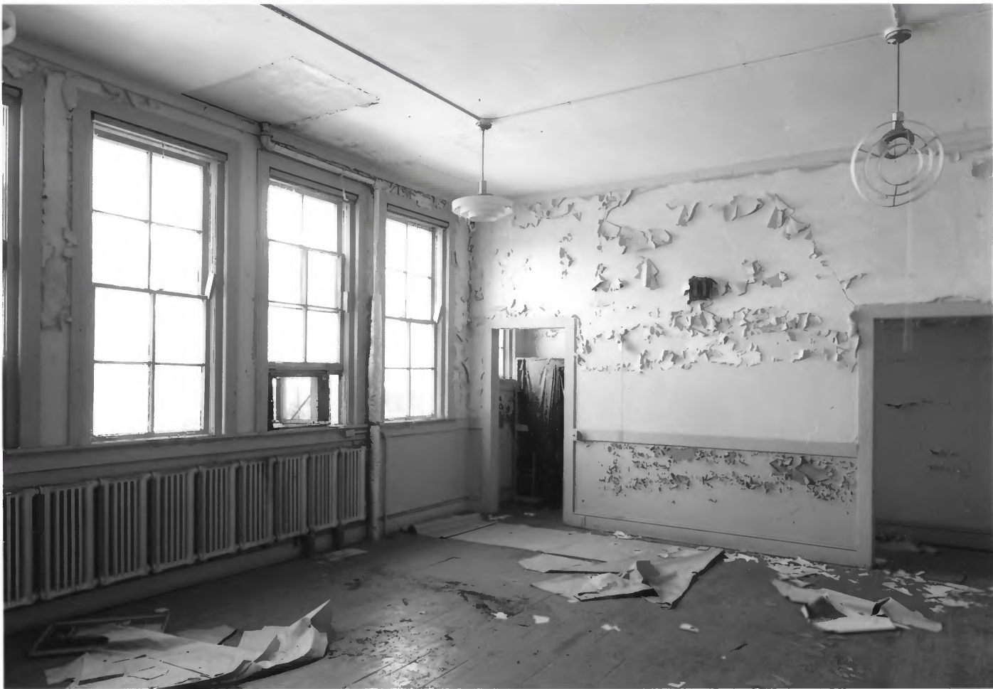
MILLEN HIGH SCHOOL MILLEN, JENKINS COUNTY, GEORGIA PHOTOGRAPH 7 OF 27
