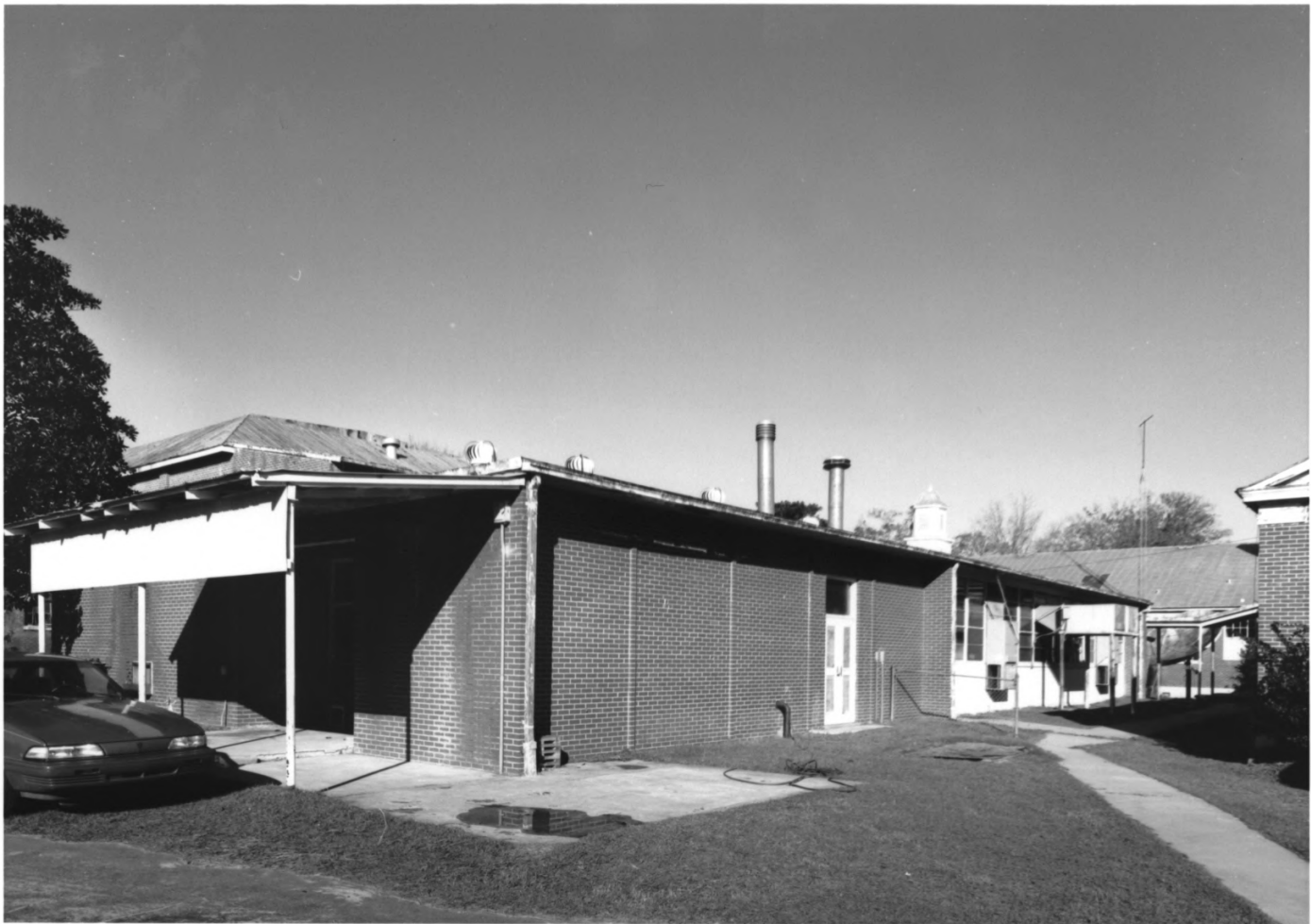
MILLEN HIGH SCHOOL MILLEN, JENKINS COUNTY, GEORGIA PHOTOGRAPH 25 OF 27
