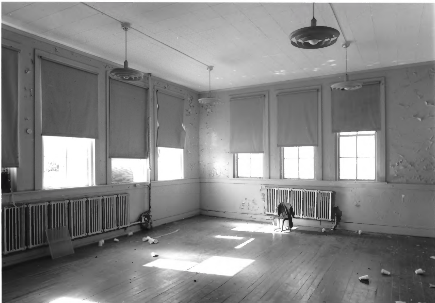
MILLEN HIGH SCHOOL MILLEN, JENKINS COUNTY, GEORGIA PHOTOGRAPH 6 OF 27
