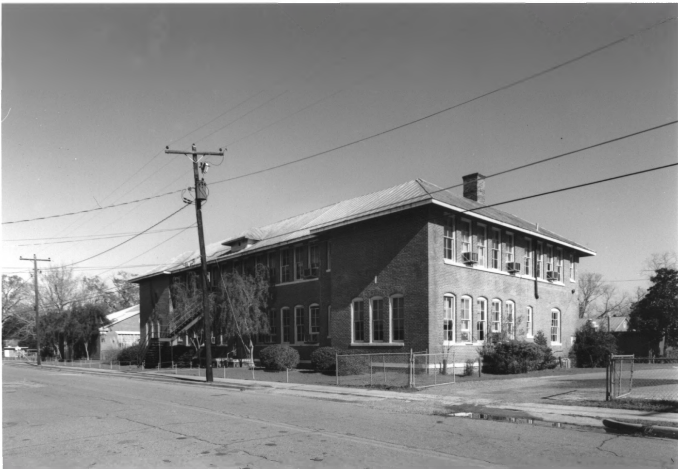
MILLEN HIGH SCHOOL MILLEN, JENKINS COUNTY, GEORGIA PHOTOGRAPH 1 OF 27
