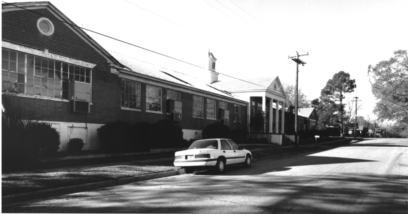
MILLEN HIGH SCHOOL MILLEN, JENKINS COUNTY, GEORGIA PHOTOGRAPH 16 OF 27
