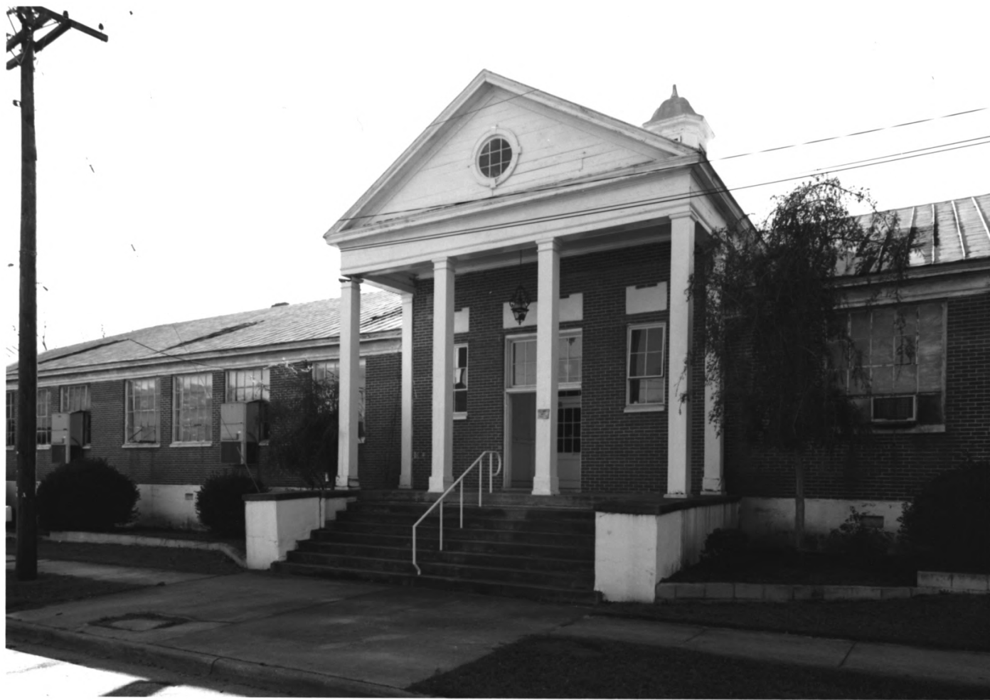
MILLEN HIGH SCHOOL MILLEN, JENKINS COUNTY, GEORGIA PHOTOGRAPH 18 OF 27
