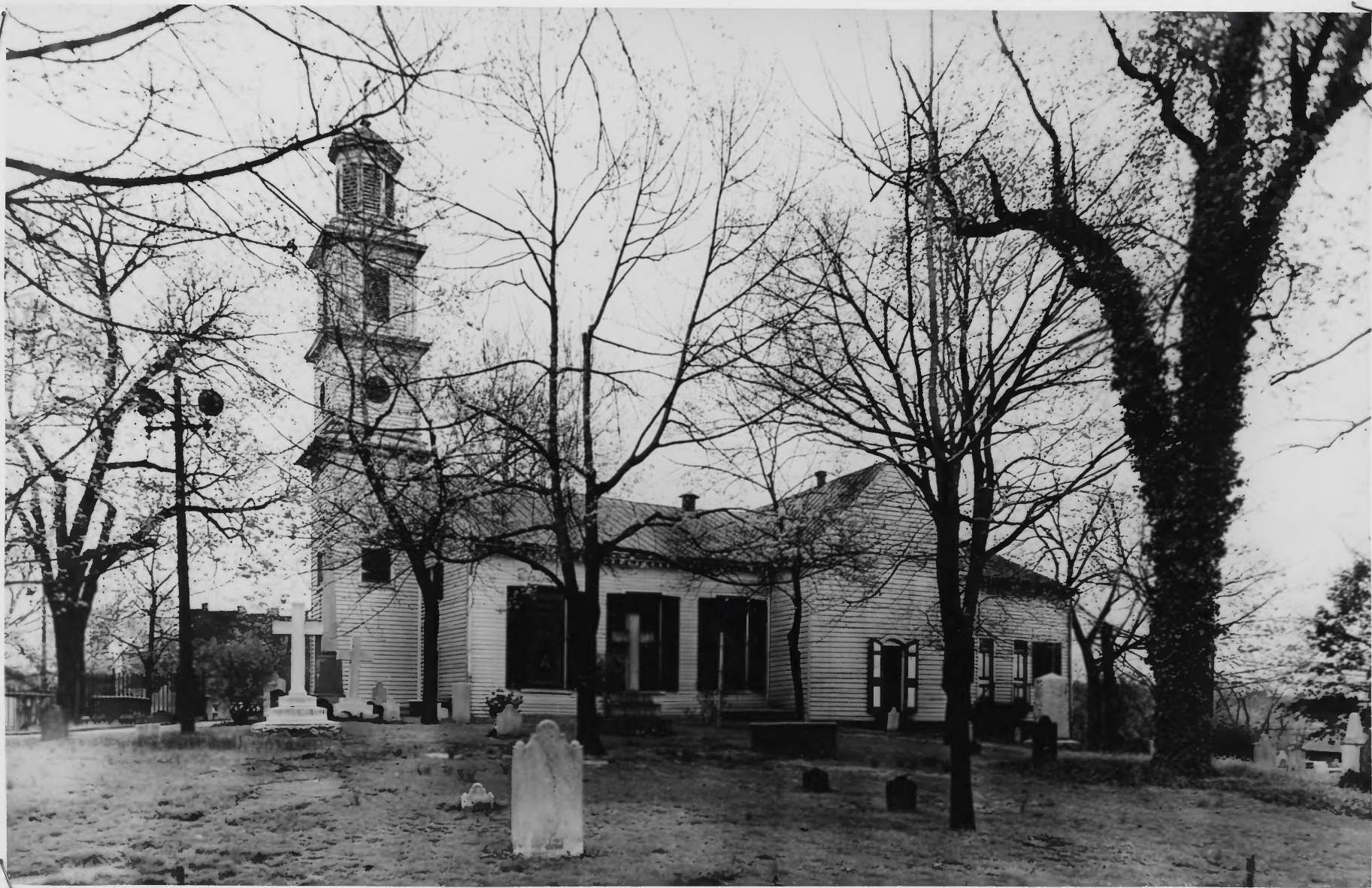
View looking east to west face of St. John's Church, Richmond, Virginia. The door framing of the door which shows at the west transept dates from 1772. Most of the siding on the transepts is original (1741). The nave, to a point at the end of the first window from the front of the church, was built in 1772. The remainder of the nave was built in 1830. The tower was erected between 1830-1835, and the present tower dates from 1896. The chancel and vestry room at the south end (right end of structure in picture) were built in 1880. George Wythe's grave is marked by the large rectangular stone directly in front of the west transept door.
