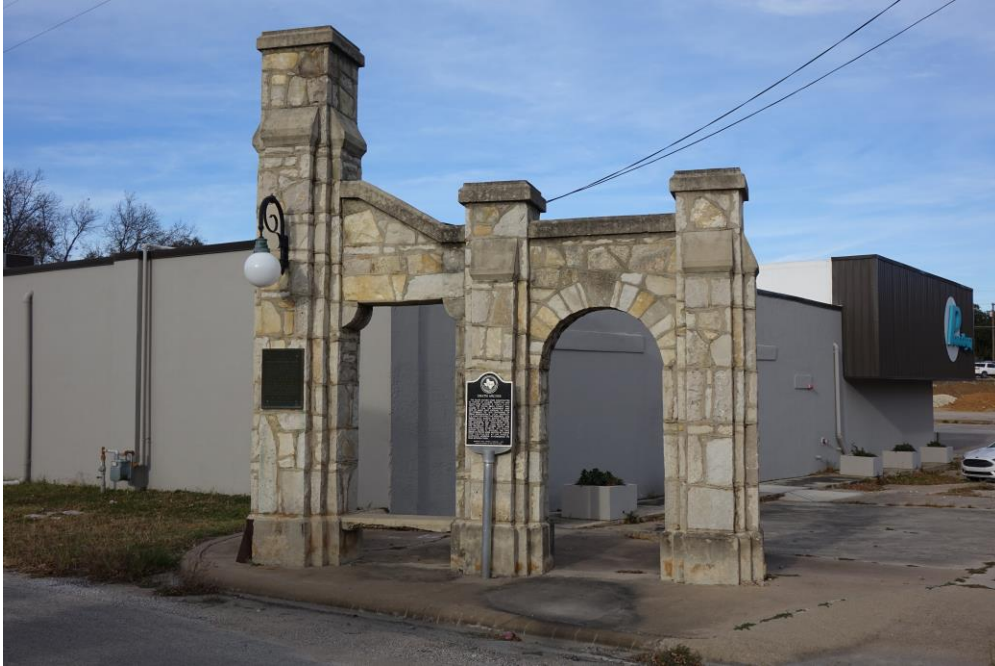
Photo 3 - East Gate, facing northeast
