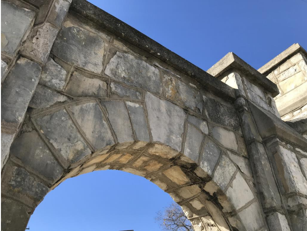
Photo 7 - East gate, detail of arch, facing northwest
