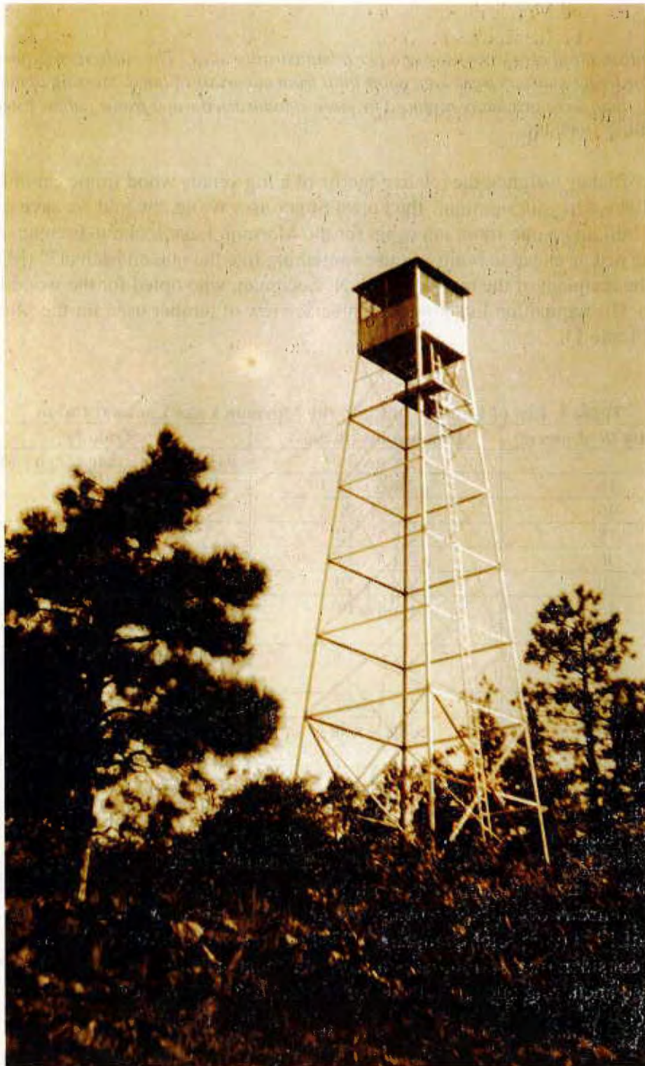
Figure 3. The 1927 Aermotor Tower
