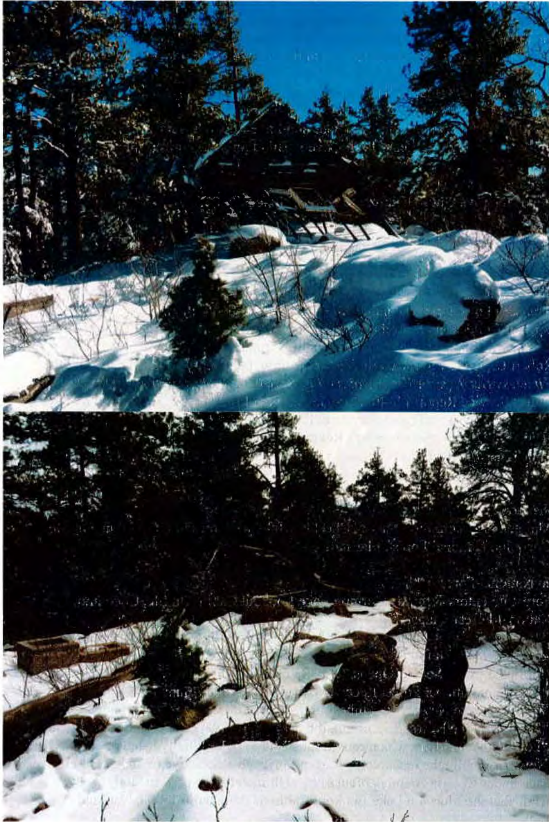
Figure 10. The Mormon Lake Lookout Cabin on 12/03/2018 (top), and then on 12/17/2018 (bottom), after it had collapsed. Photos compliments of Sue Priest.
