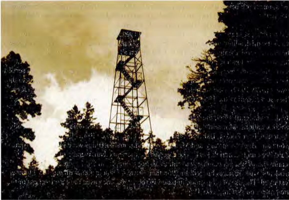
Figure 6. The Aermotor Tower in 1932, Showing New, Interior Stairs
