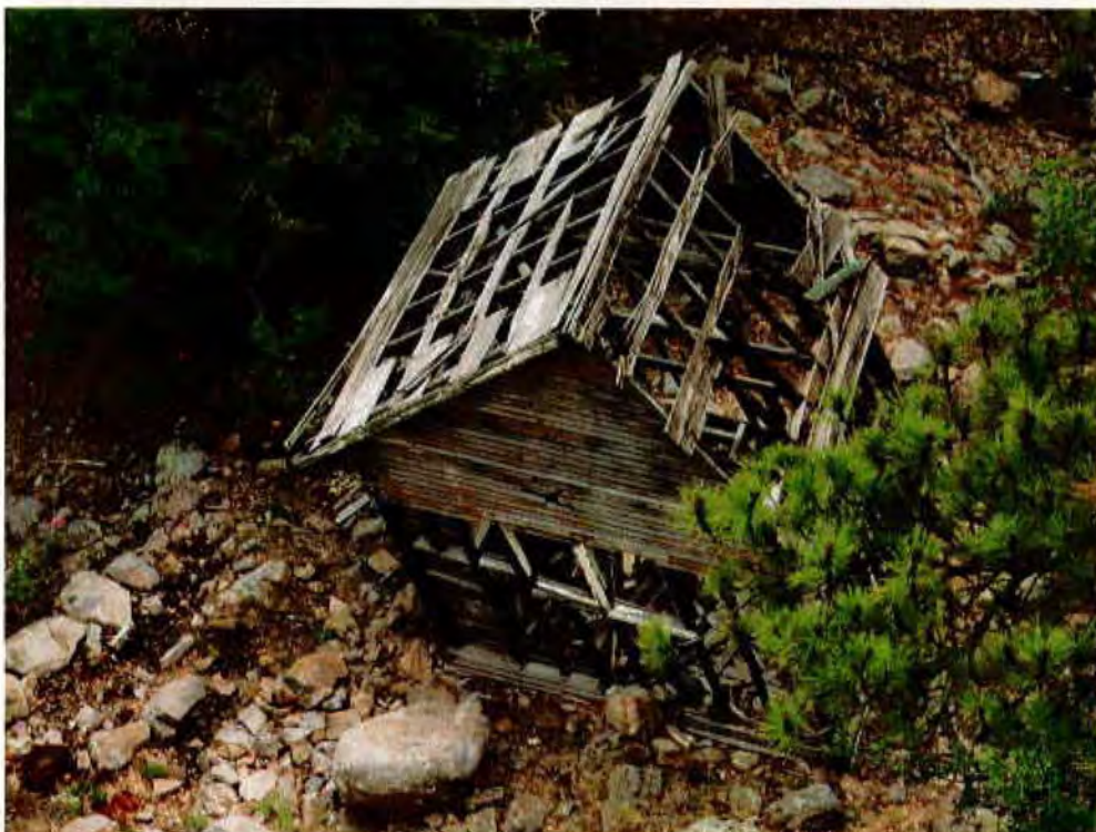
View looking down at roof of cabin
