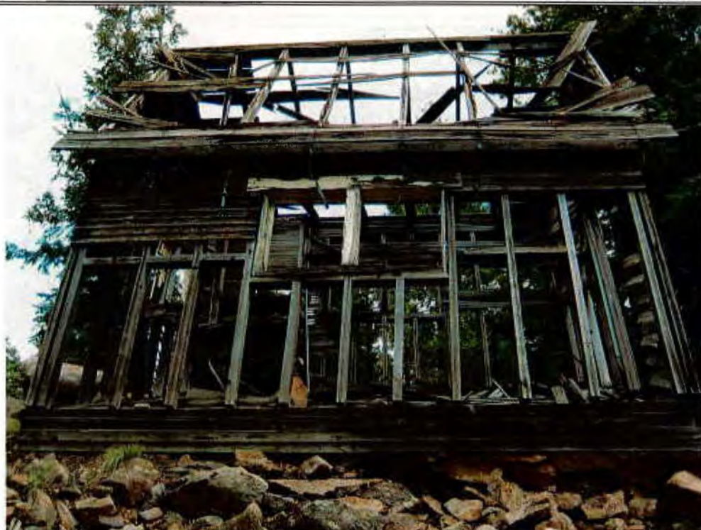
View to north and up, showing south elevation and interior
