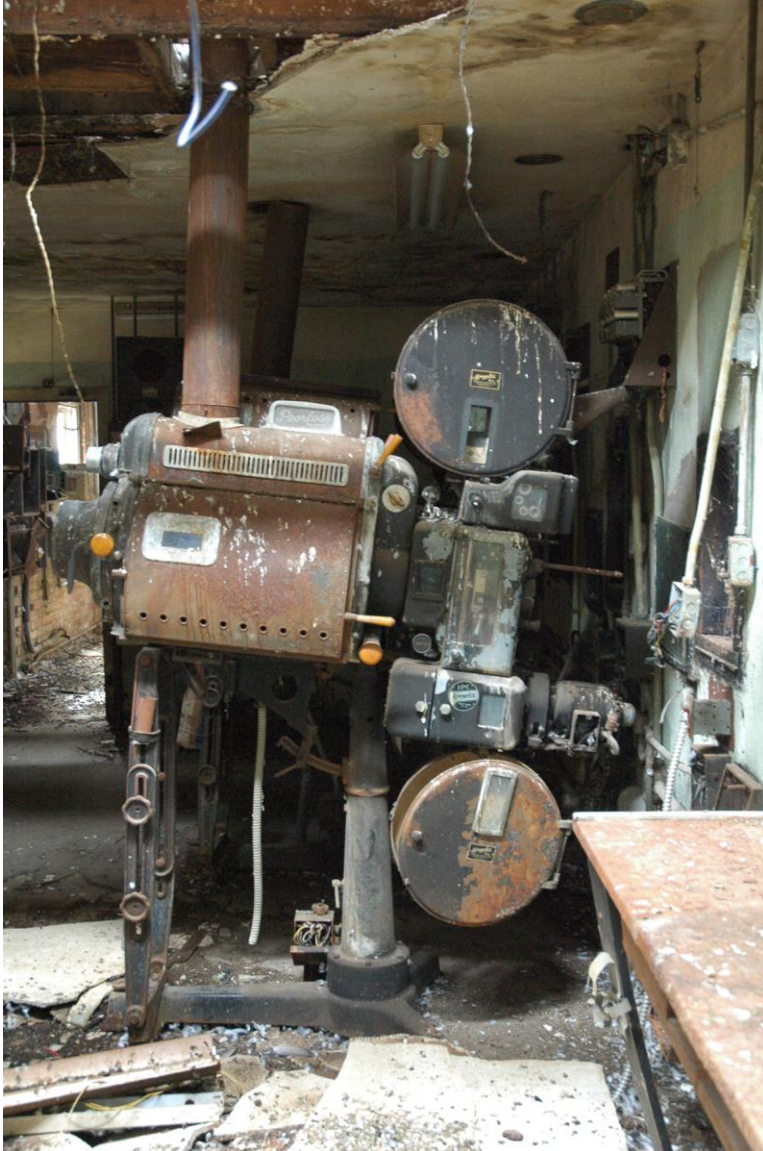
Photo 12 Projection room, Camera facing south
