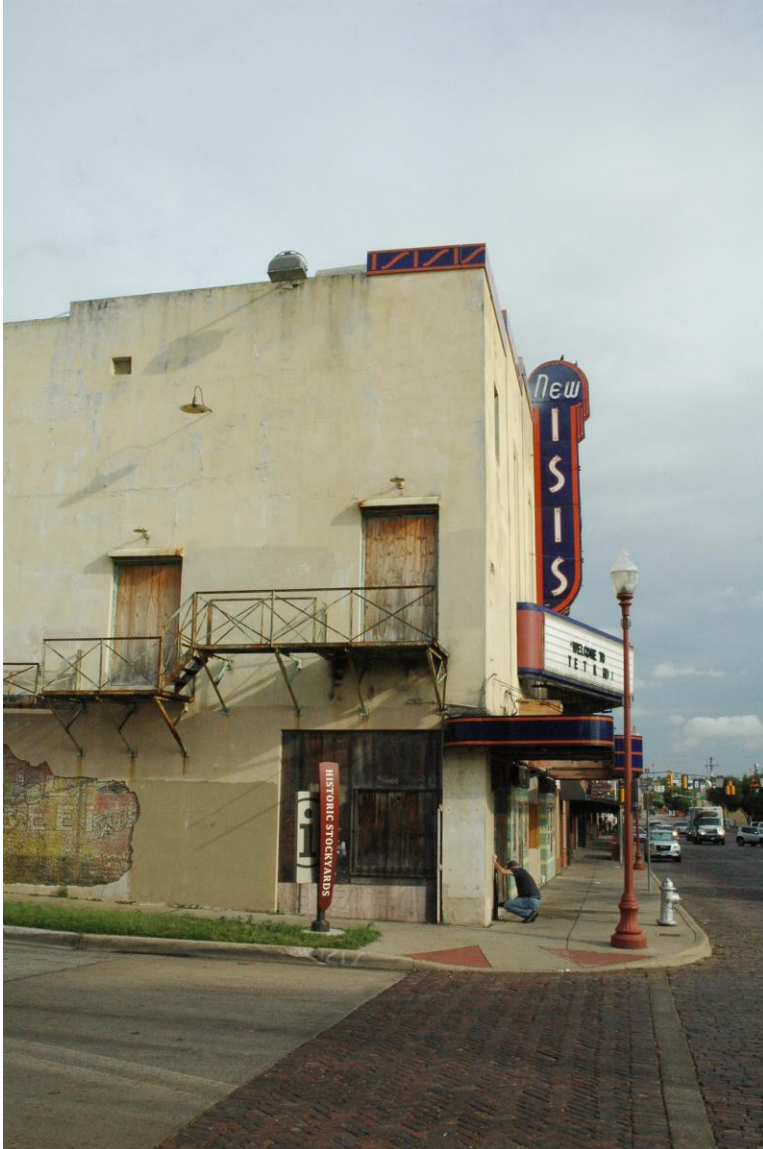
Photo 2 Southeast corner, Camera facing north
