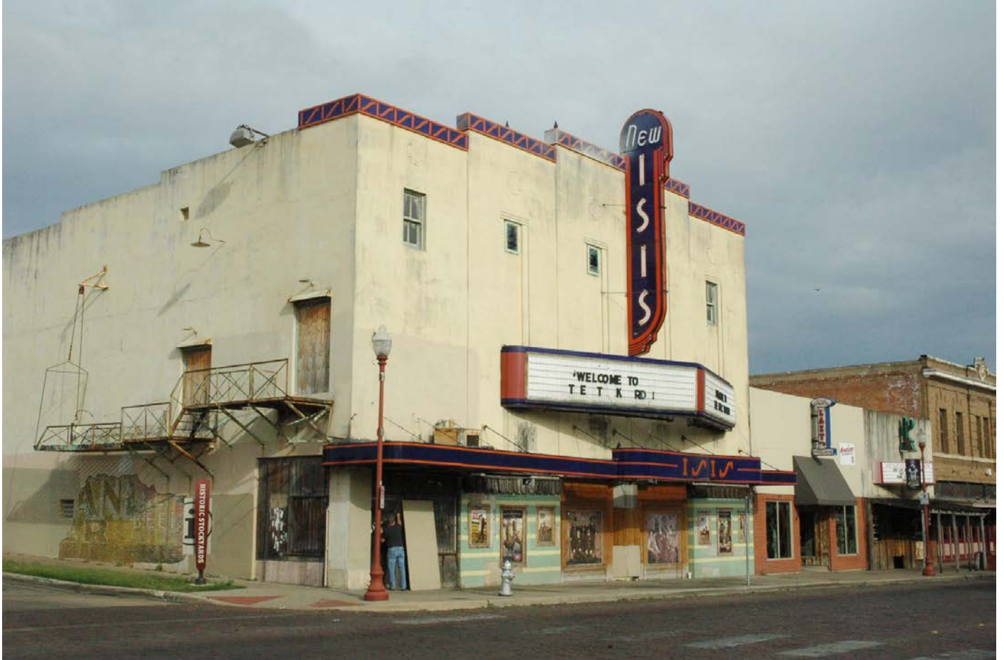
Photo 1 Southeast oblique, Camera facing northwest
