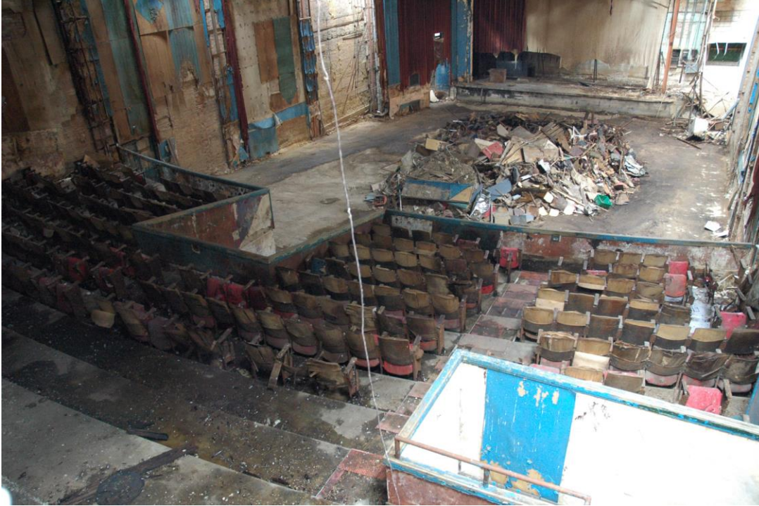
Photo 8 Looking towards stage from mezzanine, Camera facing southwest
