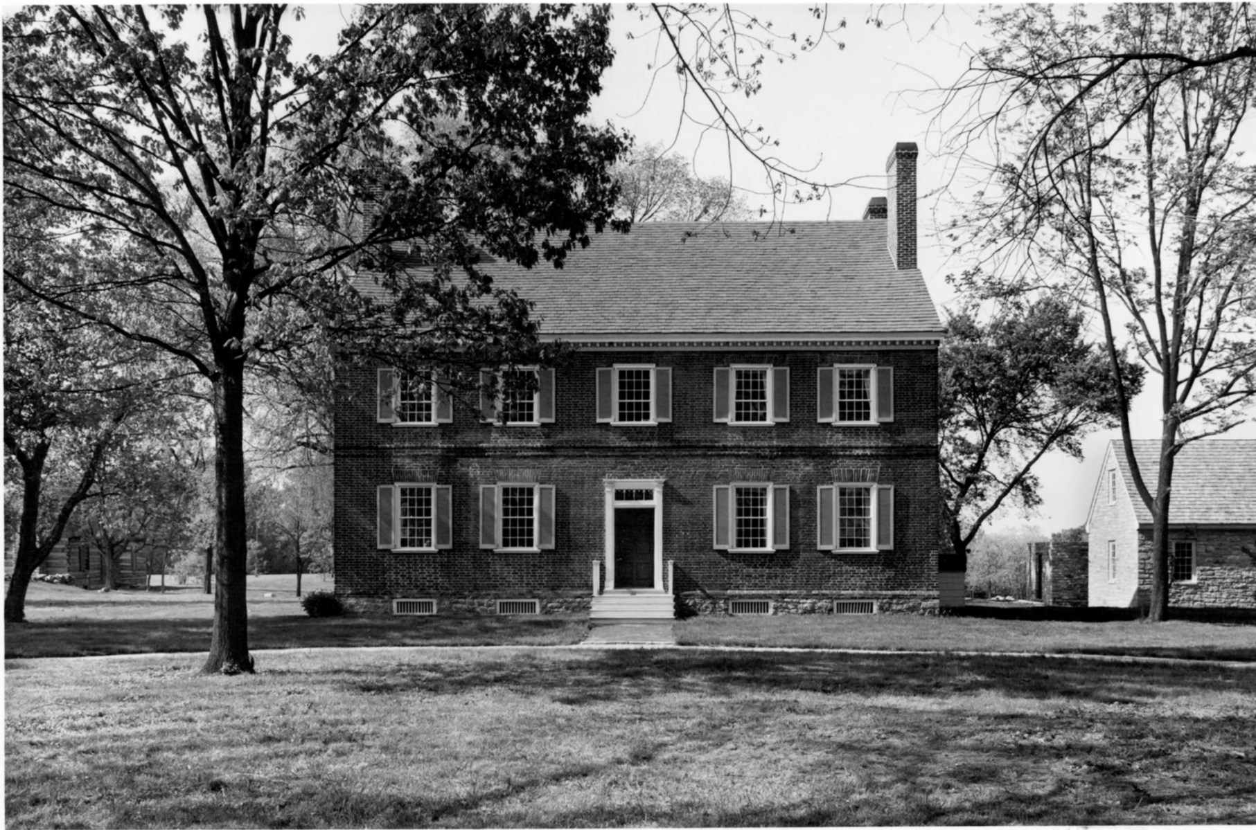
18 Locust Grove, front elevation, c. 1971 Photograph by H. J. Scheirich, III, from National Register files
