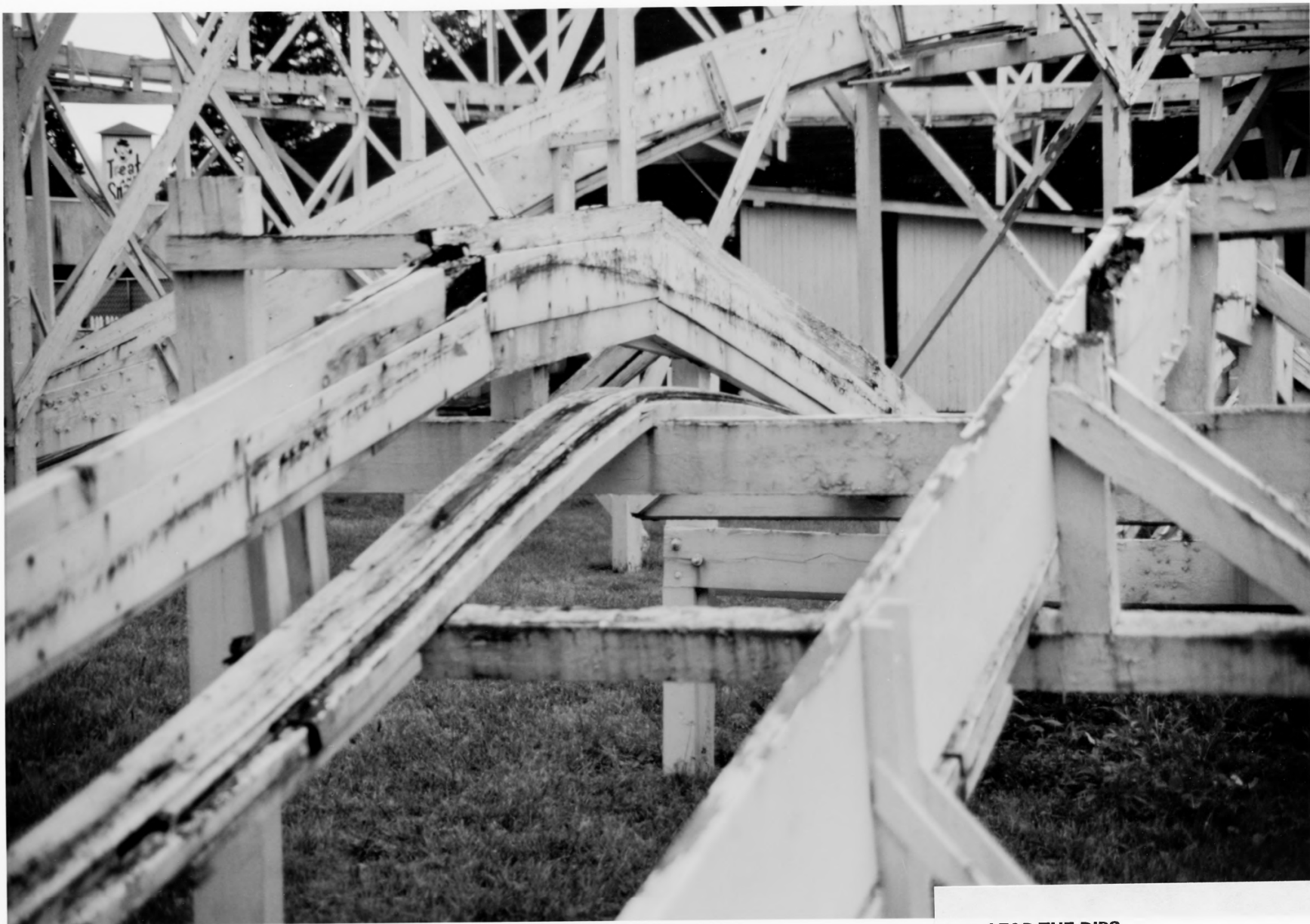
LEAP-THE-DIPS Logan Township, Pennsylvania Close-up view of the side-friction type track Photo #3: Tom Halterman, 1990
