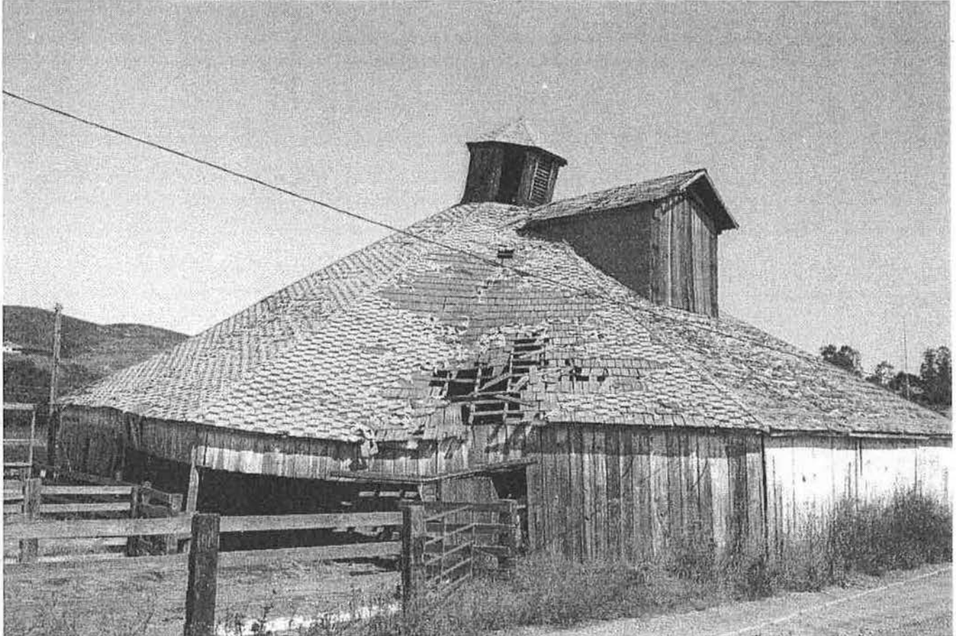
Figure 8: Octagon Barn shows great decay, and was, in fact, in danger of collapse. Photo is from Robert Vessely, engineer. This view also shows a dormer on the Barn. It is unclear whether this was part of the original structure and has not been reproduced on the restored barn.
