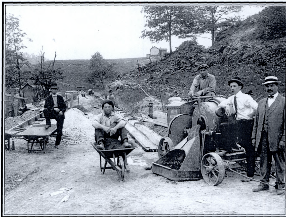
Fig. 6 A dapper Thoney Pietro appears at the far right in this photo of a paving project in the Williamson Historic District. [from the Thoney Pietro Collection, West Virginia State Archives]
