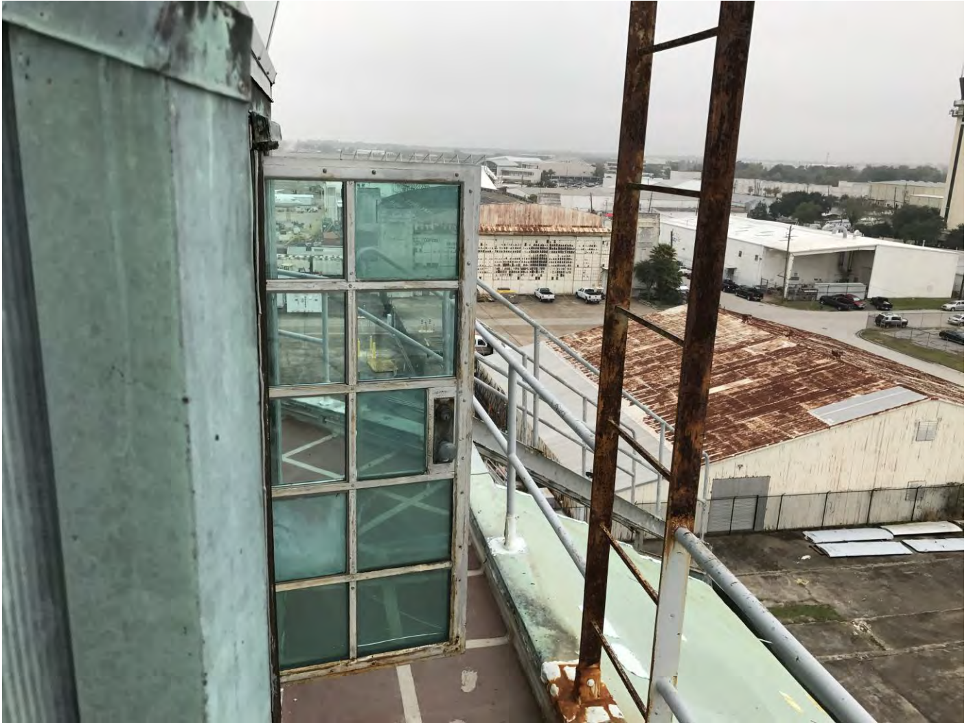
Photo 13 Control Tower exterior, facing south Photo by Gregory Smith, December 2016
