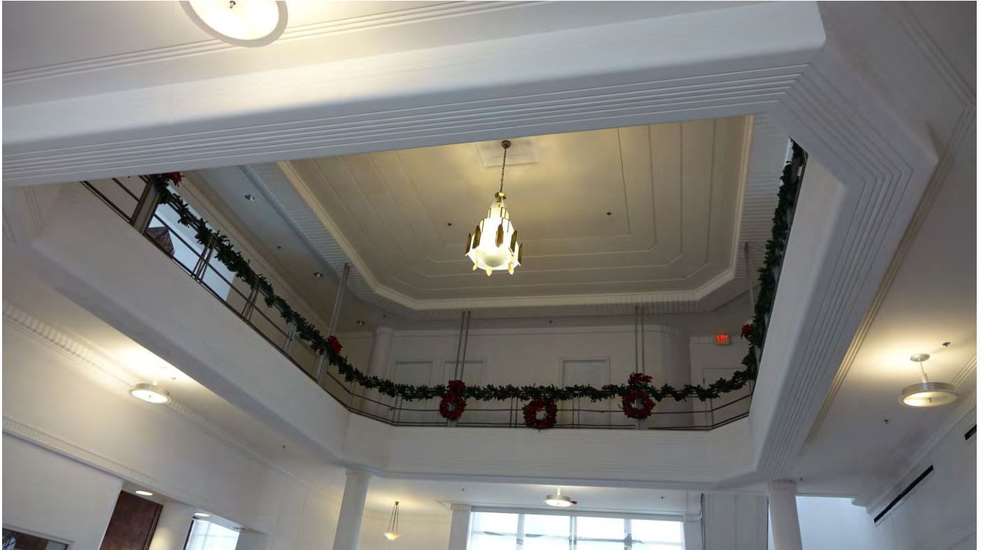
Photo 11 Lobby ceiling, facing east Photo by Gregory Smith, December 2016
