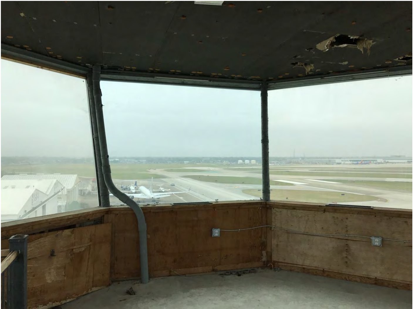
Photo 12 Control Tower interior, facing north-northeast Photo by Gregory Smith, December 2016
