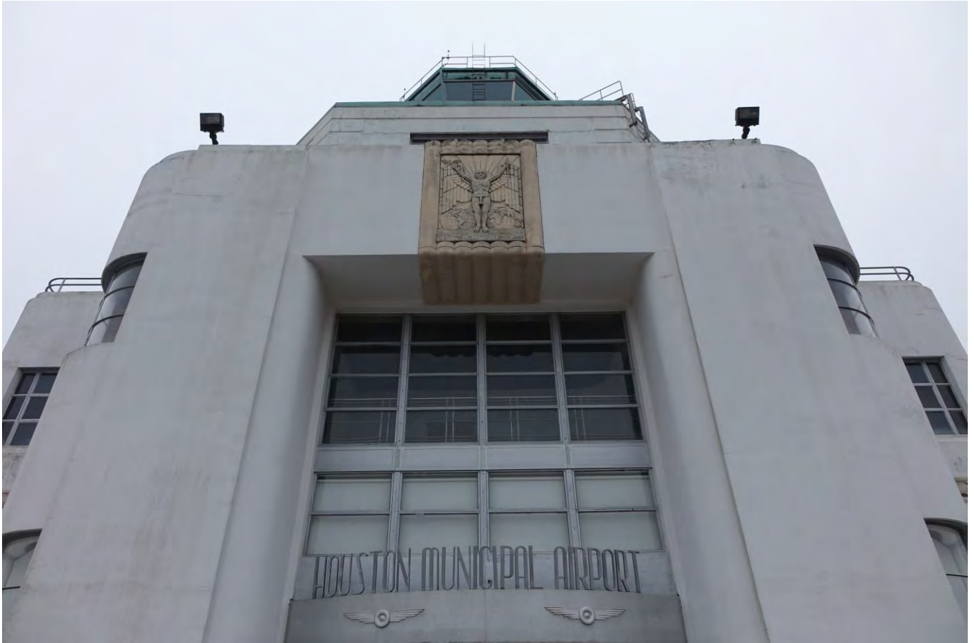
Photo 8 West elevation detail Photo by Gregory Smith, December 2016
