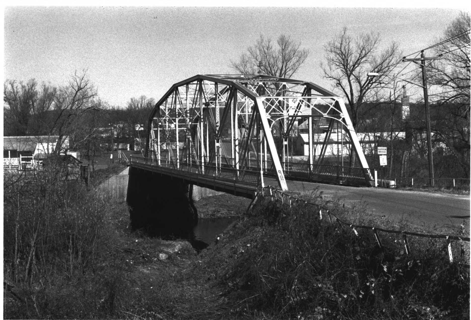
THIRD STREET BRIDGE GOODHUE CO., MN PHOTO I.D. 09140#12
