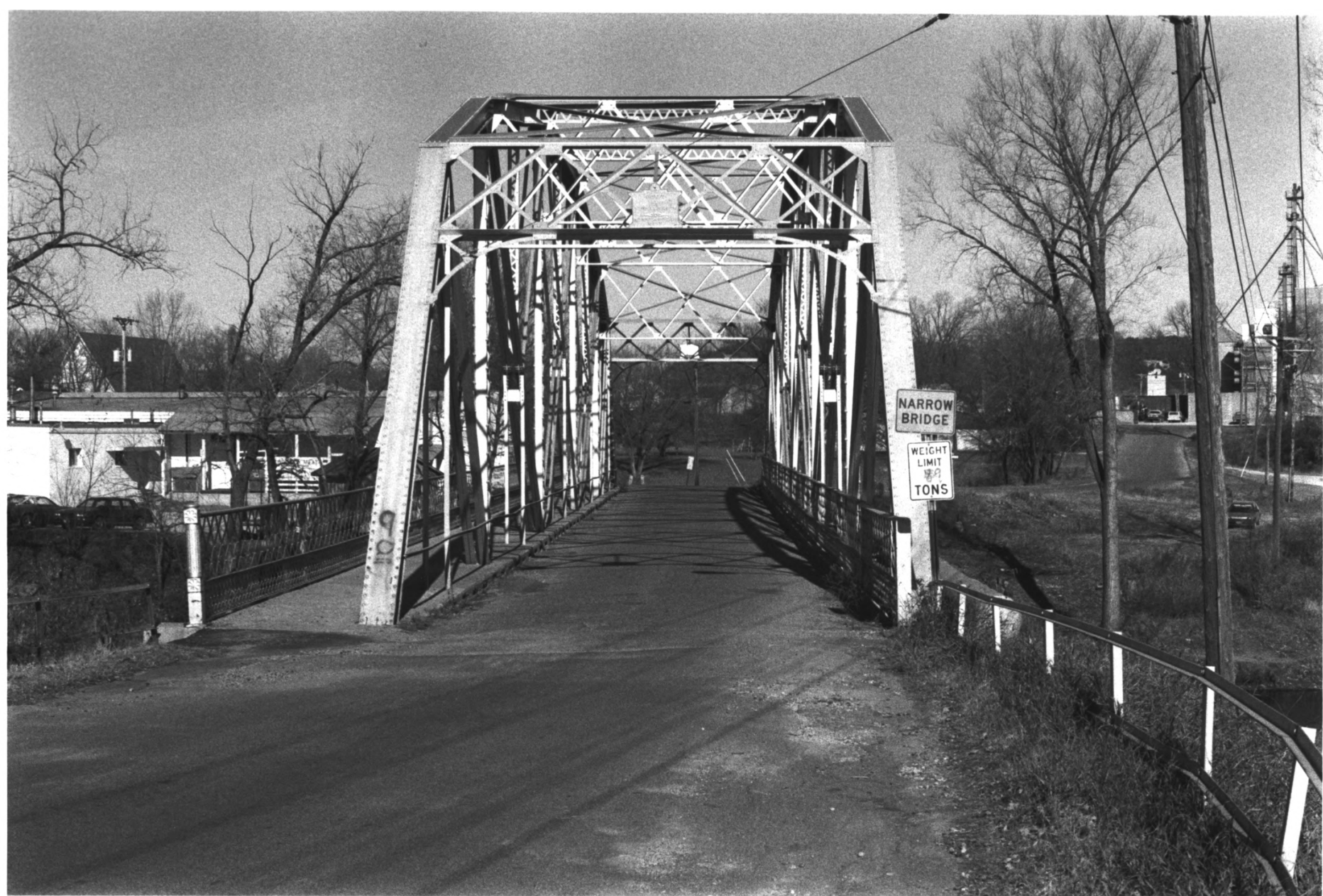
THIRD STREET BRIDGE GOODHUE CO., MN PHOTO I.D. 09140 #11
