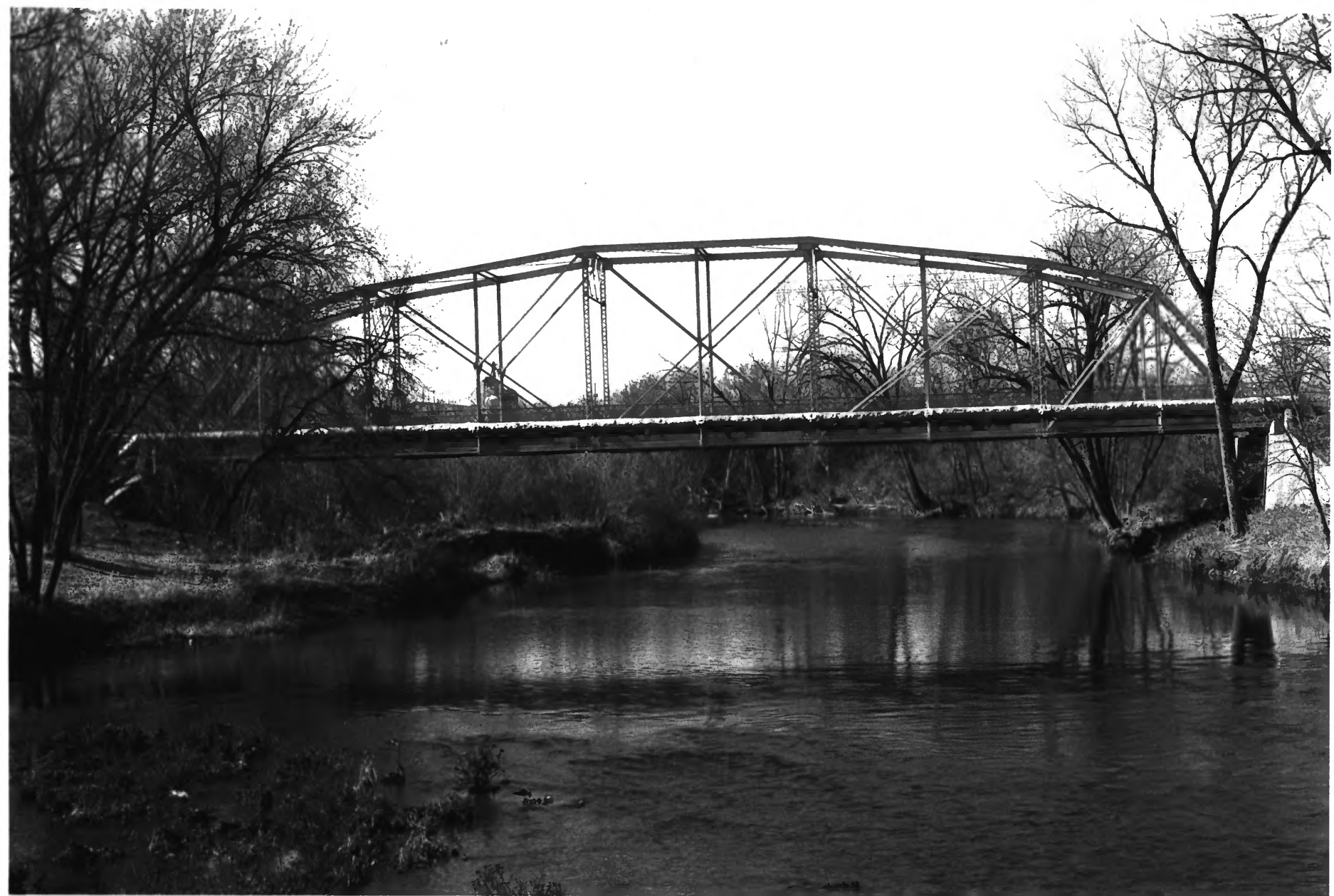
THIRD STREET BRIDGE GOODHUE CO., MN PHOTO I.D. 09140 # 16
