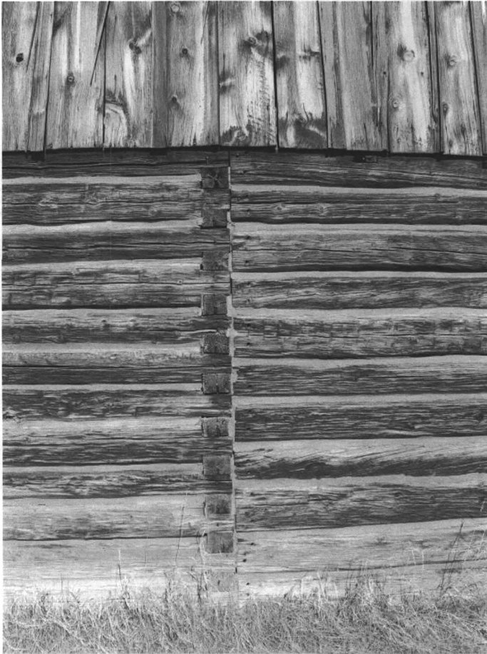
Wold Barn #17. Log joint between main component and log addition, west elevation, view to east.
