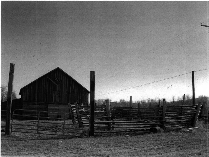
Wold Barn #3. North elevation of barn and round corral, view to the south.
