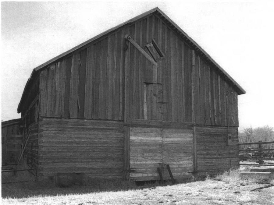
Wold Barn #12. North elevation main component, view to the south.
