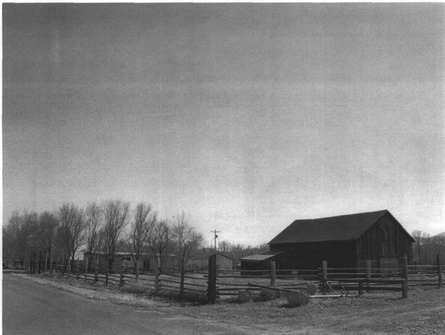
Wold Barn #2. North and east elevations of barn and east fence, view to the southwest.
