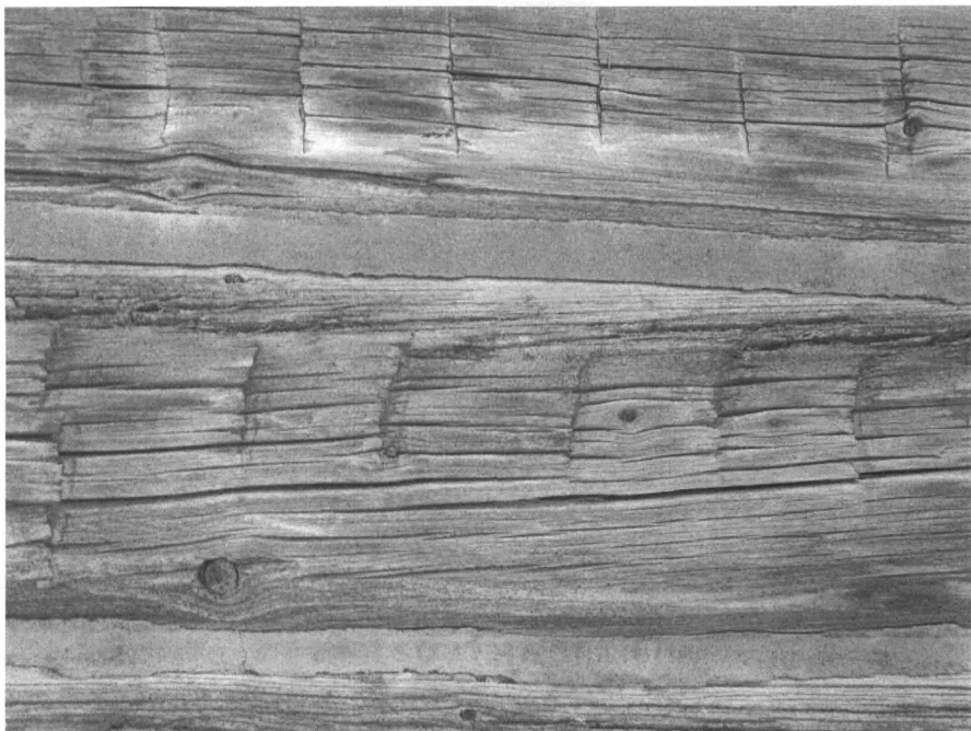
Wold Barn #14. Adze marks detail, north elevation, view to the south.
