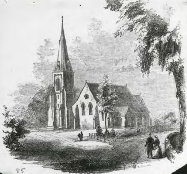
EPISCOPAL CHURCH, BROOKLINE, MASSACHUSETTS.
