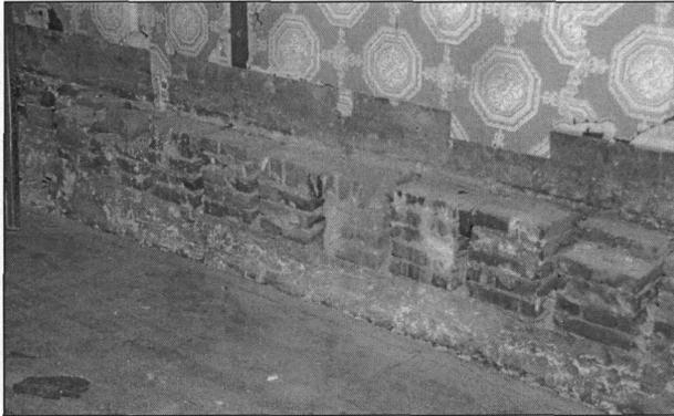
Figure 14: Dropped floor level, back of plan (note baseboard marks)
