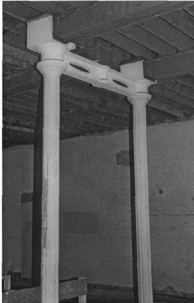
Figure 43: Second floor support column set
