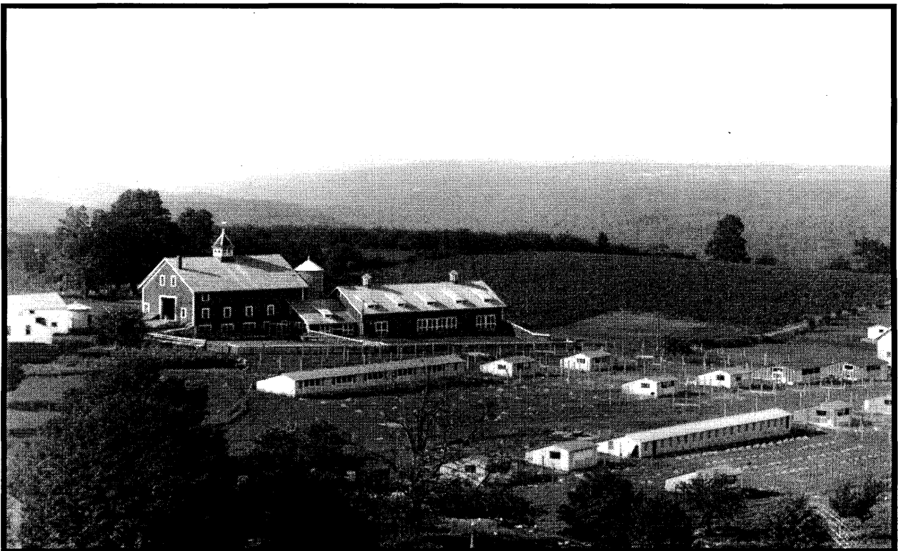
View of barn and setting, c.1920, looking northeast (Garrigus Collection, Dodd Center, University of Connecticut)
