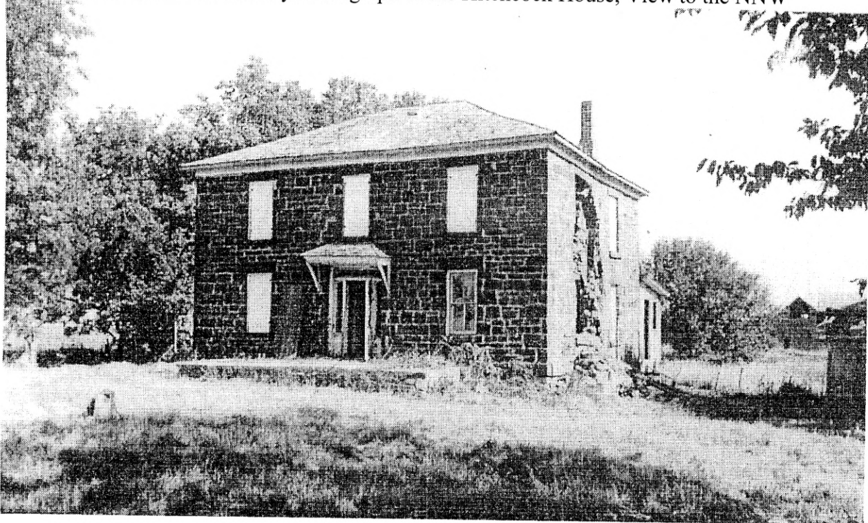
Mid-Late 20th Century Photograph of the Hitchcock House, View to the NNW
