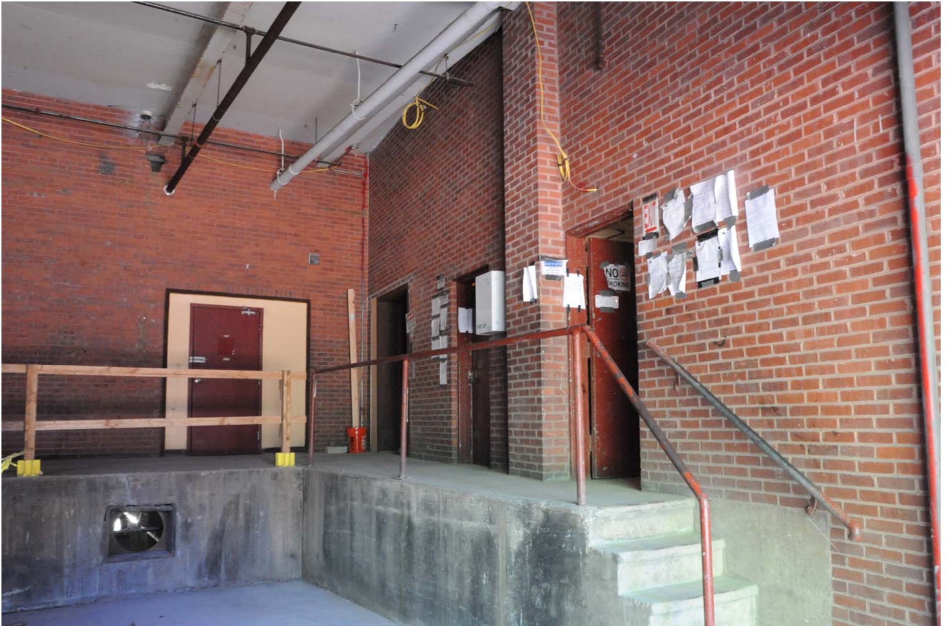
PA_Philadelphia County_Ortlieb Bottling House_0010
