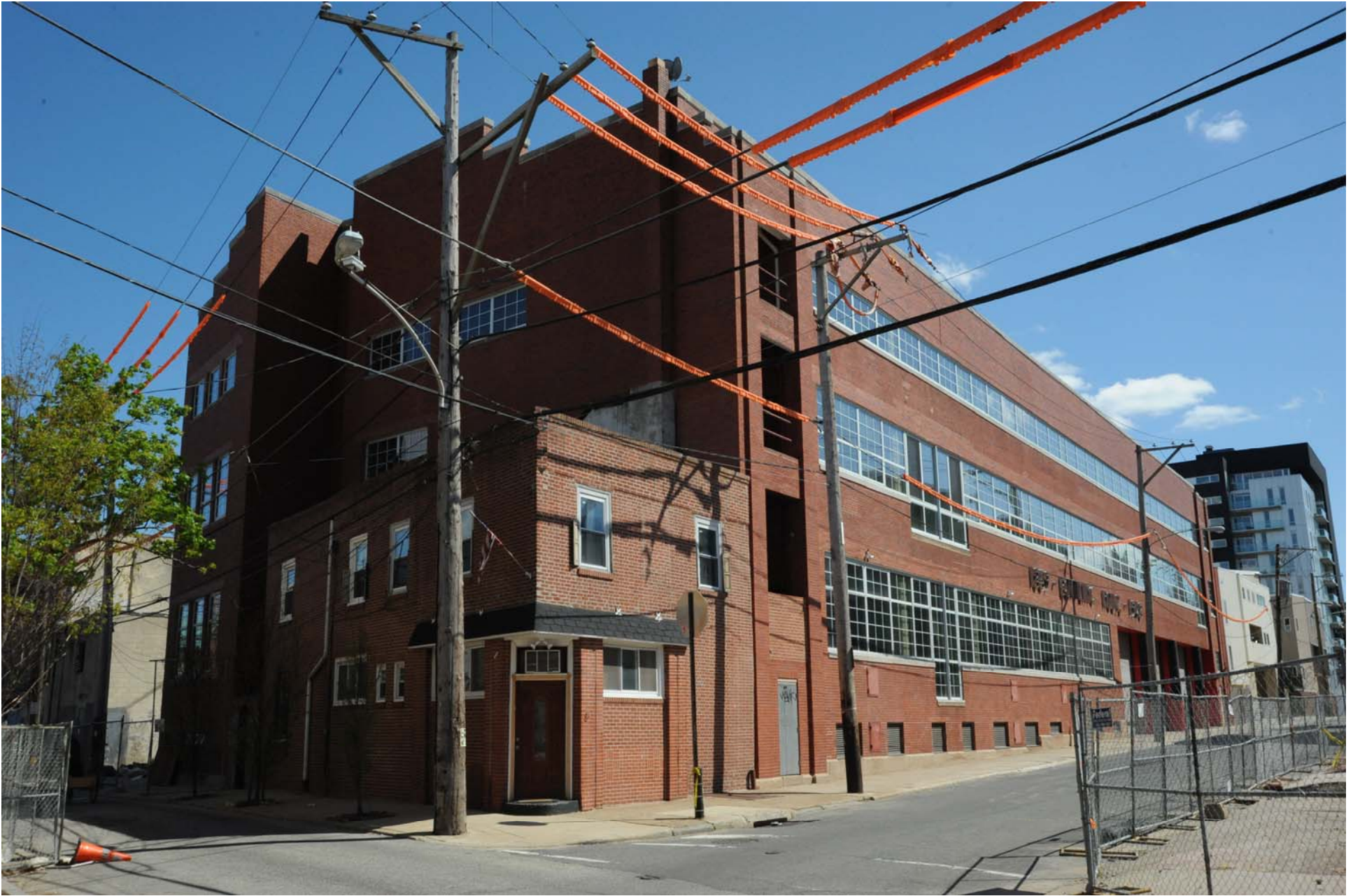
PA_Philadelphia County_Ortlieb Bottling House_0002
