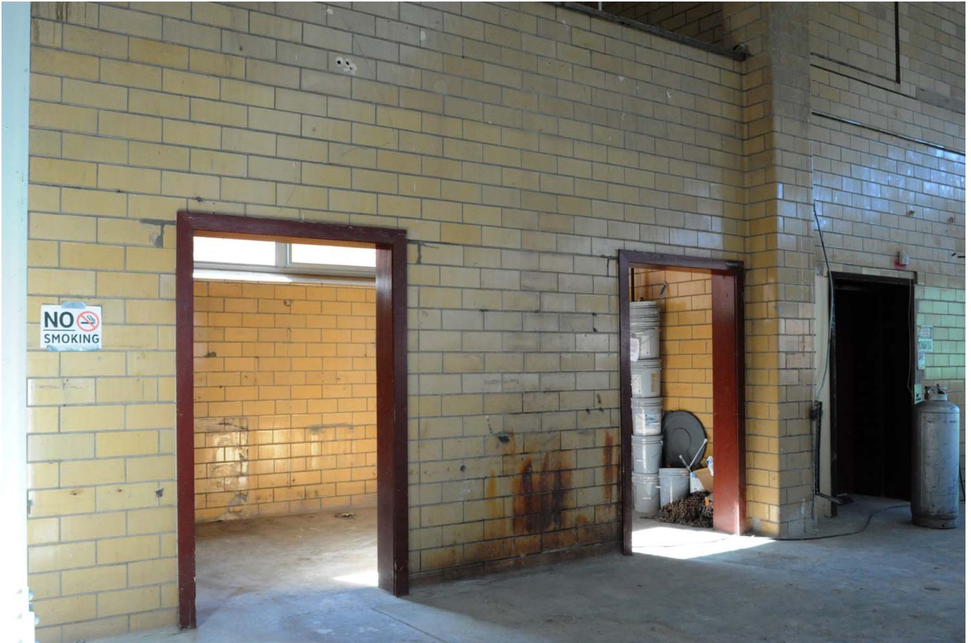
PA_Philadelphia County_Ortlieb Bottling House_0024
