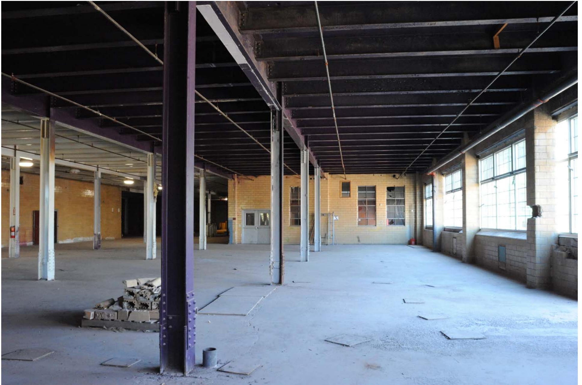
PA_Philadelphia County_Ortlieb Bottling House_0017
