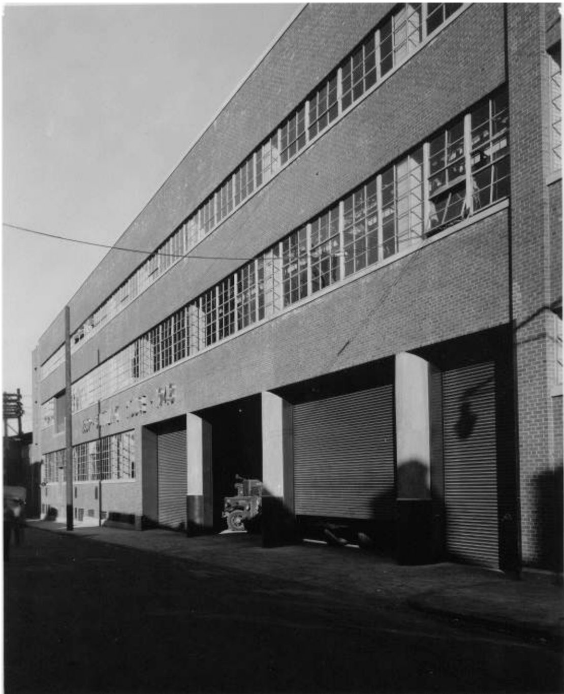
Figure 7: Historic view, c.1950, Ortlieb's Bottling House west elevation, looking northeast from southern end of building, showing historic extent of sash and former loading door at north end of first floor, as well as absence of southern second floor loading door. Courtesy Kieran Timberlake.
