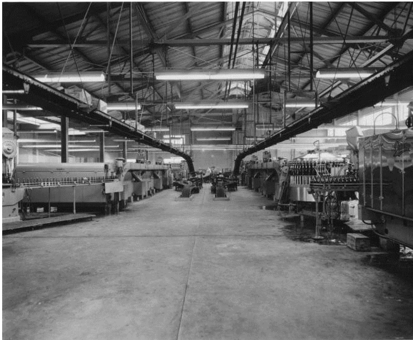
Figure 10: Historic view, c.1950, Ortlieb's Bottling House second floor interior, looking south from northern end of building, showing bottling machinery and conveyor system, including openings in floor, and half-height partition without openings at center rear. Courtesy Kieran Timberlake.
