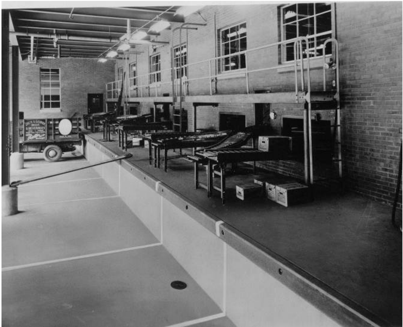
Figure 9: Historic view, c.1950, Ortlieb's Bottling House loading dock, looking northeast from southernmost bay, showing original configuration of openings in east wall, conveyors, elevated walkway, and single door into office area in north wall. Courtesy Kieran Timberlake.
