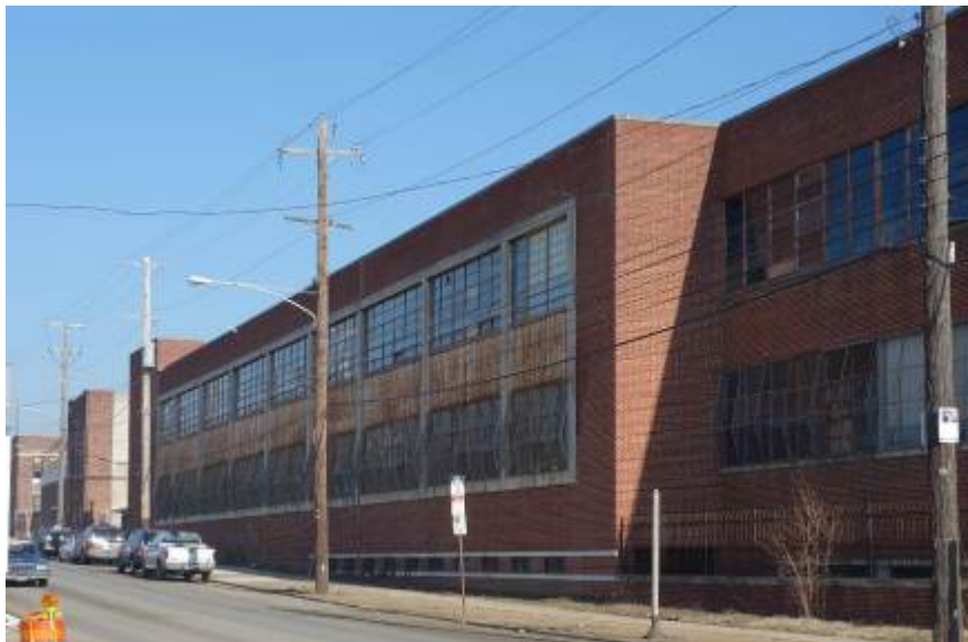
Figure 27: Budd Company Additions, c.1951-1954, Fox Street north of Hunting Park Avenue, Philadelphia. Photos: Emily T. Cooperman, 2013.
