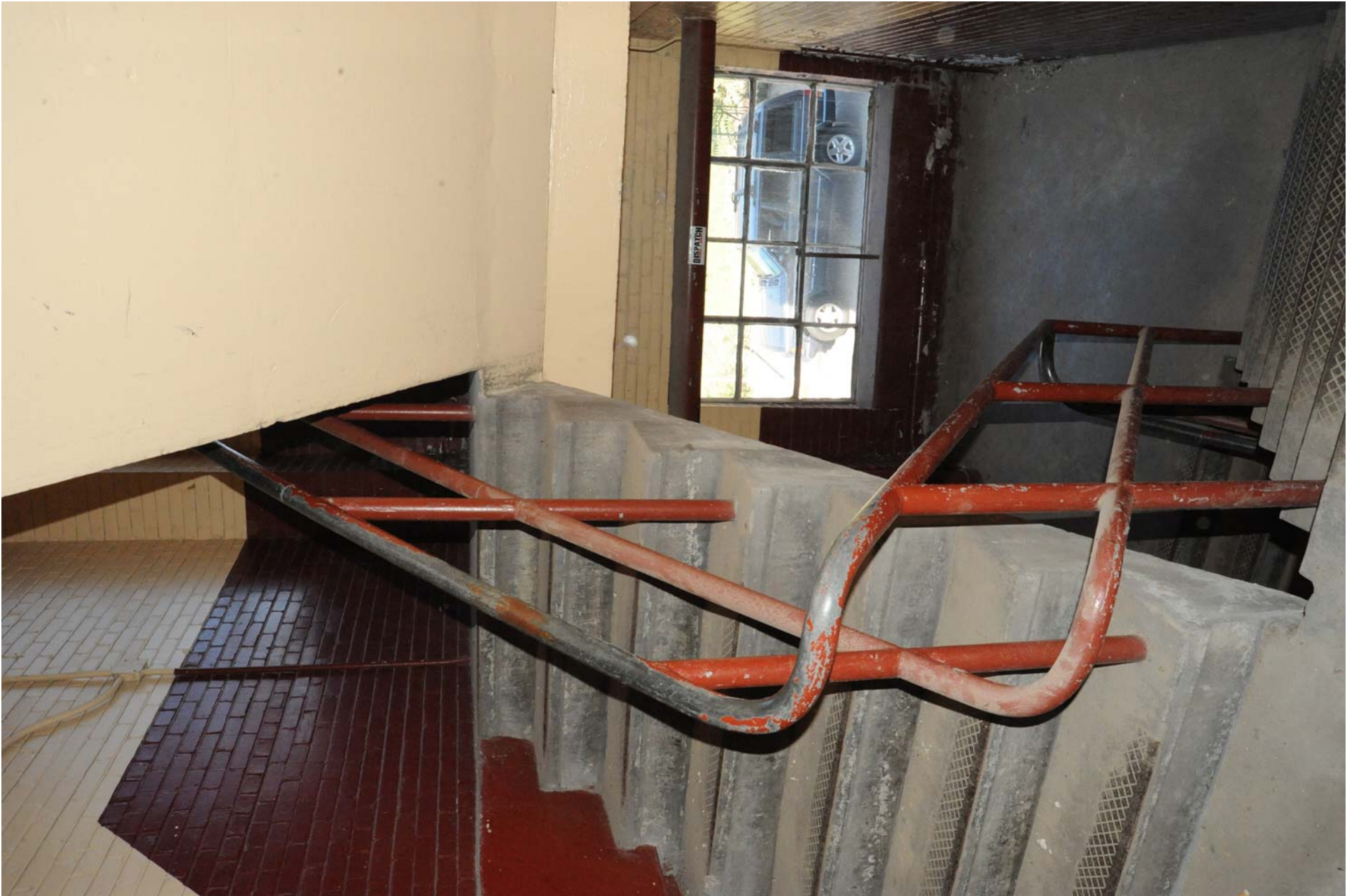
PA_Philadelphia County_Ortlieb Bottling House_0008
