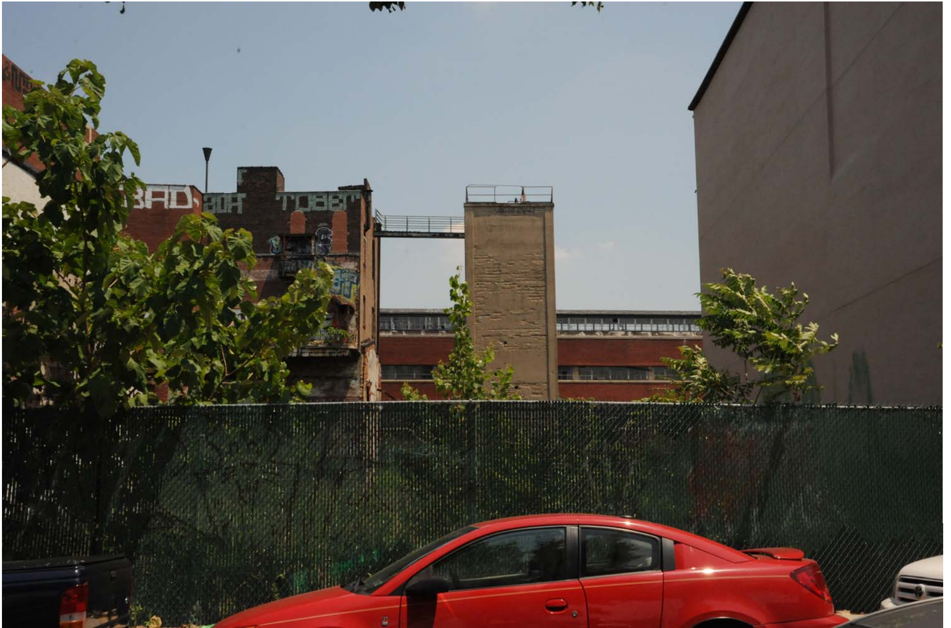
PA_Philadelphia County_Ortlieb Bottling House_0004
