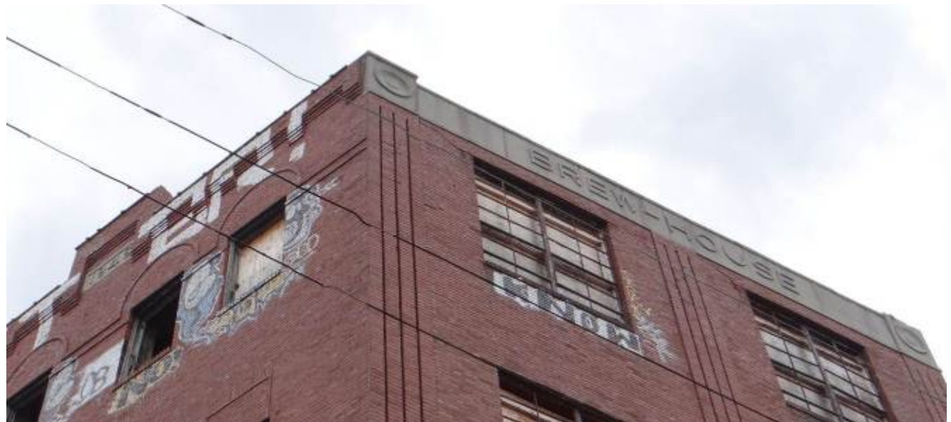
Figure 28: Cornice lines typical of former Ortliebs buildings, showing historic signage and Rundbogenstil decoration: top: 1913-14 (top) and 1946 sections (bottom) of the Brew House, north and east elevations.
