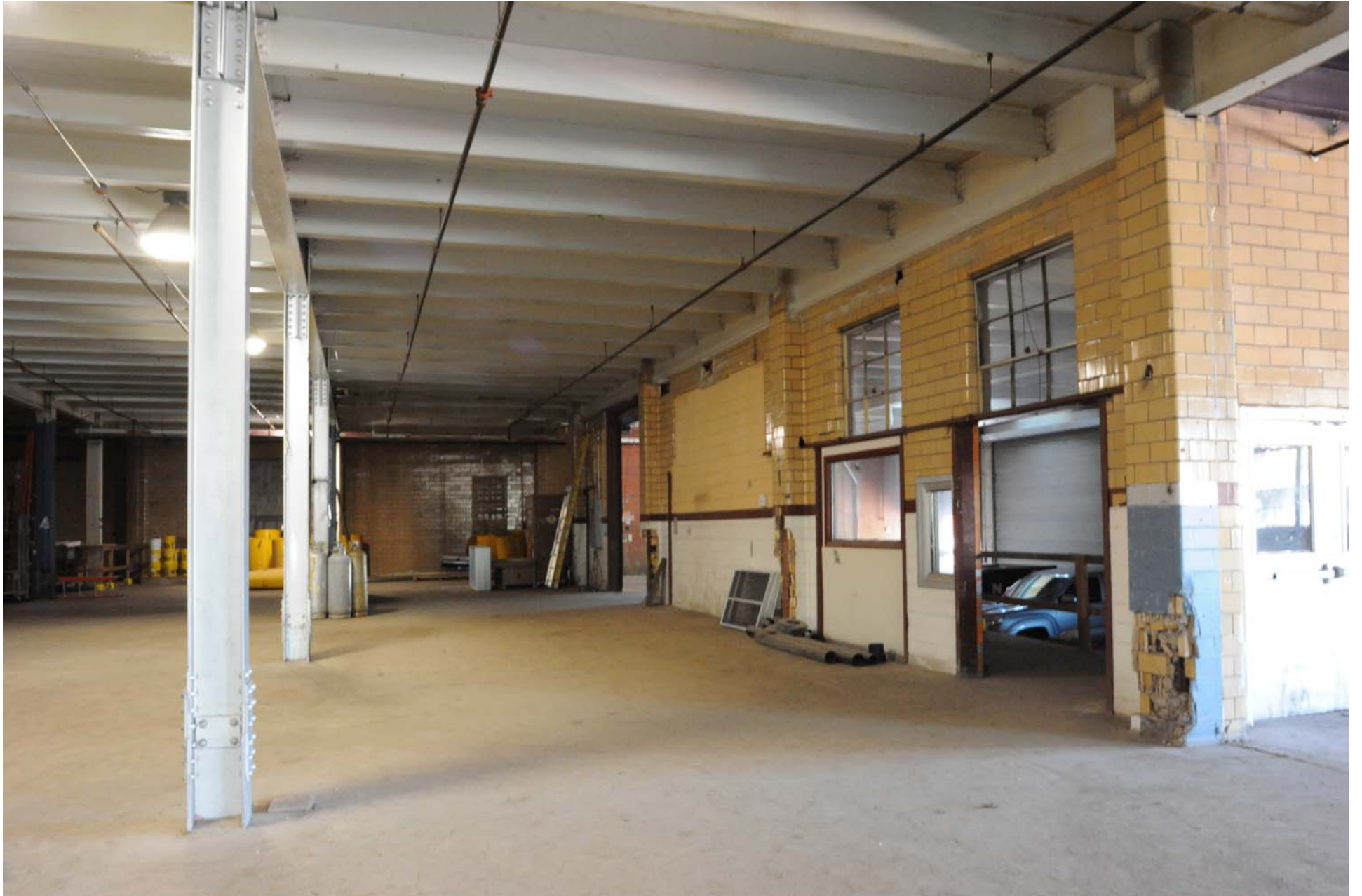
PA_Philadelphia County_Ortlieb Bottling House_0015
