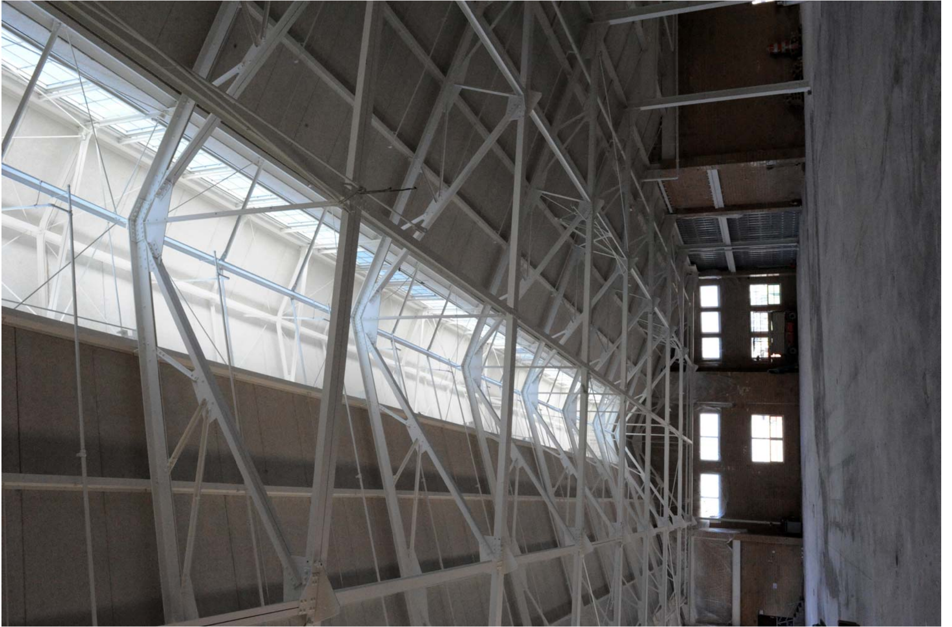
PA_Philadelphia County_Ortlieb Bottling House_0022
