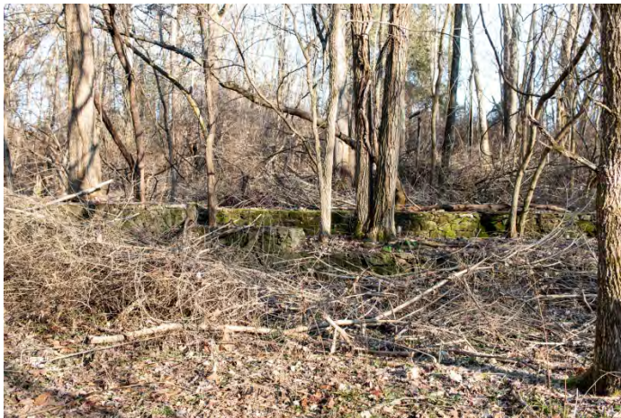
Hill House foundation ruins as seen today.
