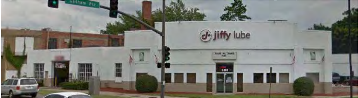
Figure 24. Sight Brothers Chevrolet Building at 3201 Gillham Plaza. Source: Google Maps 2016.
