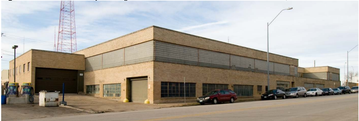
Figure 25. Aines Farm Dairy Building at 3110-30 Gillham Road. Source: Brad Finch, 2008.
