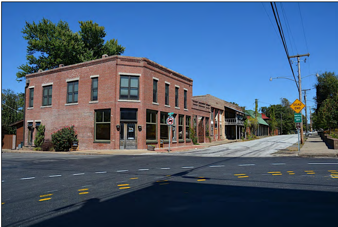
Photo 4. Oak Street from Main Street; facing northeast.
