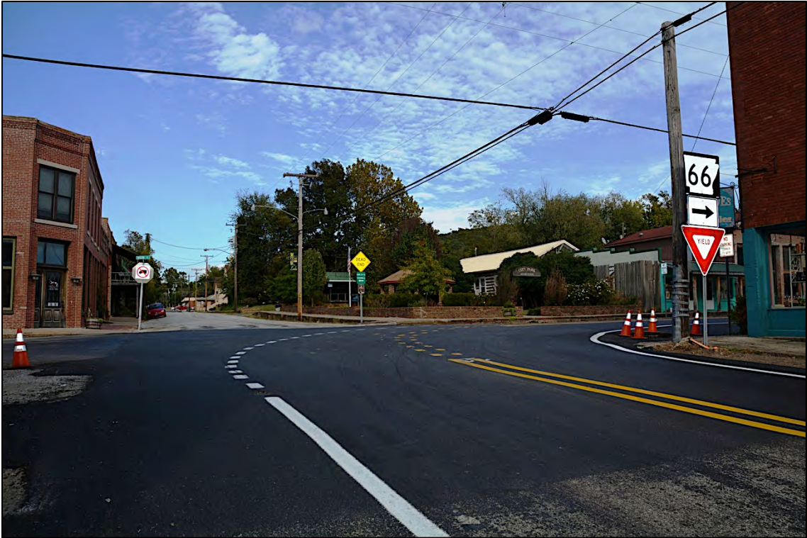
Photo 2. Intersection at Oak and Main Streets; facing southeast.
