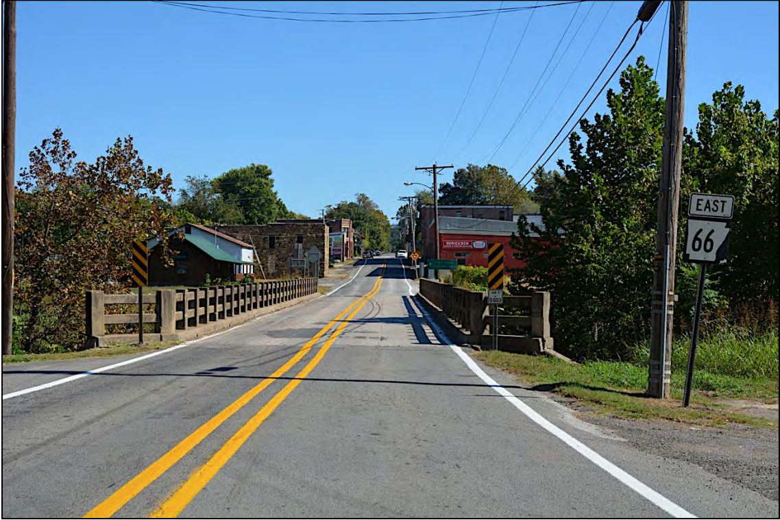
Photo 1. Oak Street from U.S. Highway 65; facing east.
