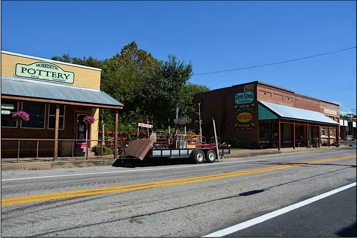
Photo 21. Eastern side of southern end of Main Street; facing southeast.
