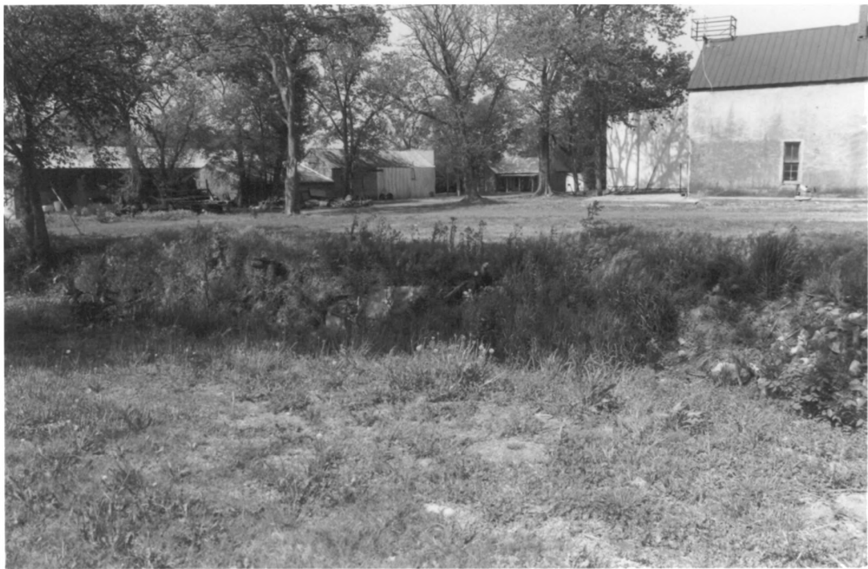
Washington Co. Kingpost Bridge Washington Co., Kansas
