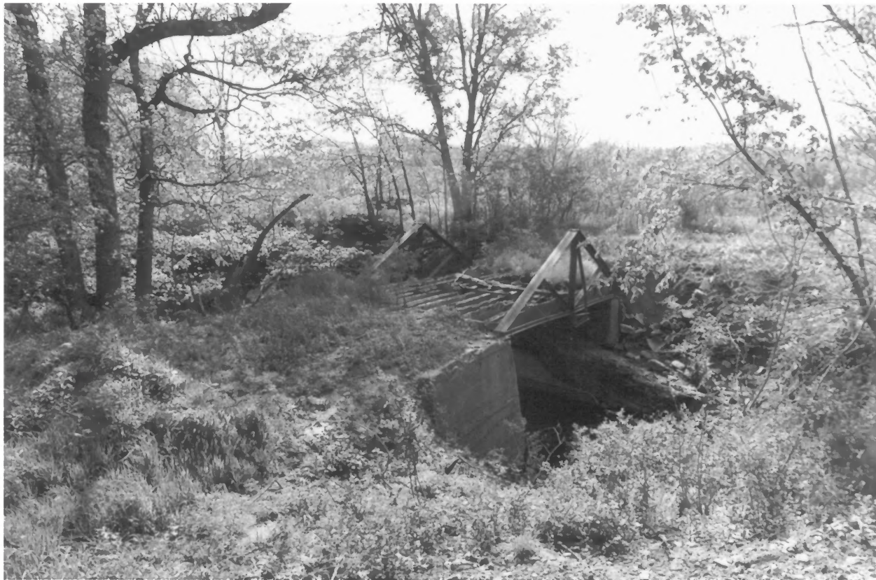
Washington Co. Kingpost Bridge Washington Co., Kansas
