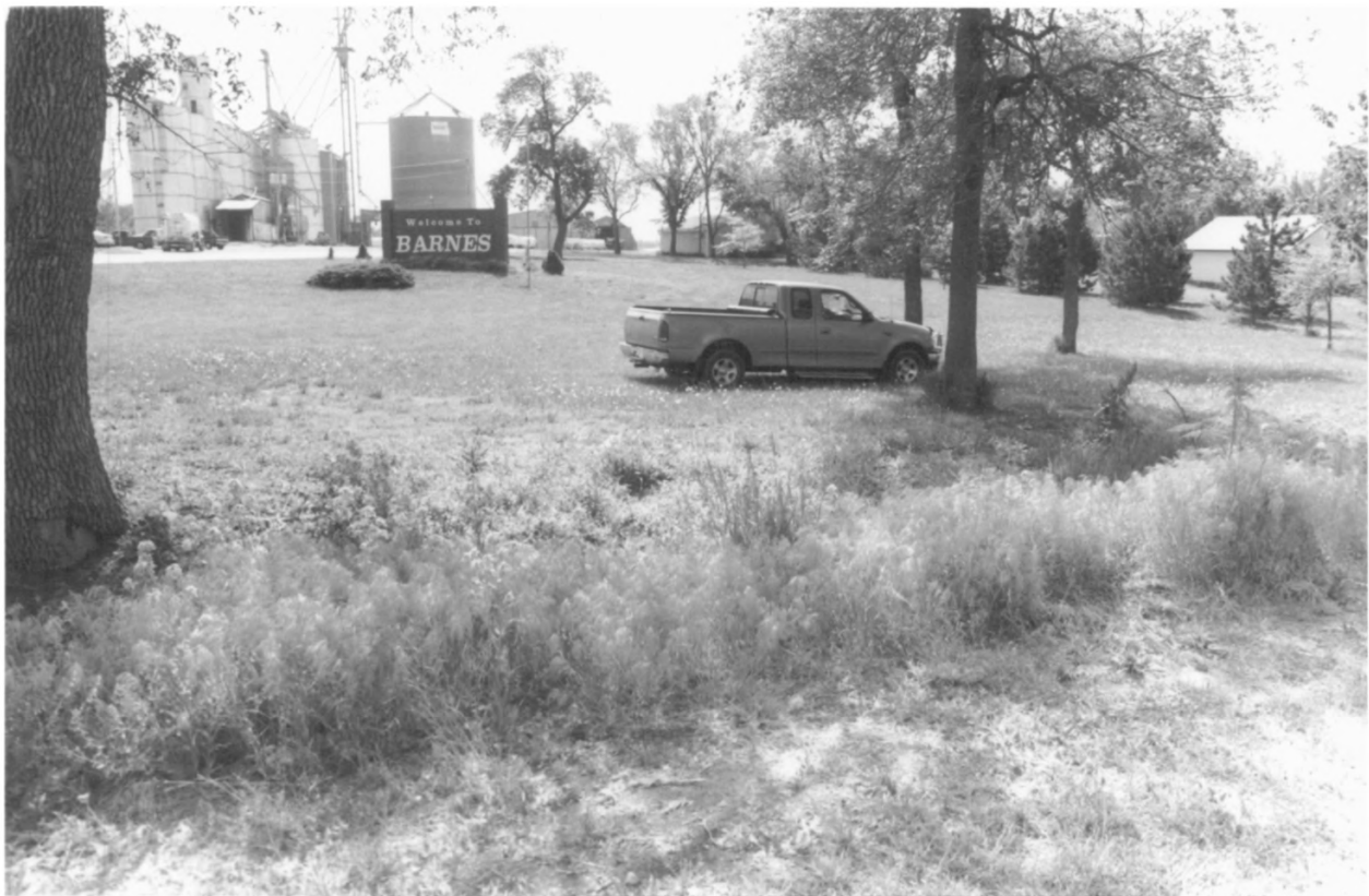
Washington Co. Kingpost Bridge #4 Washington Co., Kansas
