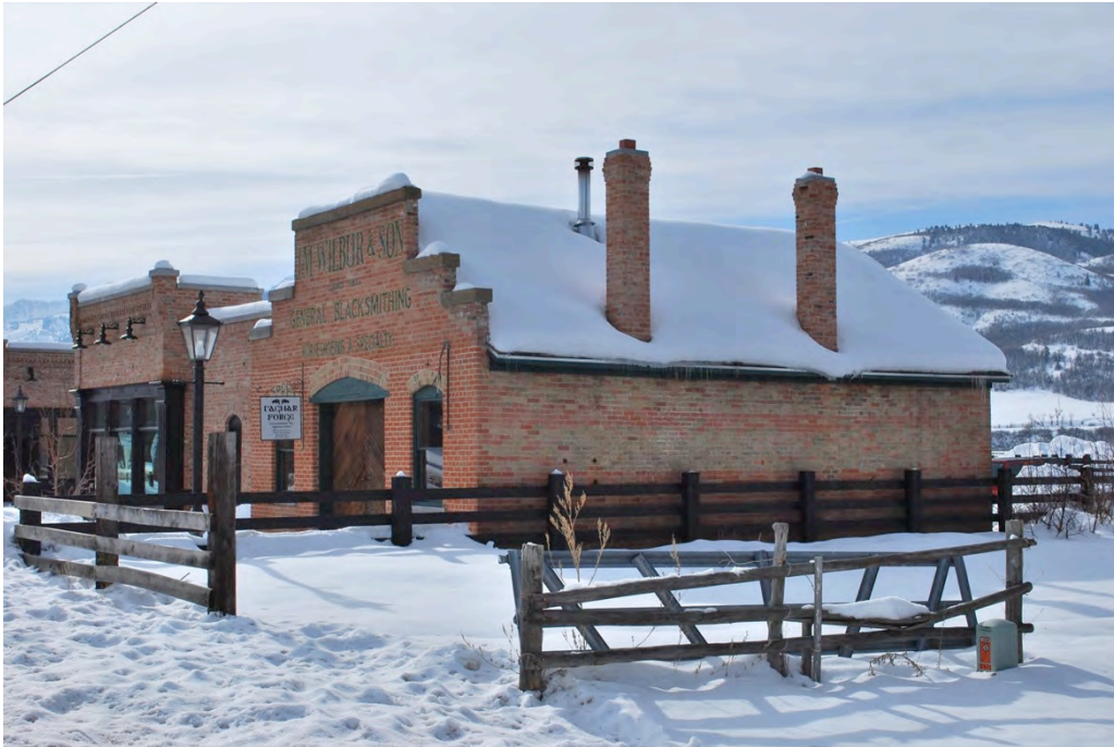
4 of 17: North and east elevations of blacksmith and new adjacent building. Camera facing southwest.
