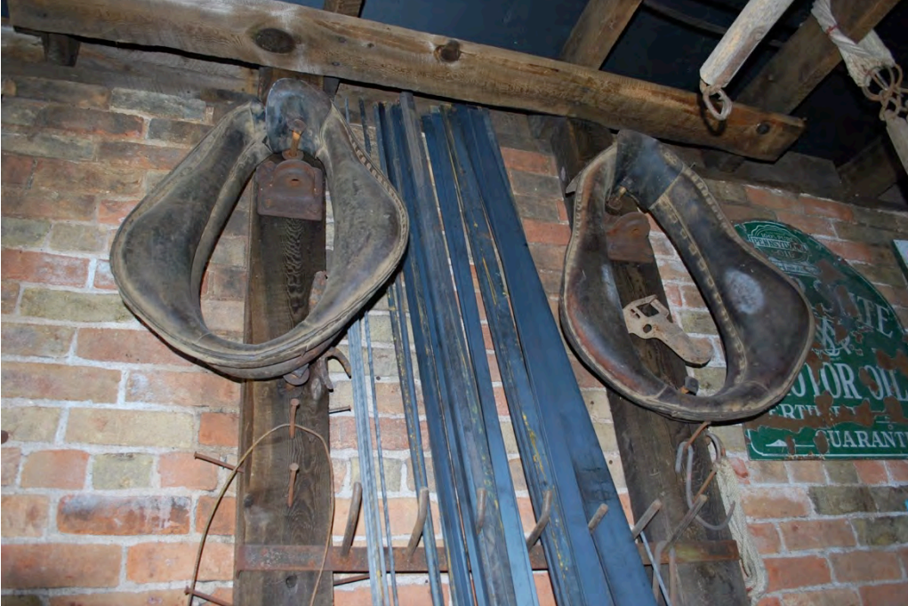
16 of 17: Interior detail view of stall posts with hinge remnants. Camera facing southwest.
