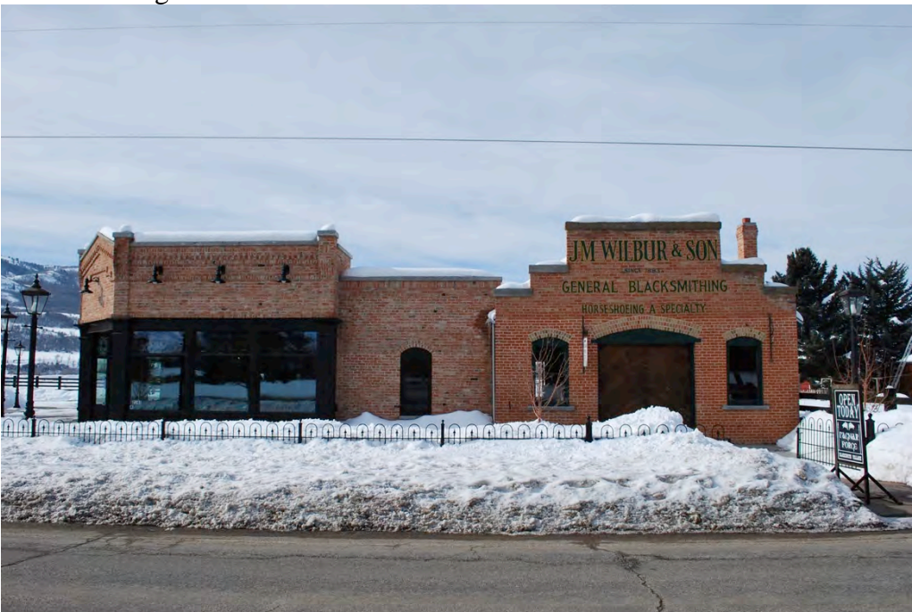
3 of 17: Context view of blacksmith with new adjacent commercial building, east elevations. Camera facing west.
