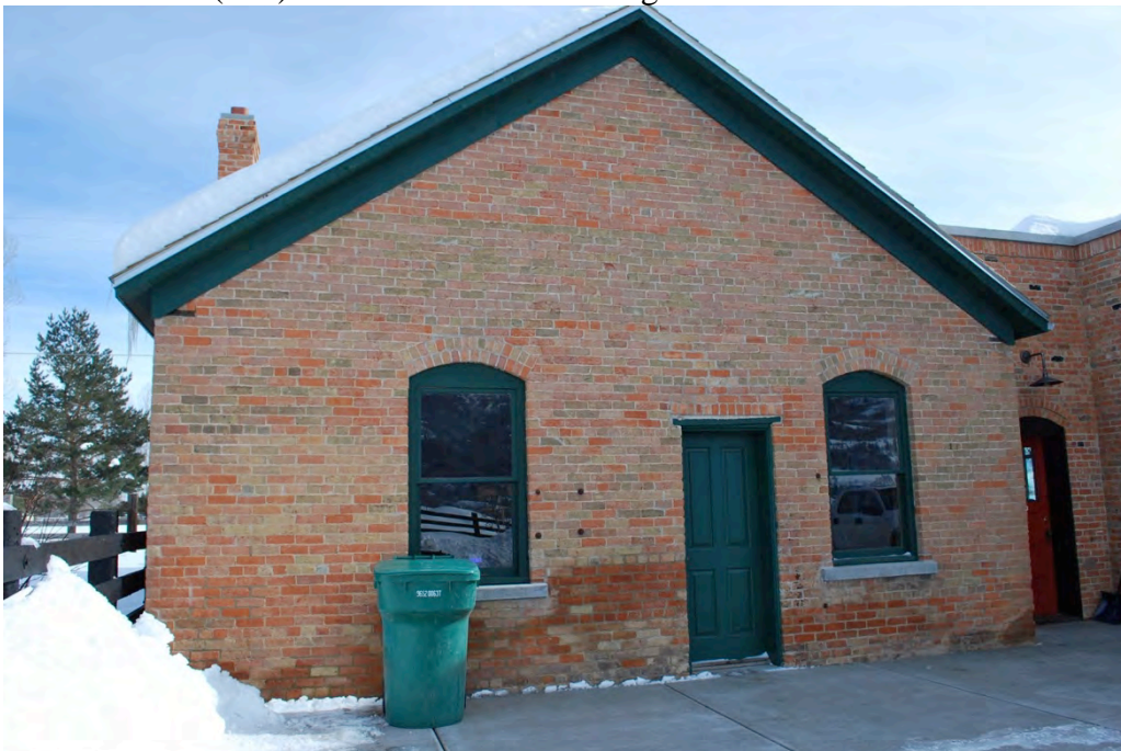
5 of 17: West (rear) elevation. Camera facing east.
