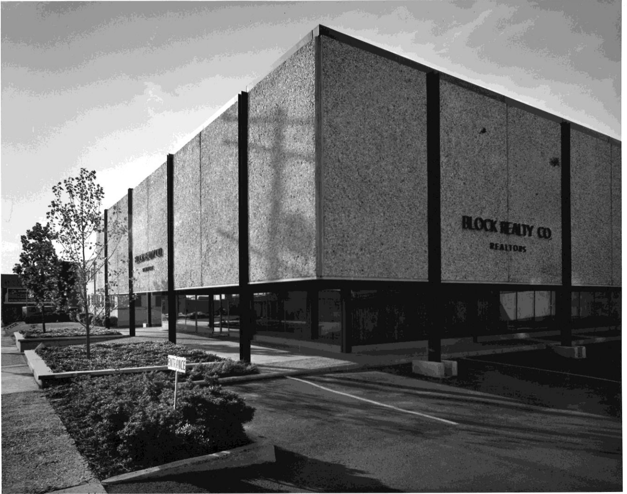
Figure 3: North and west façades of the Block Realty Building, looking southeast, 1965.
