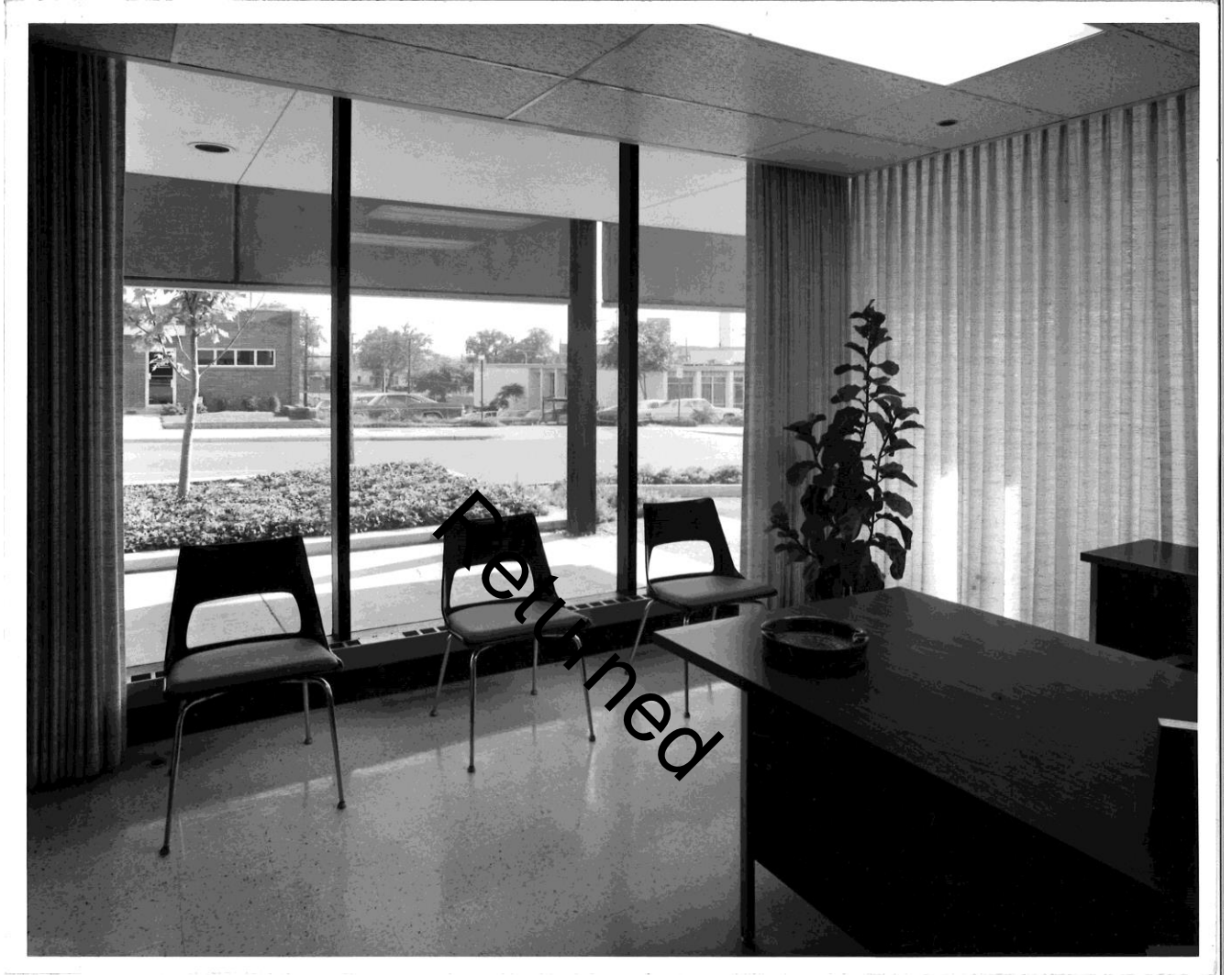
Figure 2: Office in the northeast corner of the first floor of the Block Realty Building, looking northeast, 1965.
