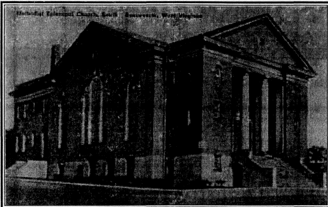
Fig. 10 The Methodist Episcopal Church of 1922 (Resource No. 229), from an early post card view.
