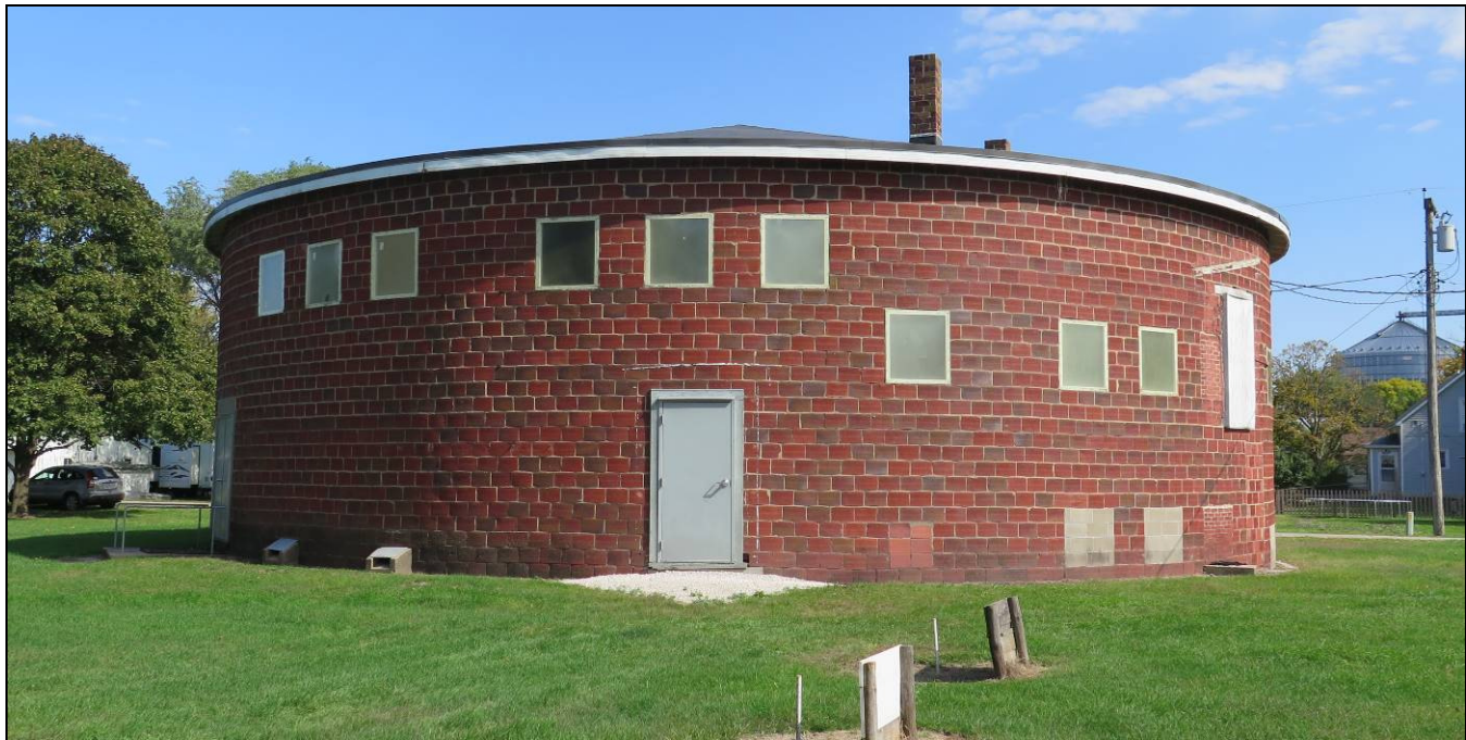
Figure 5. Southeast side of Yale High School Gymnasium showing windows replaced with Plexiglas panes and tile block and concrete block filled windows below. The former catwalk entrance is to the right side of the building in this view, which is looking to the ENE. Some of the basement vents are visible at ground level on the left side of the building. Photograph taken by Leah Rogers, Tallgrass Archaeology LLC, October 9, 2017.
