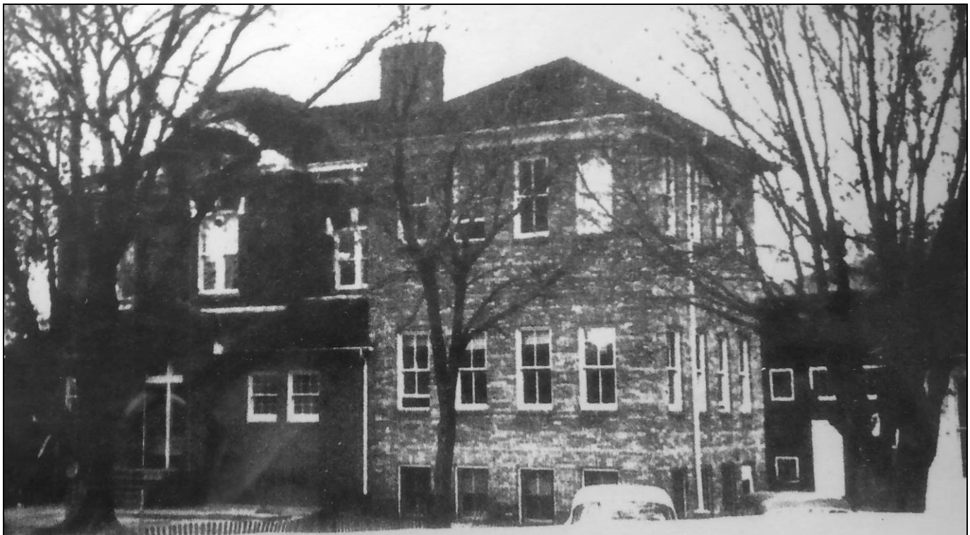
Figure 21. Post-1932 photographs of the Yale High School with a portion of the round gymnasium visible in the background to the right in these views looking north (top) and north-northeast (bottom). Sources: Fox 1982 (top) and digital scan provided by Brandon Godwin, City of Yale, 2018 (bottom).
