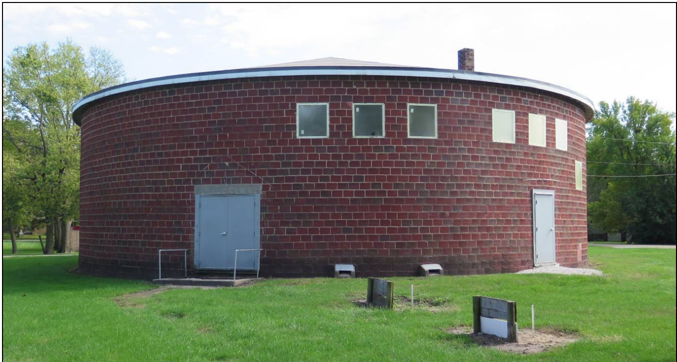
Figure 3. Yale High School Gymnasium looking ESE.
