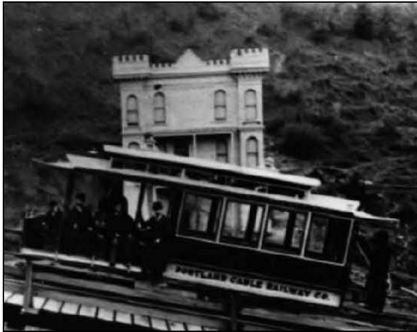
Image 15. The Alice Druhot House, also known as the Cable House, ca. 1890. Image courtesy of Oregon Historical Society (ORHI 9008).
