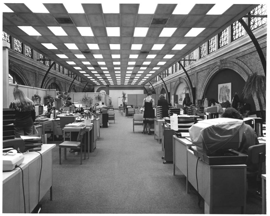
3rd Floor office South wing of Ferry Building. Note the original brick archs and windows. Braces were added later, perhaps after 1906 Earth quake. Photo taken 1977
