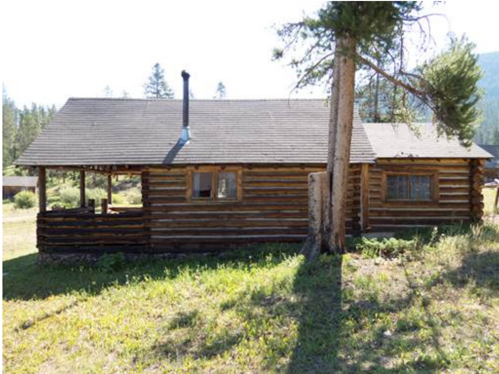
MT_GallatinCounty_ElkhornRanchHistoricDistrict_0057 Feature #14, Prospector west elevation, camera facing east.
