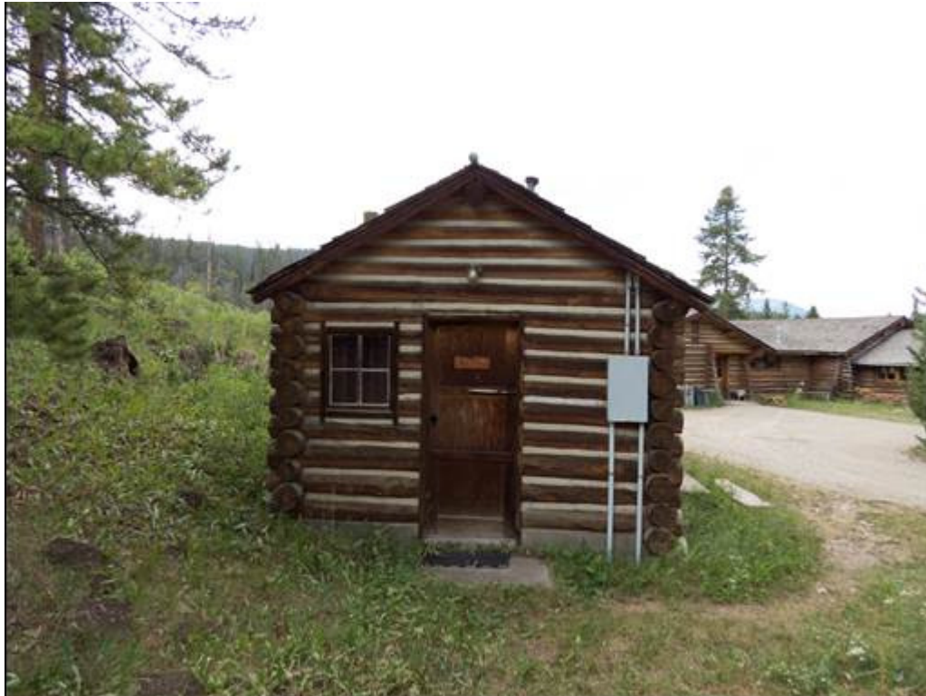
MT_GallatinCounty_ElkhornRanchHistoricDistrict_0086 Feature #22, Crew Bathrooms east elevation, camera facing west.
