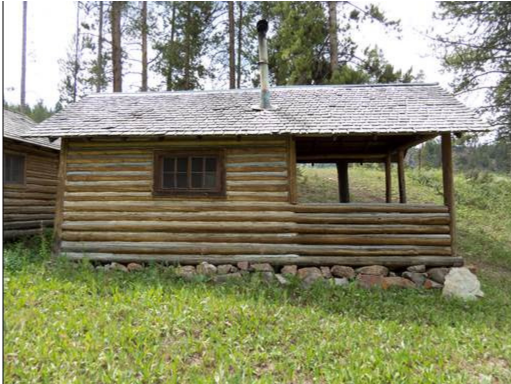
MT_GallatinCounty_ElkhornRanchHistoricDistrict_0090 Feature #23, Lean To east elevation, camera facing west.
