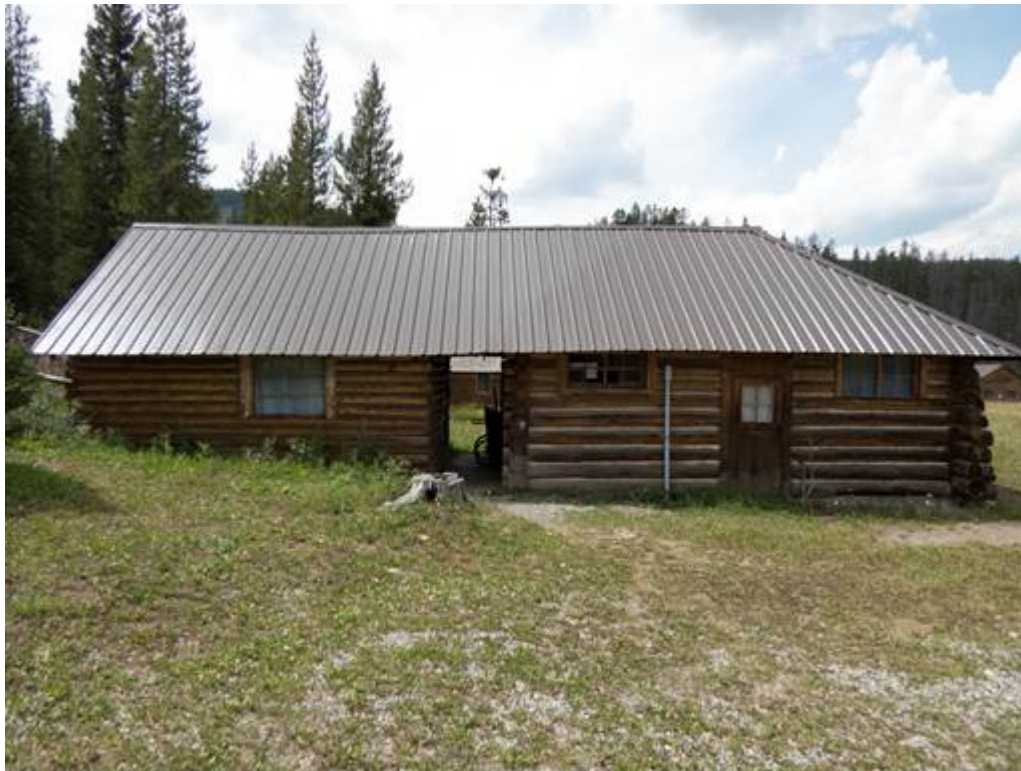
MT_GallatinCounty_ElkhornRanchHistoricDistrict_0041 Feature #11, Washhouse east elevation, camera facing west.
