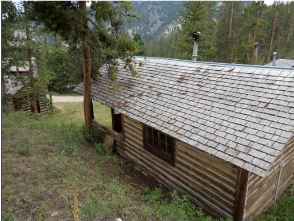
MT_GallatinCounty_ElkhornRanchHistoricDistrict_0093 Feature #23, Lean To west elevation, camera facing northwest.
