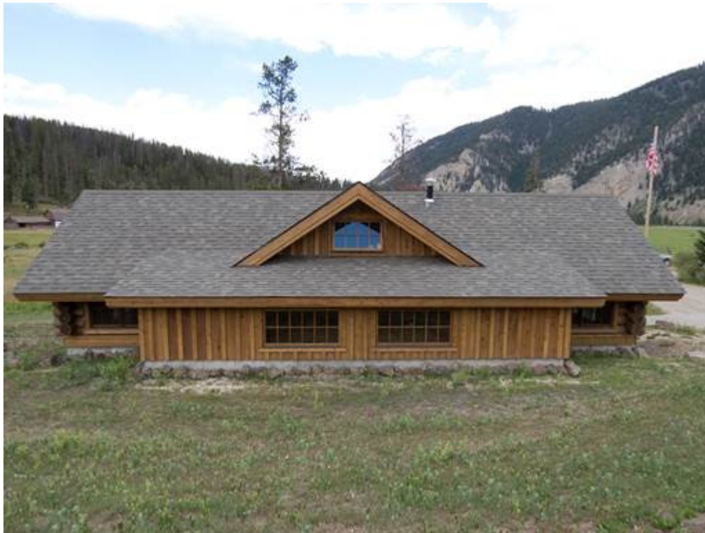
MT_GallatinCounty_ElkhornRanchHistoricDistrict_0008 Feature #2, Office south elevation, camera facing north.
