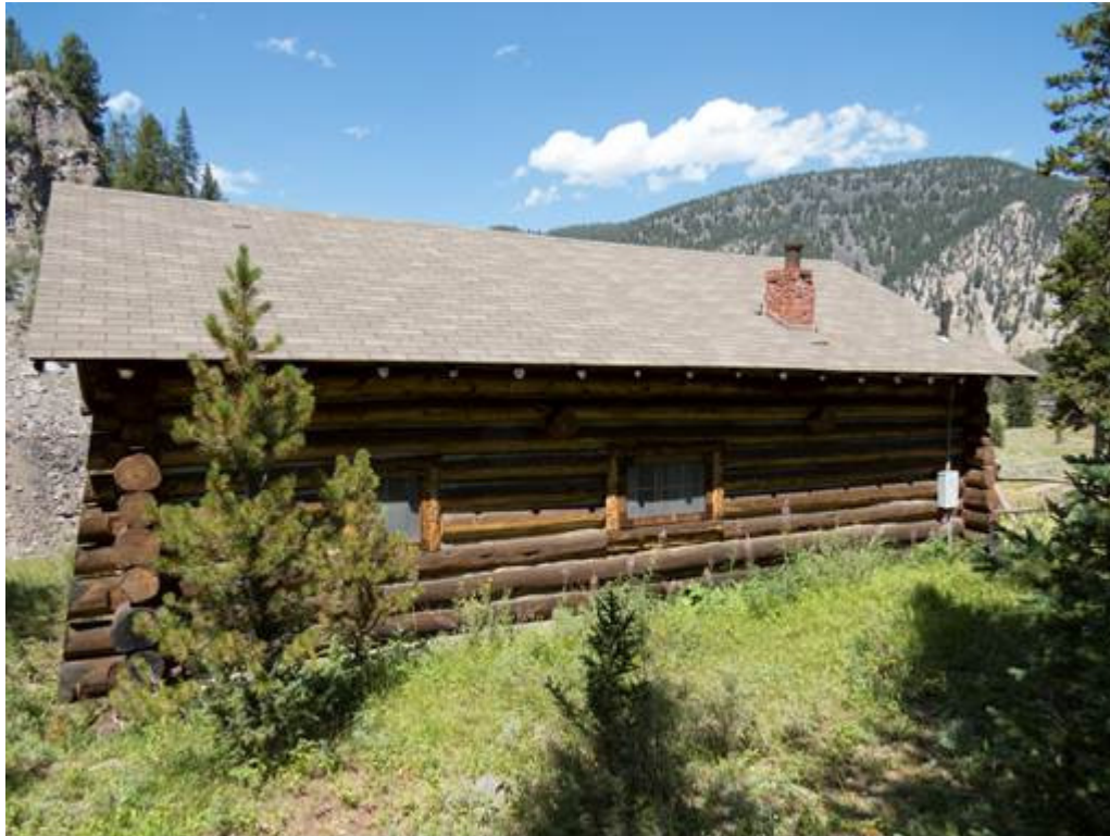
MT_GallatinCounty_ElkhornRanchHistoricDistrict_0019 Feature #5, Highpoint south elevation, camera facing north.
