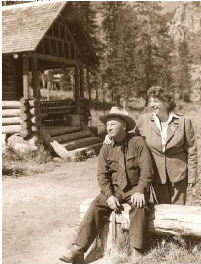
Figure 6. The porch of the Old Office is shown in its original location behind Ernest and Grace Miller, founders of the Elkhorn Ranch, in this photograph from the 1940s. Note the modified queen post multi-chord gable truss, a distinctive element that occurs on many ranch buildings.
