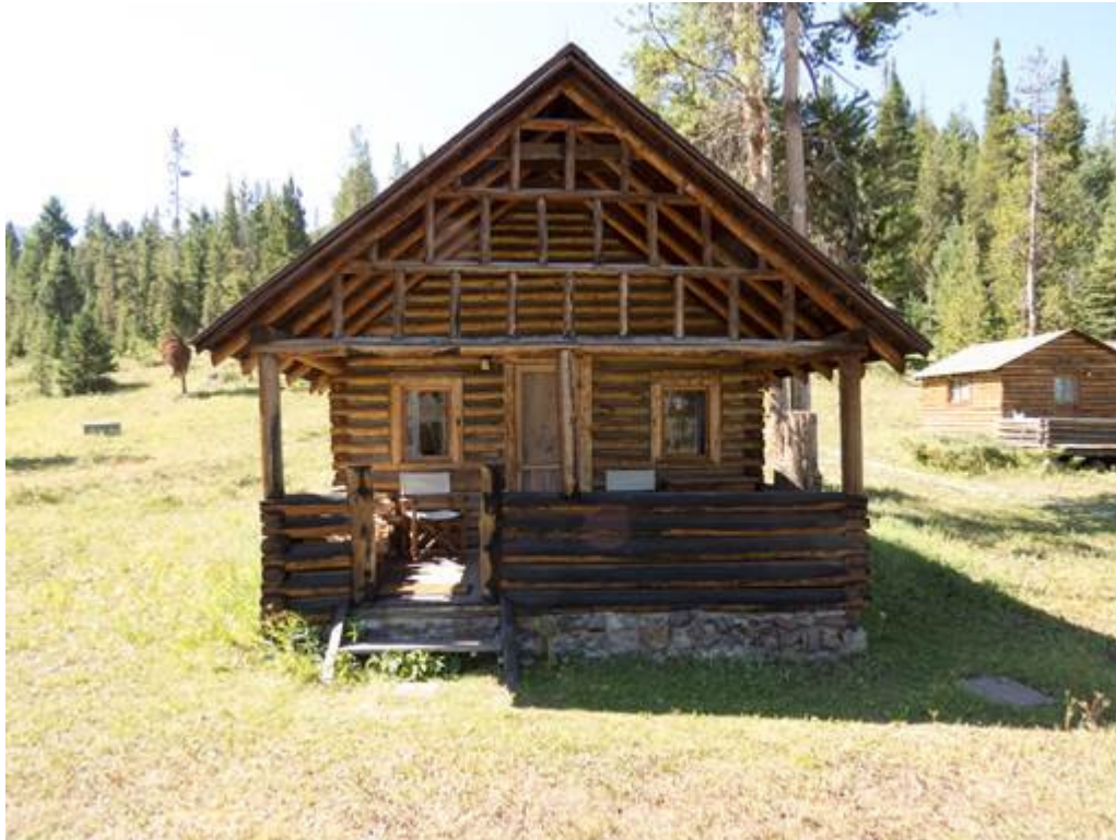
MT_GallatinCounty_ElkhornRanchHistoricDistrict_0054 Feature #14, Prospector, north façade, camera facing south.
