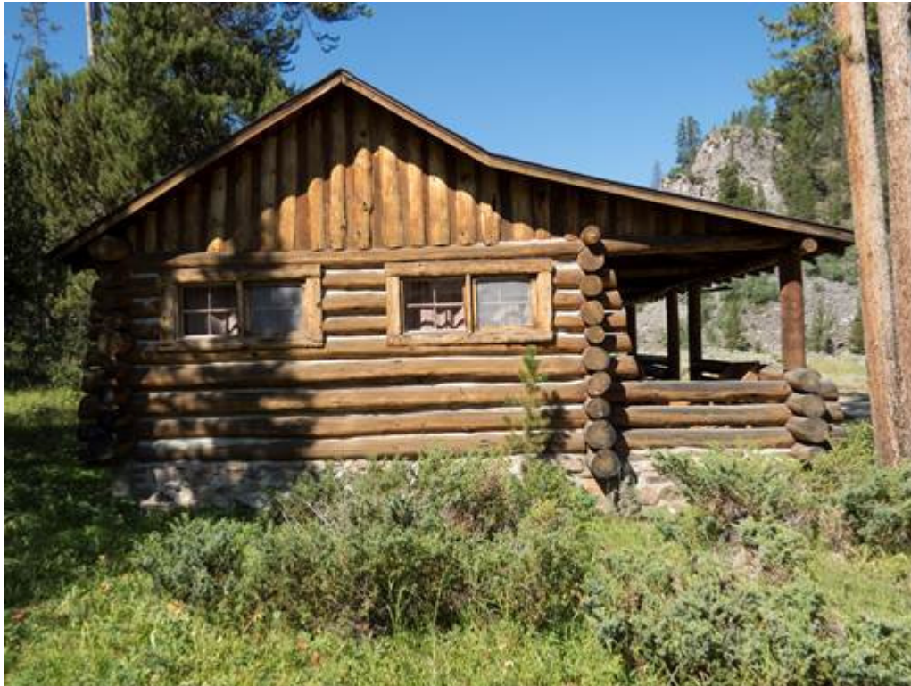
MT_GallatinCounty_ElkhornRanchHistoricDistrict_0025 Feature #7, Squaw east elevation, camera facing west.
