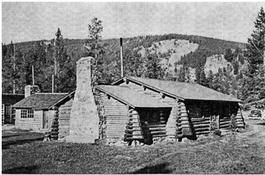
Figure 8. This circa 1950 photograph shows on the extreme left the door to the old store room and the 1923 fireplace added to the original homestead cabin. Center and right of the photograph shows the Guest Dining Room added during the Great Depression.
