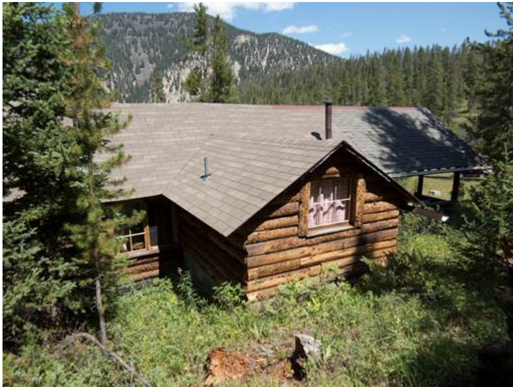
MT_GallatinCounty_ElkhornRanchHistoricDistrict_0051 Feature #13, B.O.Q. south elevation, camera facing north.
