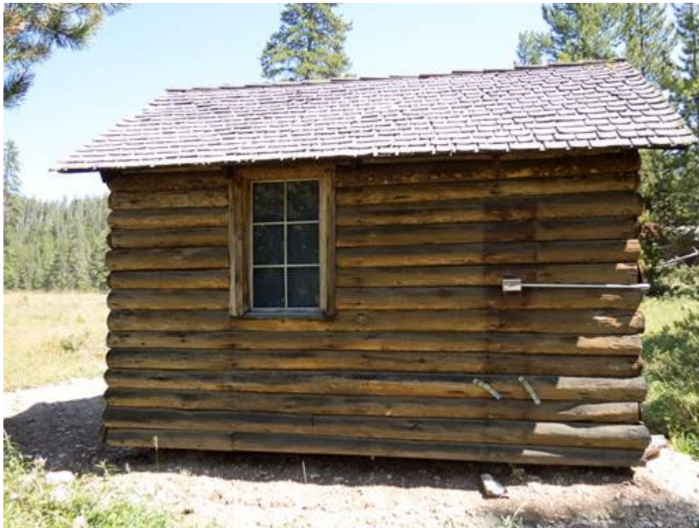
MT_GallatinCounty_ElkhornRanchHistoricDistrict_0040 Feature #10, Trappers Cabin west elevation, camera facing east.
