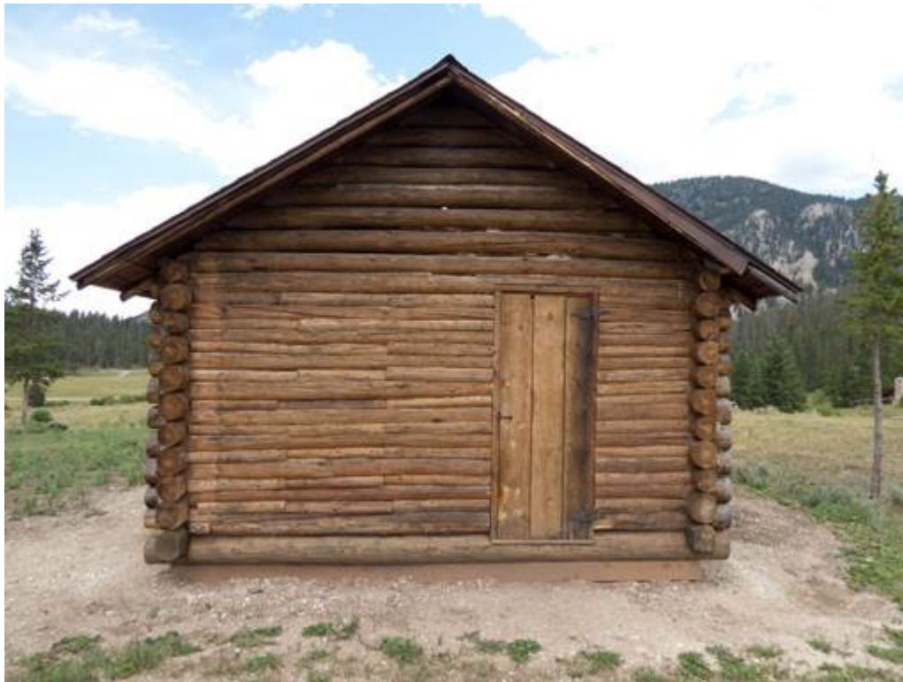
MT_GallatinCounty_ElkhornRanchHistoricDistrict_0011 Feature #3, Old Office south elevation, camera facing north.
