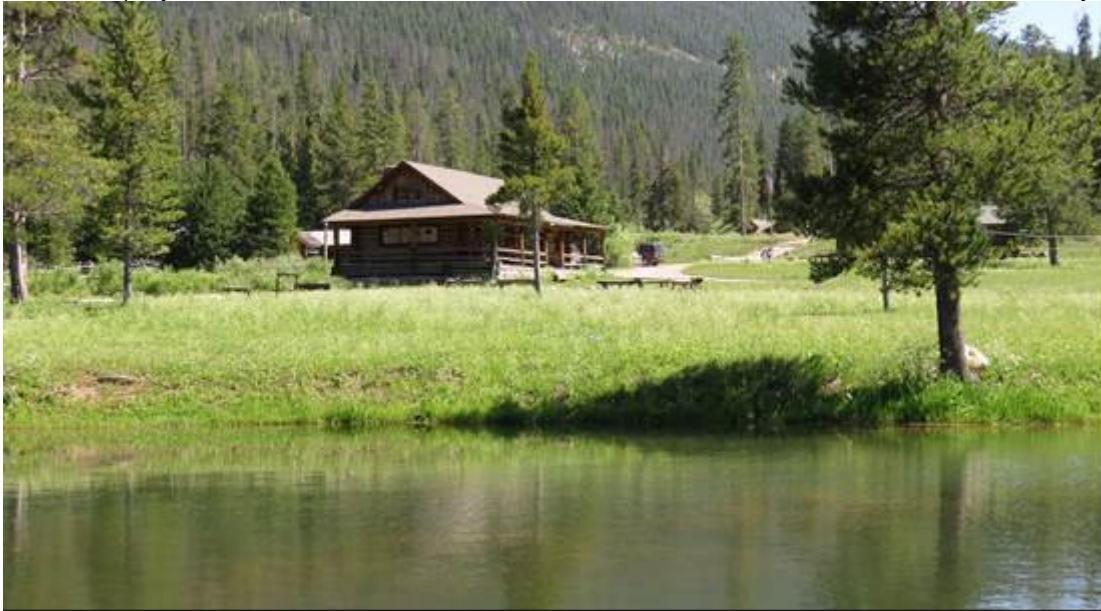
Figure 2. Overview (to south) of Pond and Recreation Hall (2014).
