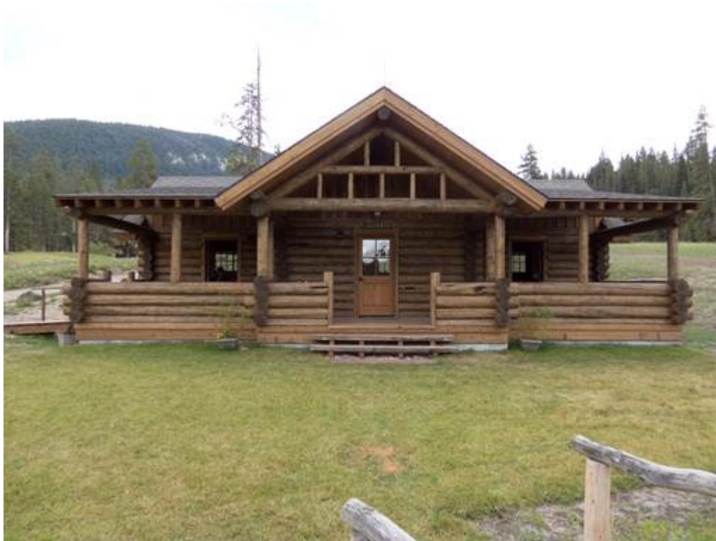
MT_GallatinCounty_ElkhornRanchHistoricDistrict_0006 Feature #2, Office north elevation, camera facing south.
