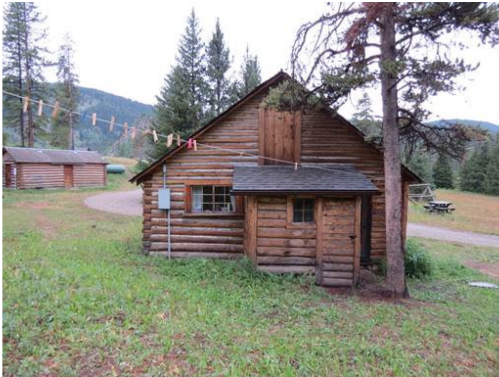
MT_GallatinCounty_ElkhornRanchHistoricDistrict_0104 Feature #27, Turnabout east elevation, camera facing west.
