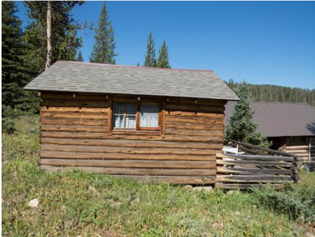
MT_GallatinCounty_ElkhornRanchHistoricDistrict_0045 Feature #12, Hiawatha east elevation, camera facing west.
