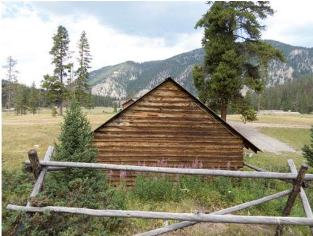
MT_GallatinCounty_ElkhornRanchHistoricDistrict_0043 Feature #11, Washhouse south elevation, camera facing north.
