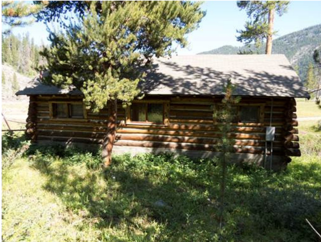
MT_GallatinCounty_ElkhornRanchHistoricDistrict_0027 Feature #7, Squaw south elevation, camera facing north.
