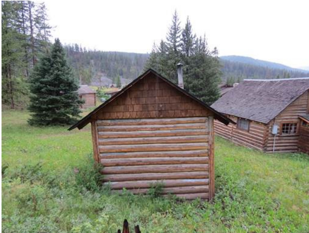
MT_GallatinCounty_ElkhornRanchHistoricDistrict_0100 Feature #26, Papoose east elevation, camera facing west.
