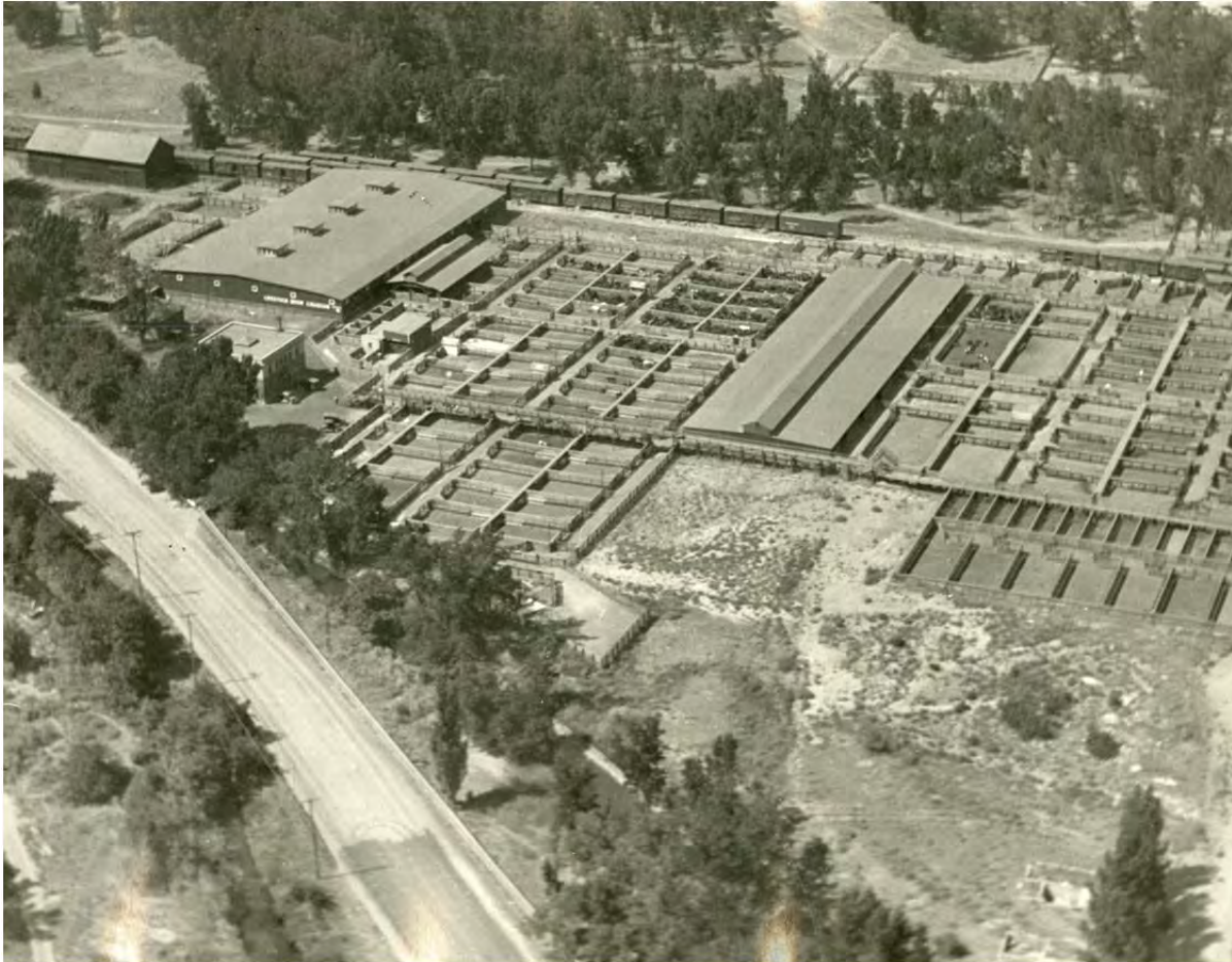
Figure 5 C. 1922-31 aerial of stockyard, prior to construction of the Exchange Building.
