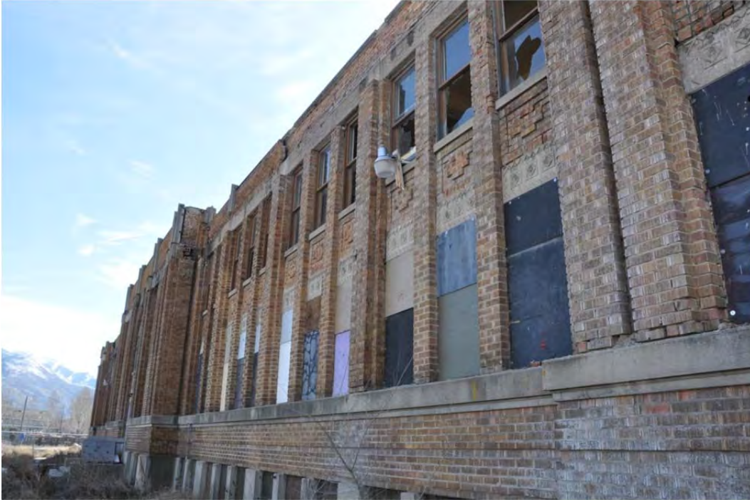
Photograph 7 of 13 North elevation. Camera facing southeast.
