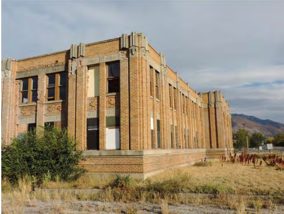
Photograph 3 of 13 South and west elevations. Camera facing northeast.
