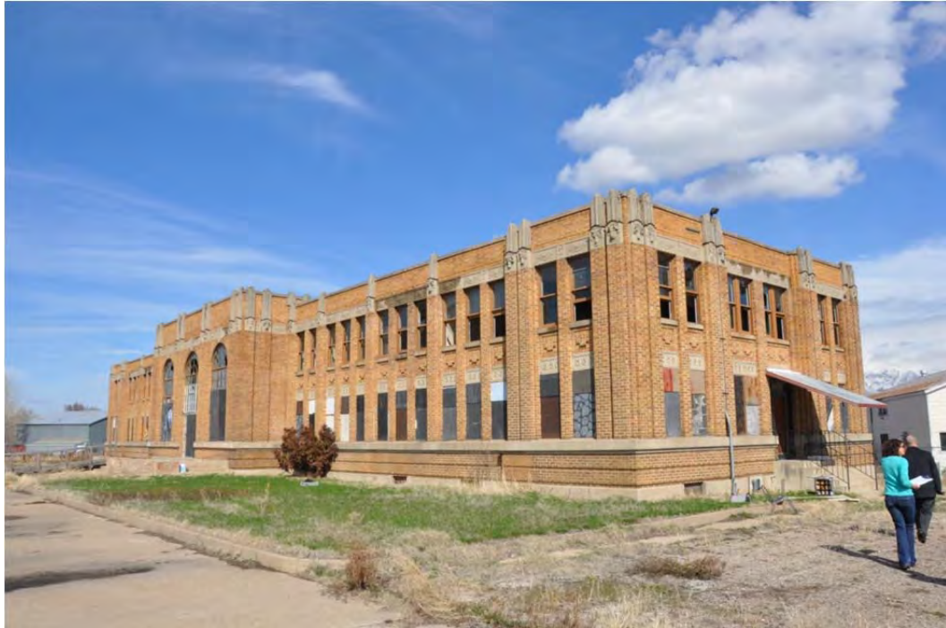
Photograph 1 of 13 South and east elevations. Camera facing northwest.
