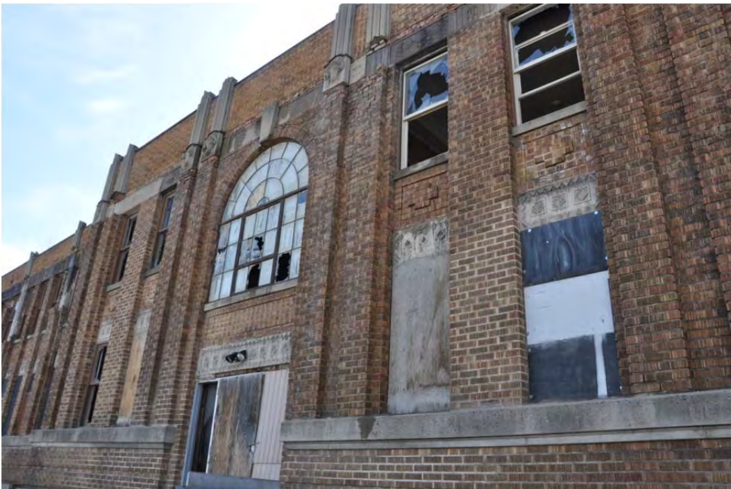
Photograph 8 of 13 Entry way, north elevation. Camera facing southeast.
