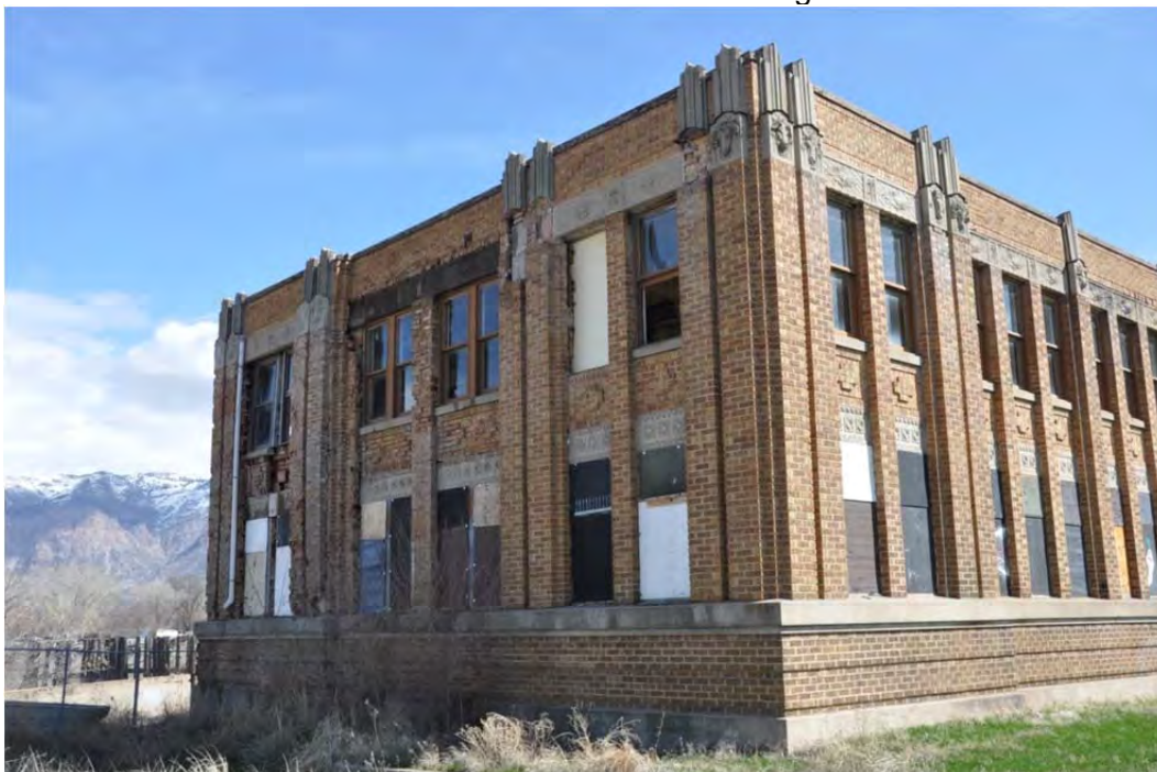
Photograph 4 of 13 South and west elevations, detail. Camera facing northeast.
