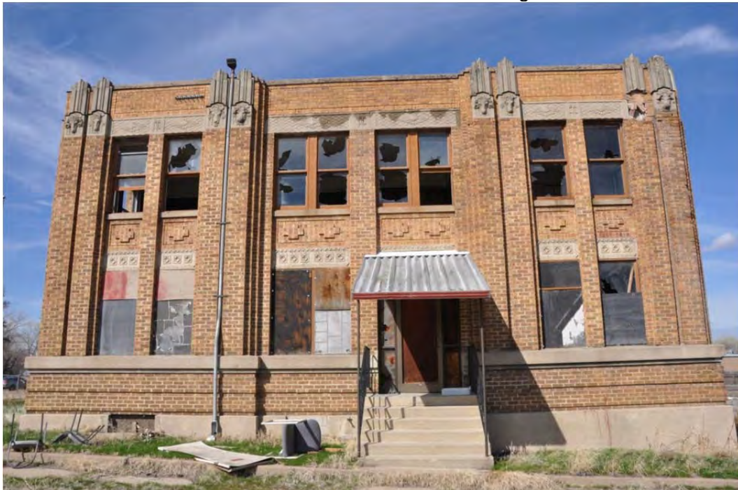
Photograph 2 of 13 East elevation of building. Camera facing west.
