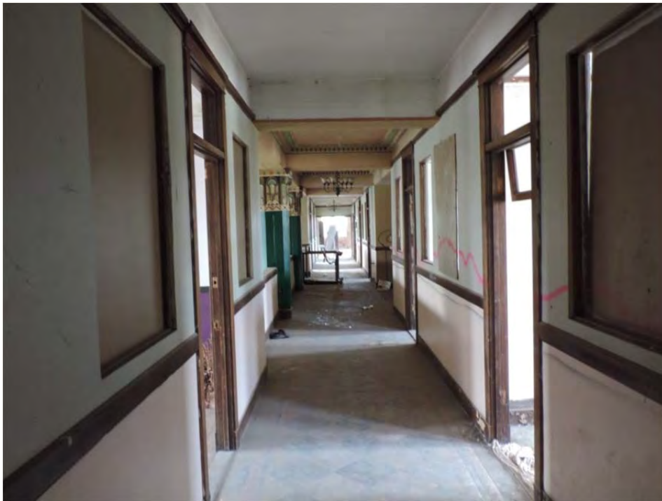
Photograph 12 of 13 Interior detail of the second floor hallway. Camera facing west.
