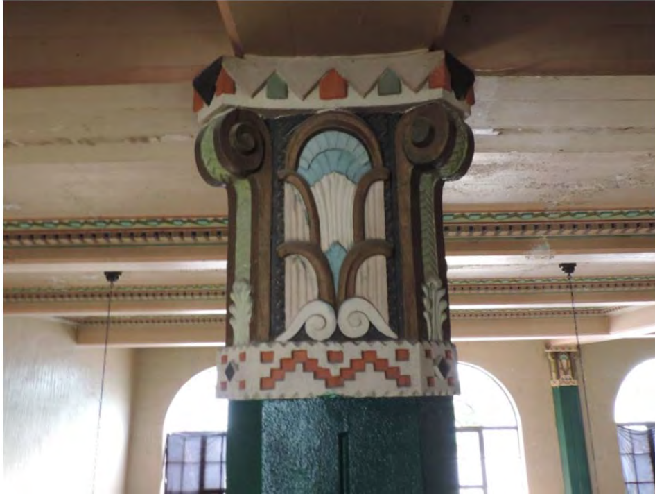
Photograph 11 of 13 Column and ceiling detail in lobby area. Camera facing south.
