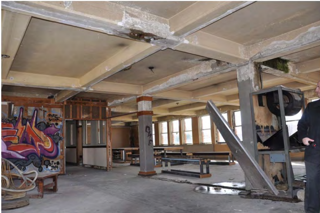
Photograph 13 of 13 West room, second floor. Camera facing southeast.
