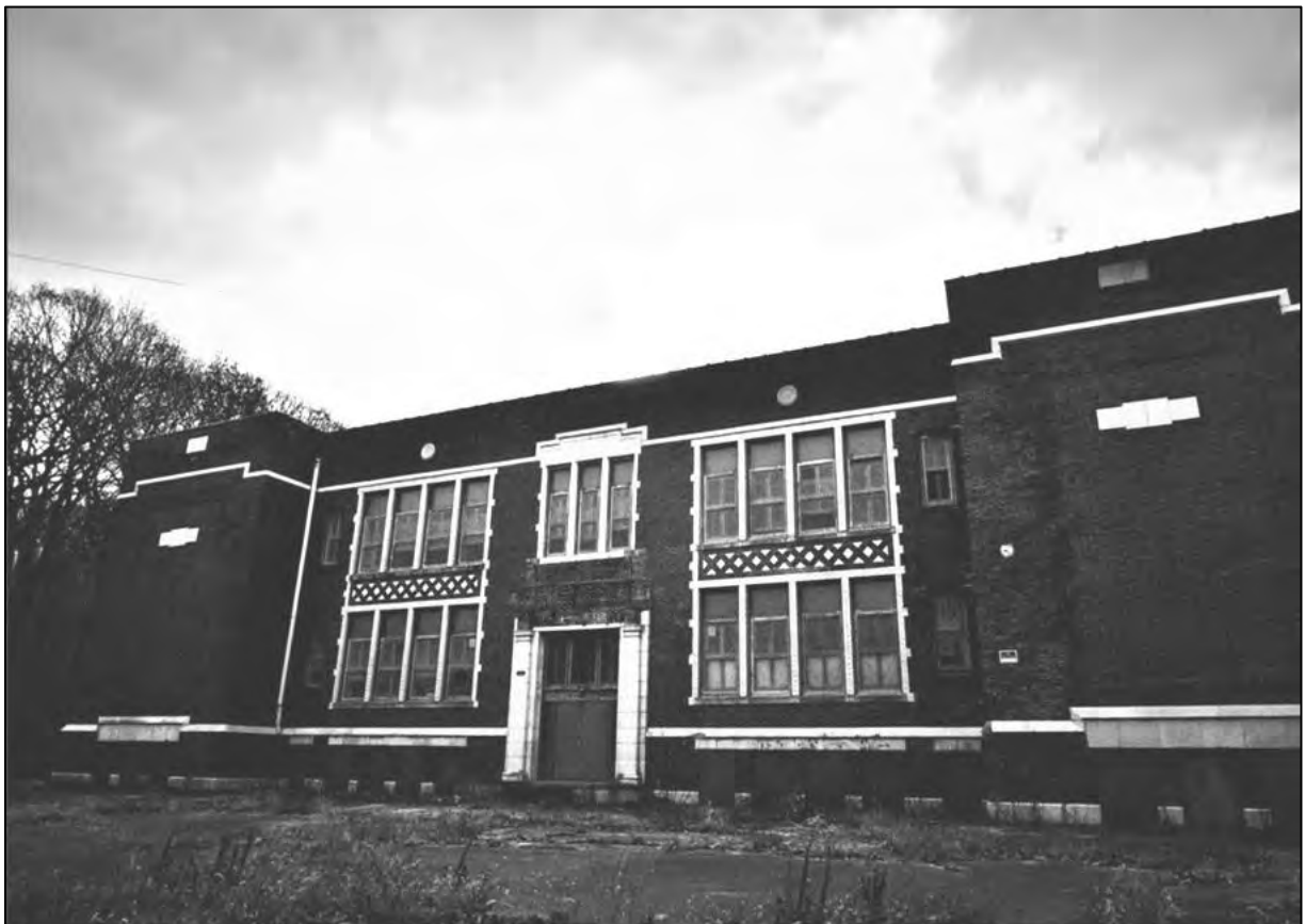
Figure 12: Current photograph (2015) of the McKinley School showing alterations to the original crenelated parapet
