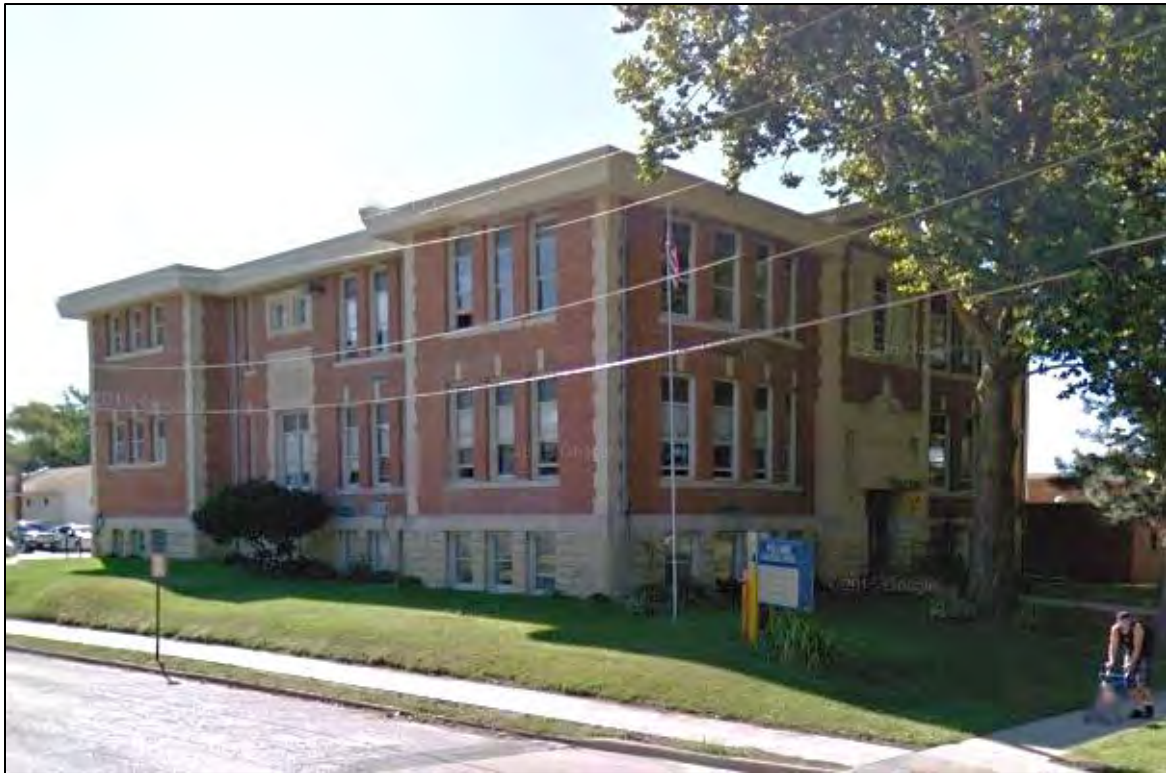
Figure 13: Current photograph (2015) of the Willard School, looking southeast toward the west and north elevations showing the altered roof line and non-historic cornice
