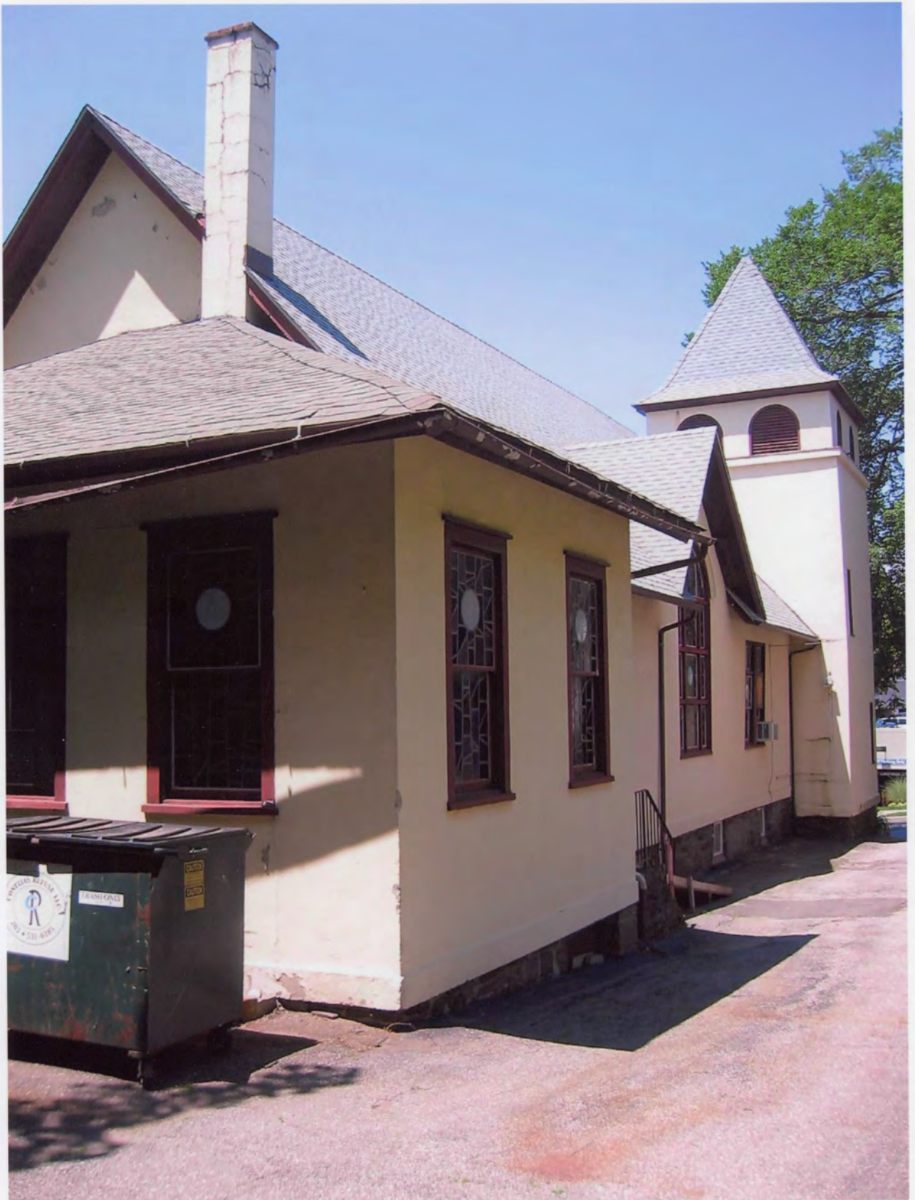
Little Bethel A.M.E. Church Greenwich, Fairfield County, Connecticut Photograph 2 – The building from the southeast. 10 July 2009 James Sexton
