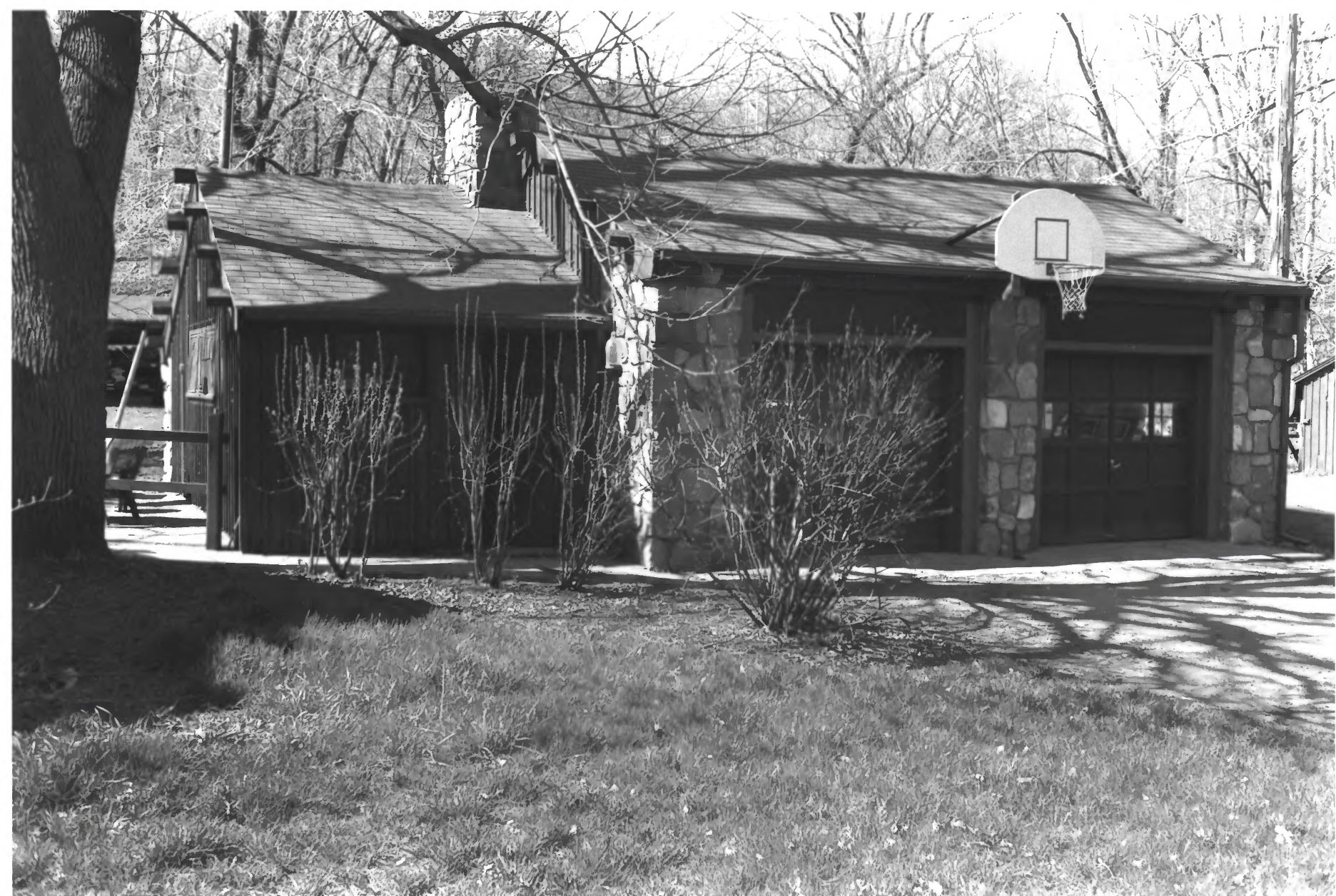
CAMDEN STATE PARK - WAREHOUSE / GARAGE LYON CO. MN BLDG # '11 PHOTO I.D. 09720 # 2
