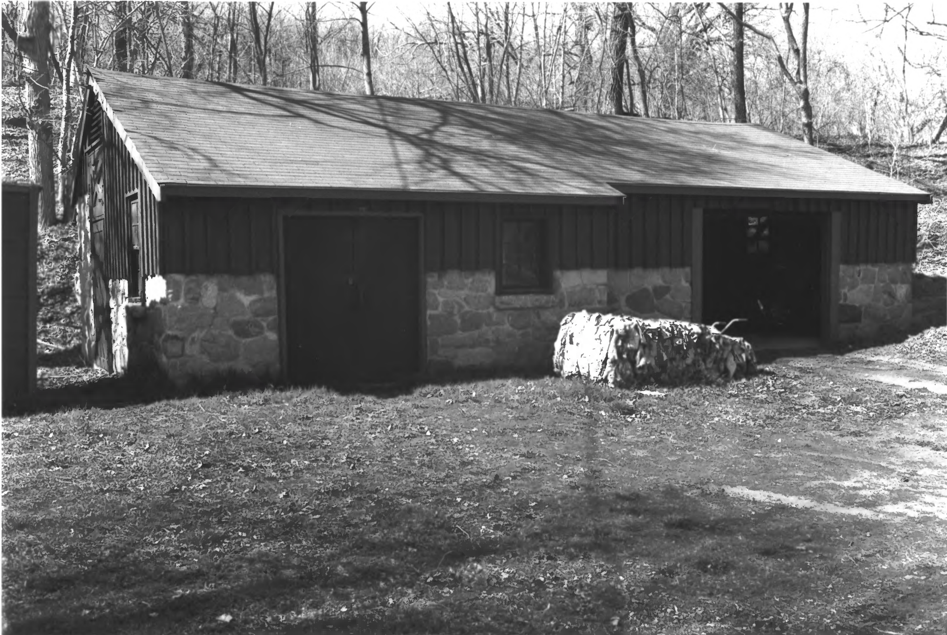
CAMDEN STATE PARK - ICE & WOOD HOUSE LYON CO., MN BLDG #12 PHOTO I.D. 09720 #3
