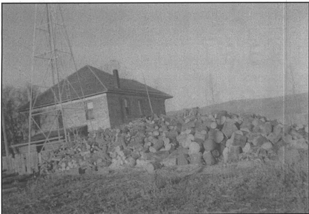
View of the rear of the ranch house showing the tower for the Jacobs wind-powered electrical generating system.
