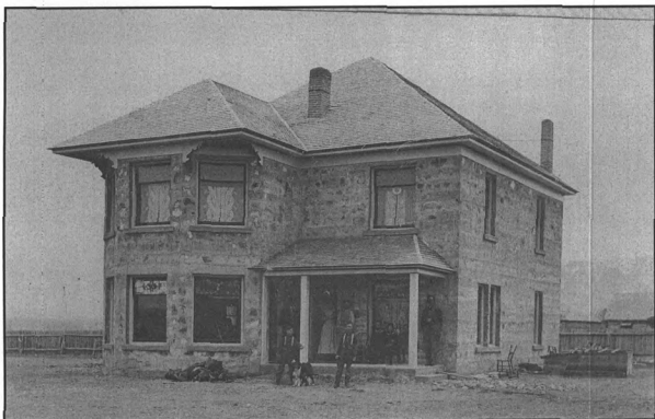
Ranch house after completion.
