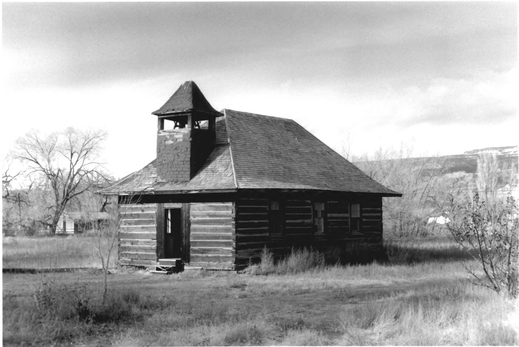
TORREY LOG CHURCH / SCHOOL HOUSE TORREY, WAYNE CO., UT. PHOTO # 1
