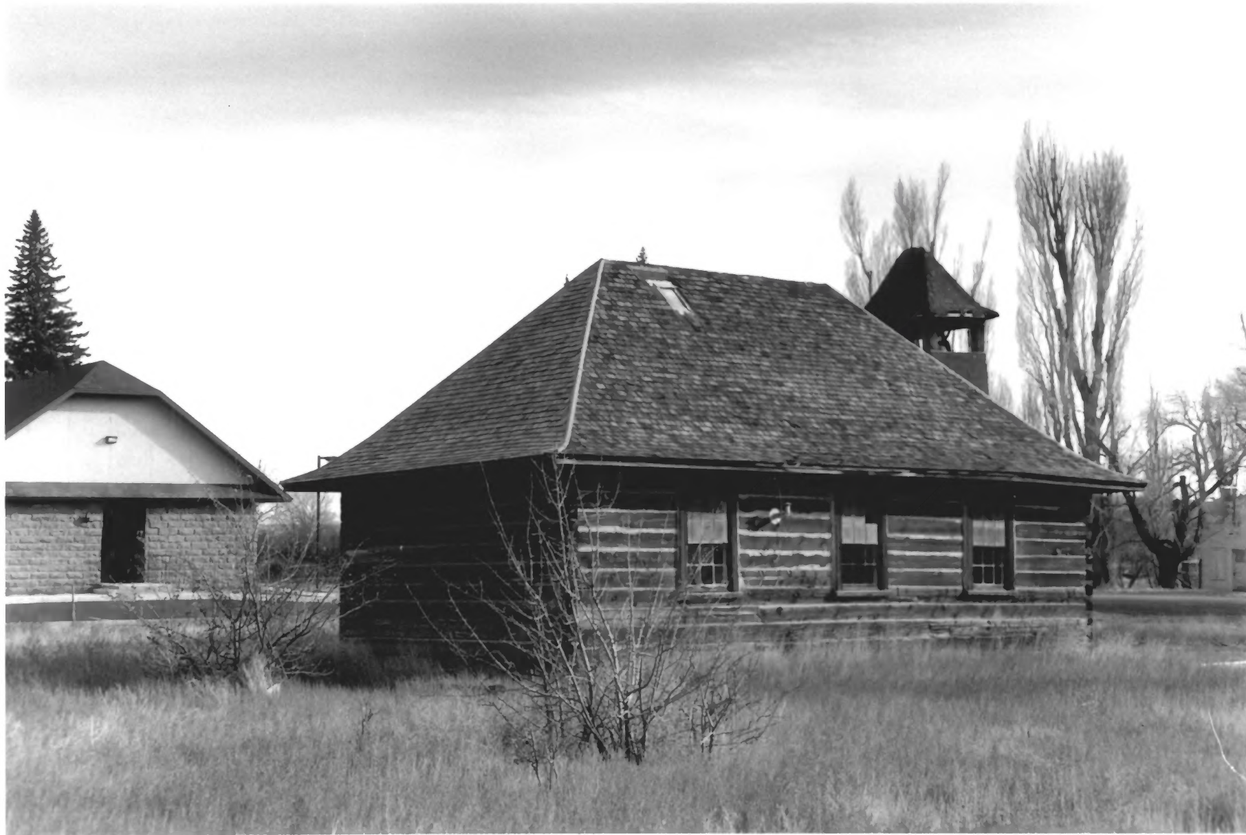
TORREY LOG CHURCH / SCHOOL HOUSE TORREY, WAYNE CO., UT. PHOTO #2
