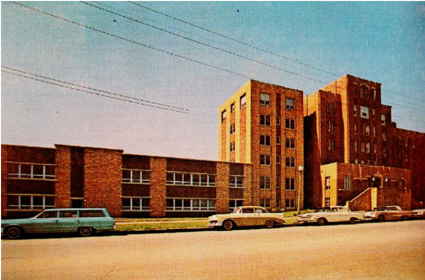
Figure 12 – c.1970 view of 2-story east wing constructed in 1964 (prior to 1979 addition of two floors) Downloaded at website railwaysurgeons.org 2 February 2016.
