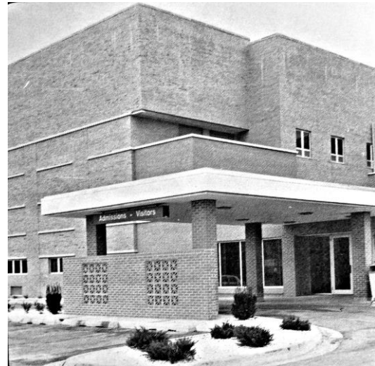
Figure 15 – c.1982 view of last building addition – new Emergency entry at south end of west wing (Undated Memorial Hospital Brochure, Topeka Public Library).
