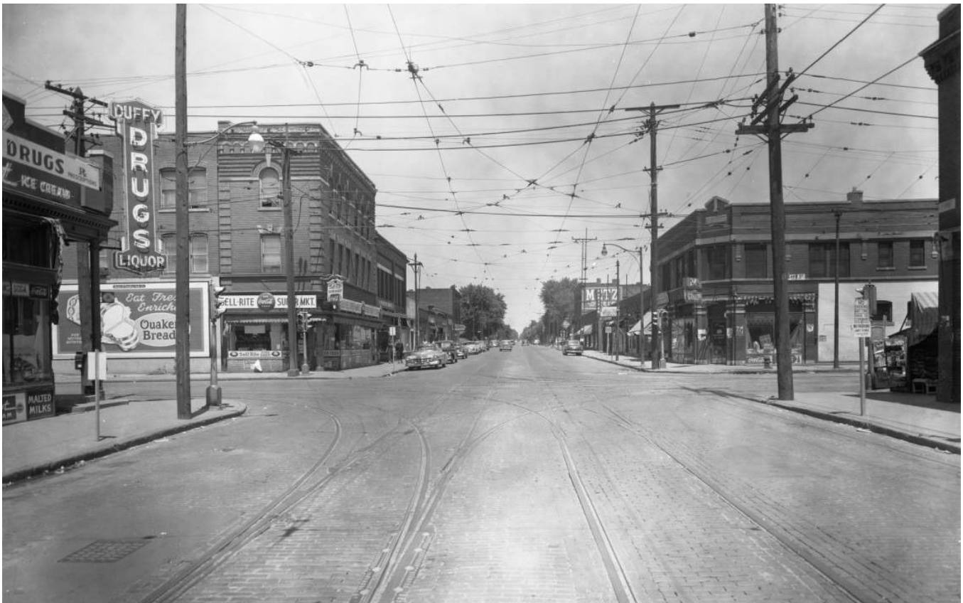
Looking north on North 24 th Street. Lake Street is in the foreground. (1953, June 28). Love plaza now occupies the site of the three-story building on the left, while the buildings on the right were demolished in 1964 to construct the Safeway supermarket parking lot. From the Bostwick-Frohardt collection owned by KMTV on permanent loan to the Durham Museum. Identifier BF6153-890.
