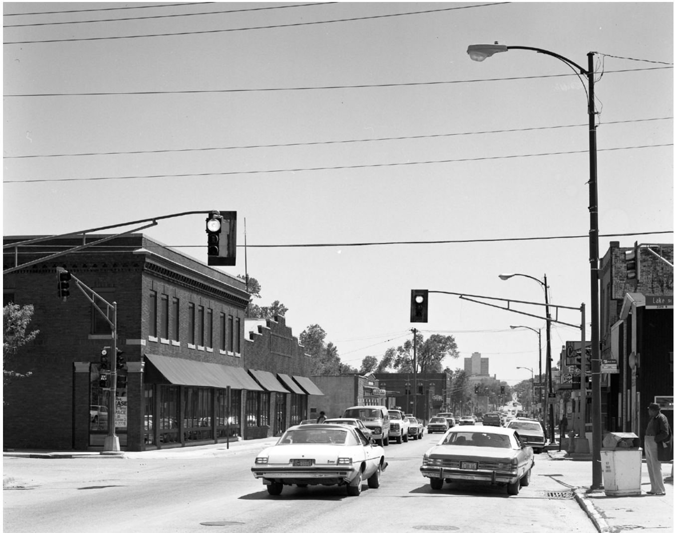
North 24th and Lake Streets looking southeast. Photograph taken by Lynn Meyer. (Circa 1983). Photograph courtesy of City of Omaha.
