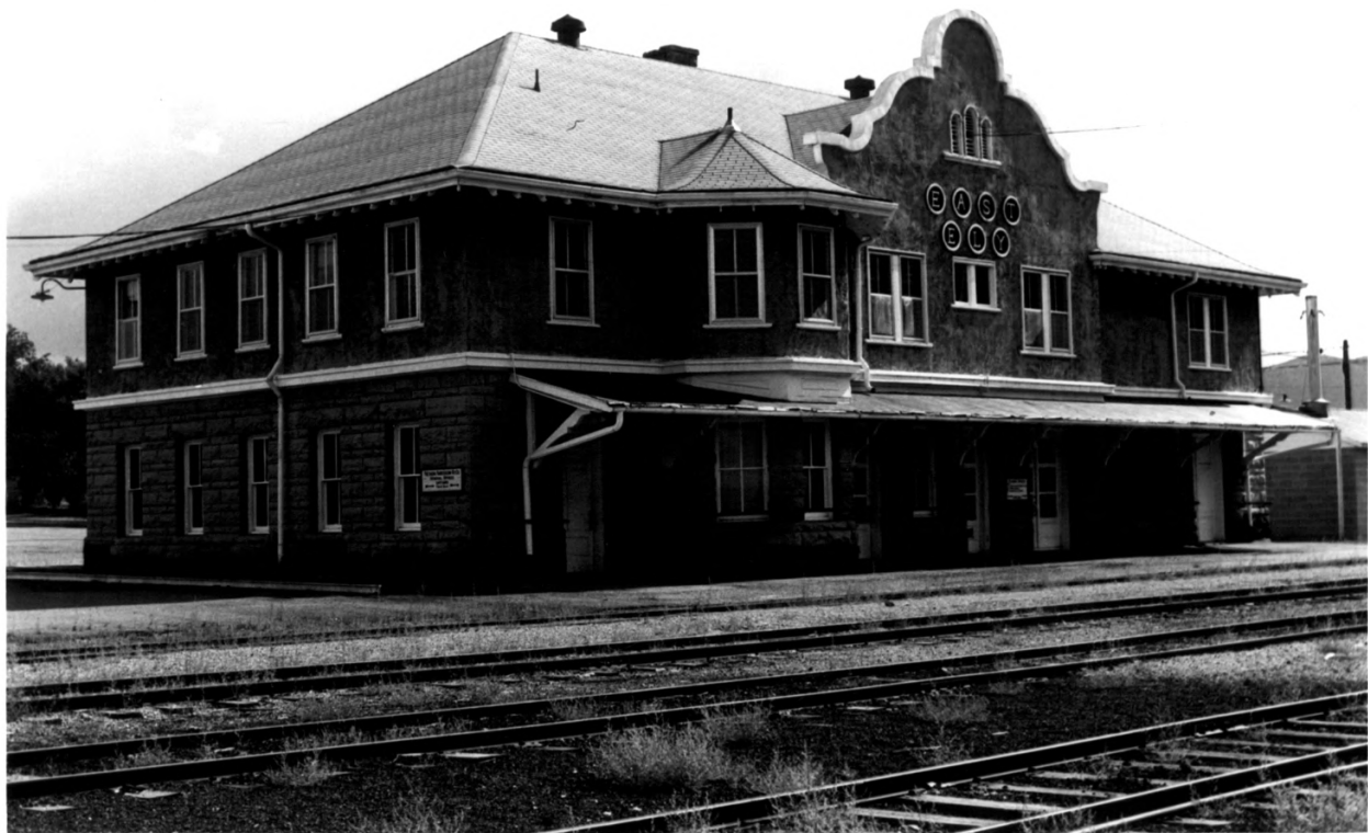
DEPOT BLDG. (S & W. Elevations) EAST ELY YARD - NEVADA NORTHERN RAILROAD
