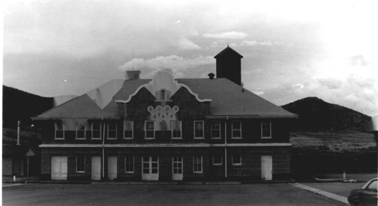
DEPOT BLDG. (S. Elevation) EAST ELY YARD - NEVADA NORTHERN RAILROAD AT 11 th ST. E. KLAMATH - 1983.
