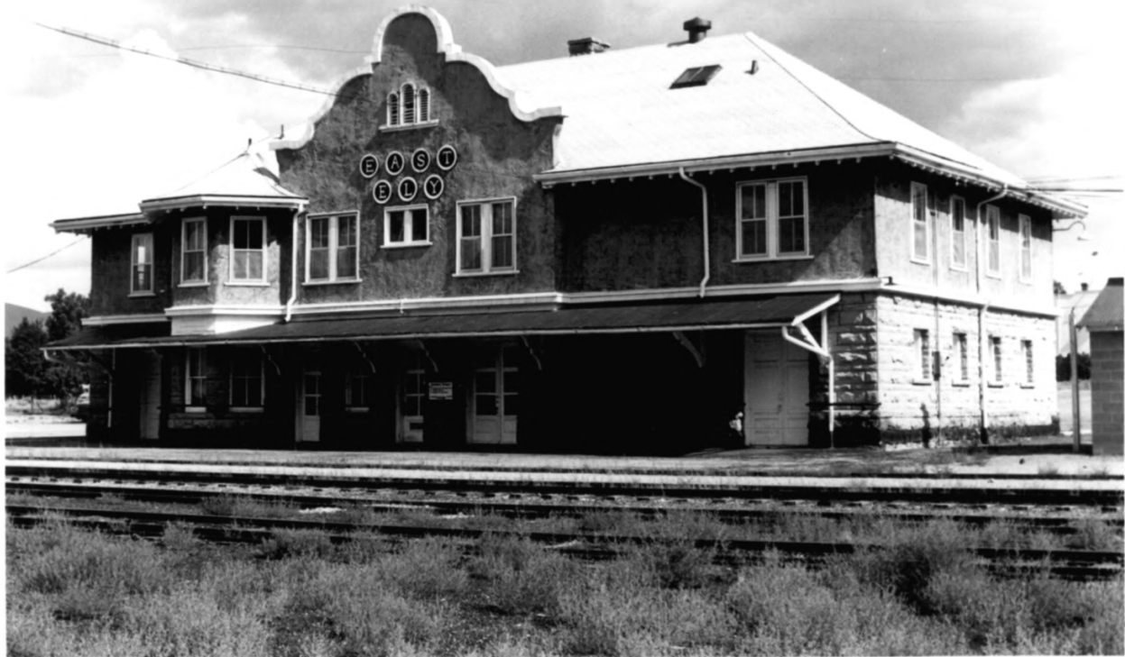
...NT BLDG. (N. & W. Elevations) EAST ELY YARD - NEVADA NORTHERN RAILROAD 1983
