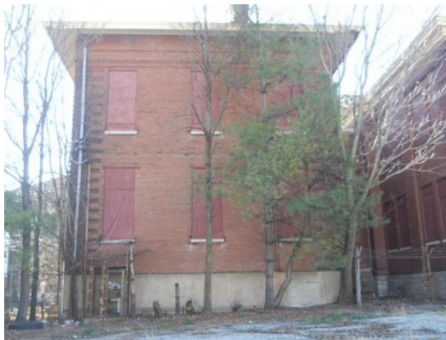
North Façade of 1906 addition
