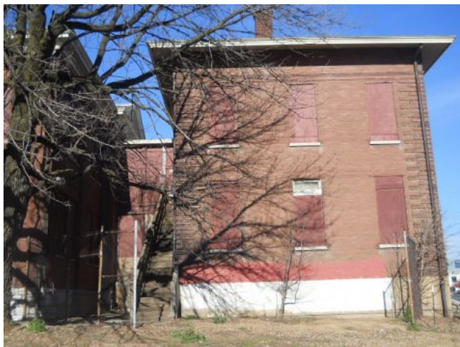
South Façade of 1906 addition
