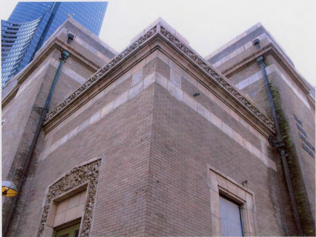
Photo #11 (WA_KingCounty_FirstUnitedMethodistChurch_0011) Exterior Feature – Typical corner pavilion
