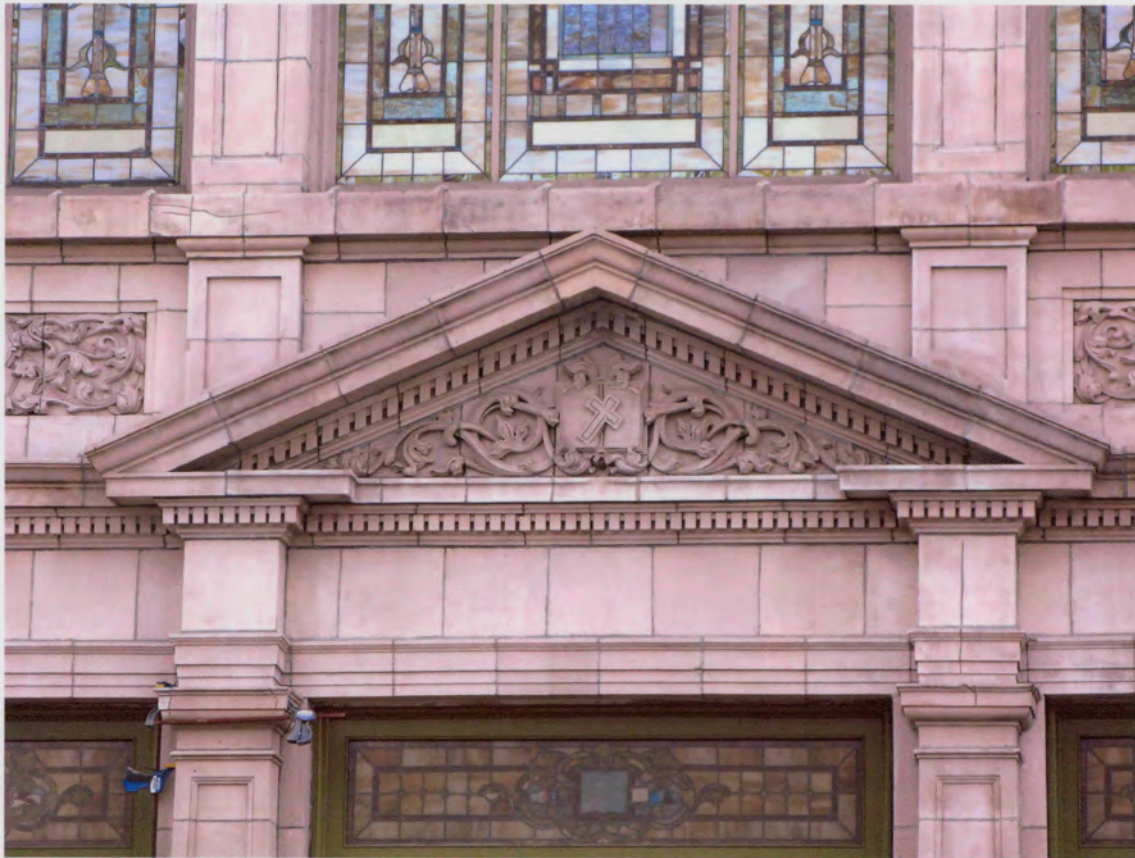
Photo #8 (WA_KingCounty_FirstUnitedMethodistChurch_0008) Exterior Detail – Main Entrance pediment
