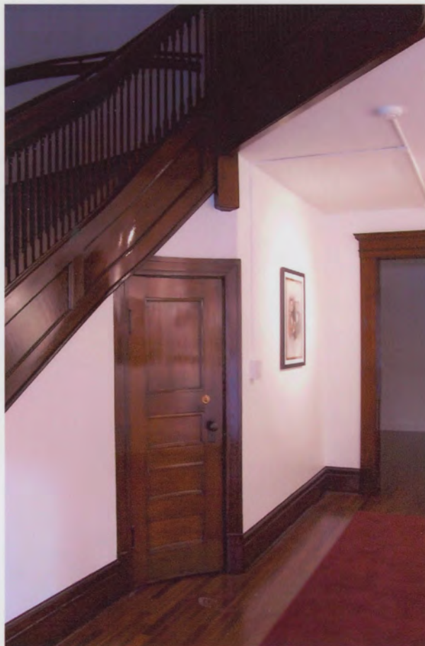
Photo #30 (WA_KingCounty_FirstUnitedMethodistChurch_0030) Marion Street Entrance Vestibule - NW stairwell w/ typical wood flooring & trim
