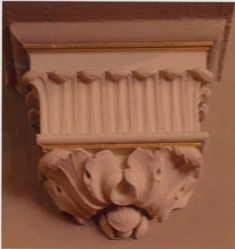
Photo #24 (WA_KingCounty_FirstUnitedMethodistChurch_0024) Main Auditorium – Detail – typical plaster bracket/ornament at gallery beam ends
