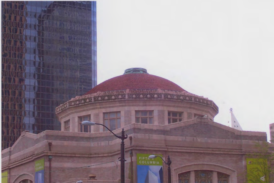
Photo #6 (WA_KingCounty_FirstUnitedMethodistChurch_0006) Exterior Feature – Main Auditorium Dome (K. Krafft 5-16-10)
