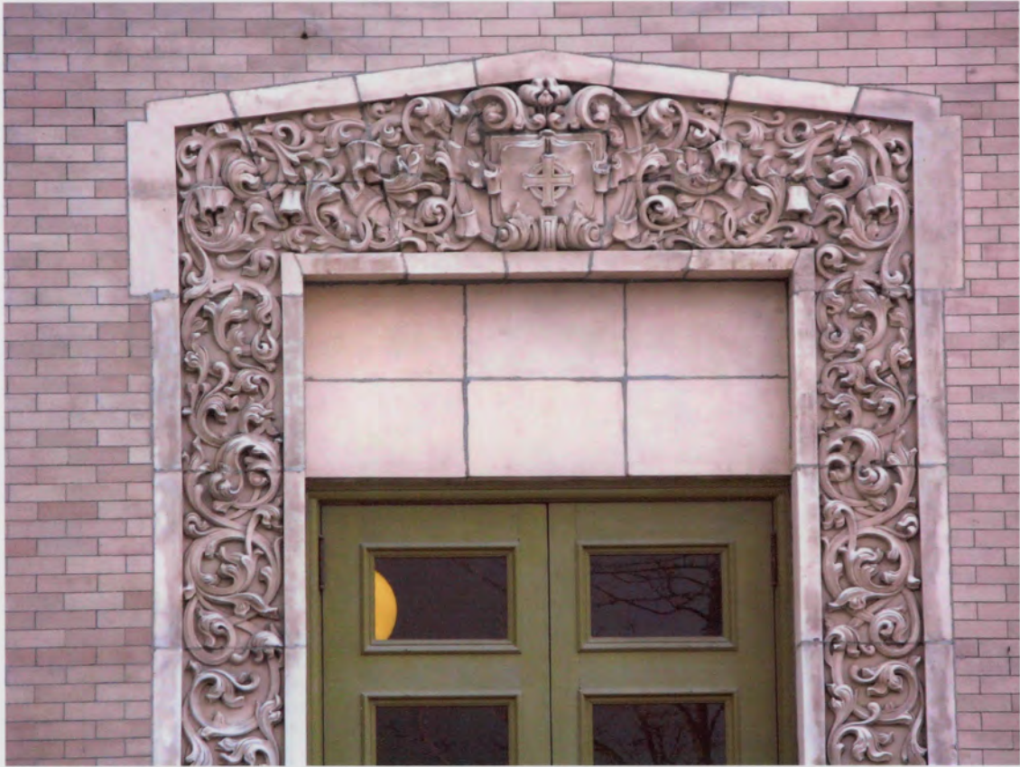
Photo #9 (WA_KingCounty_FirstUnitedMethodistChurch_0009) Exterior Detail – Typical side vestibule entry door surround
