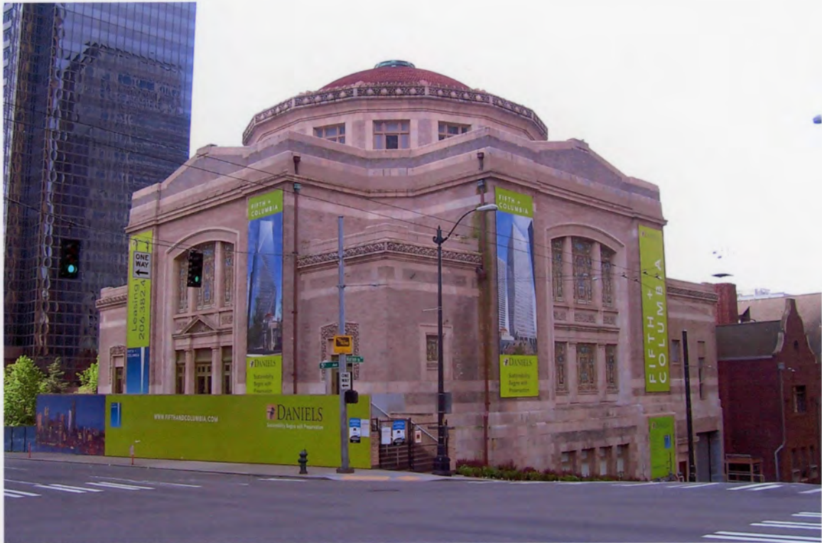
Photo #3 (WA_KingCounty_FirstUnitedMethodistChurch_0003) East & North Elevations (K. Krafft 5-16-10)
