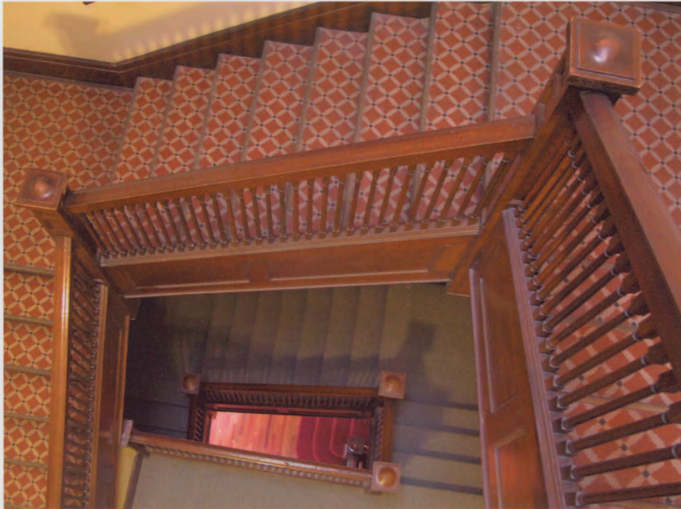
Photo #29 (WA_KingCounty_FirstUnitedMethodistChurch_0029) NW Stairwell – Typical handrails & linoleum flooring
