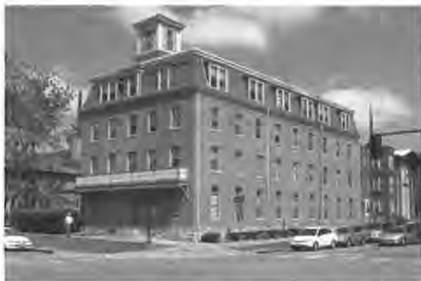
Figure 13 Park House in 2009. According to its National Register nomination, the mansard roof (suggesting the Second Empire style) was added around 1875. Photo by William E. Whittaker and used with permission.
