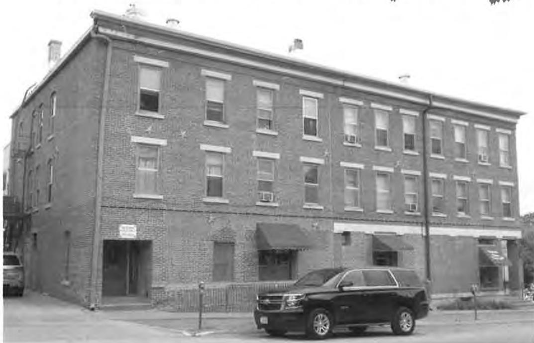
Figure 4 - Westside alley elevation and long southside Market Street elevation. The four upper level windows on the left are in the 1893 rear L addition.
