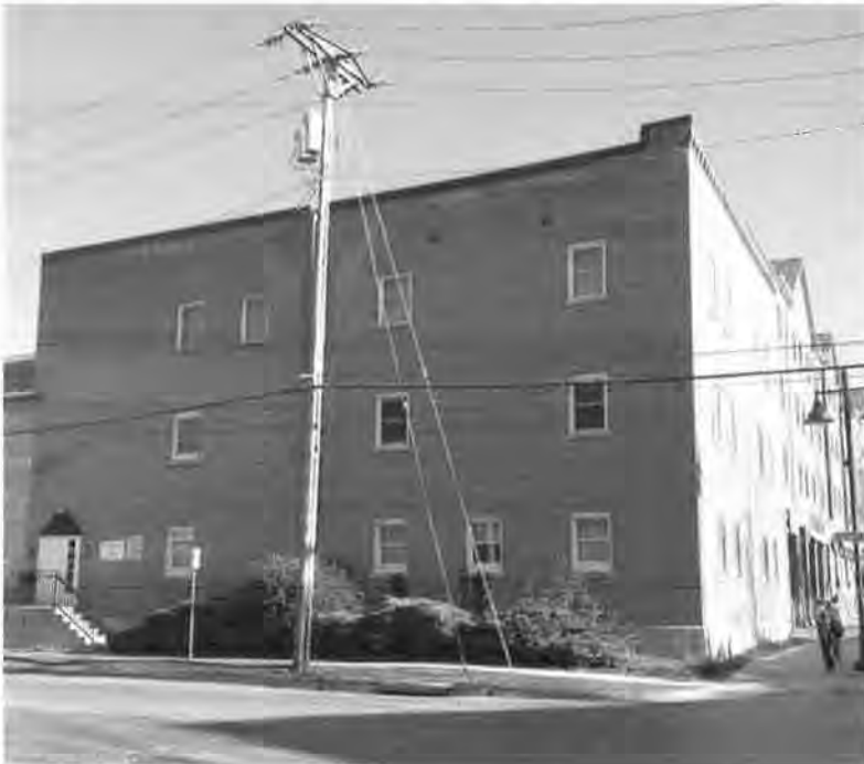
Figure 17 The Iowa City Mills building is severely plain and utilitarian in form. The only decorative detail is found at the façade's roofline where there is a narrow band of brick corbelling. The building now houses a law firm on the ground floor and probably student apartments on the upper levels. Image looks northwest. Court Street is to the bottom of the image; Gilbert Street just off camera to the right.
