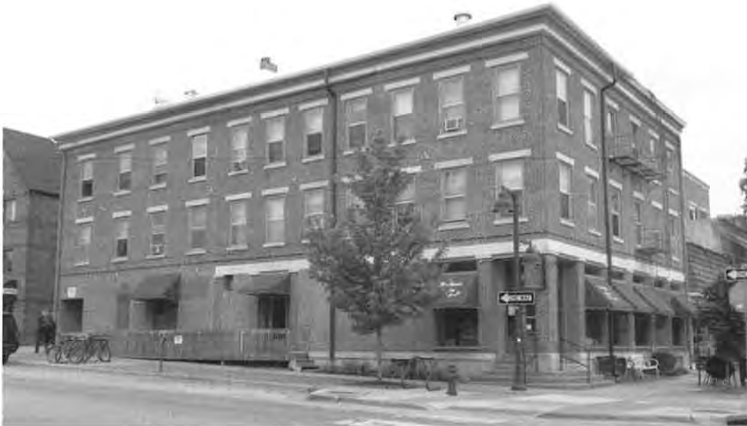
Figure 3 – The seven windows from the corner to the left (west) are part of the c. 1862 original building.
