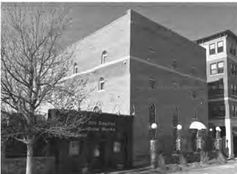
Figure 18 This building is the sole surviving building of the M.T. Close & Co. linseed oil works (though the factory owner's residence is extant across the street) and functioned as a warehouse. The top floor, denoted by the darker brick color, was added in recent years. Image looks northwest and is from Google.maps on 7/1/2015.
