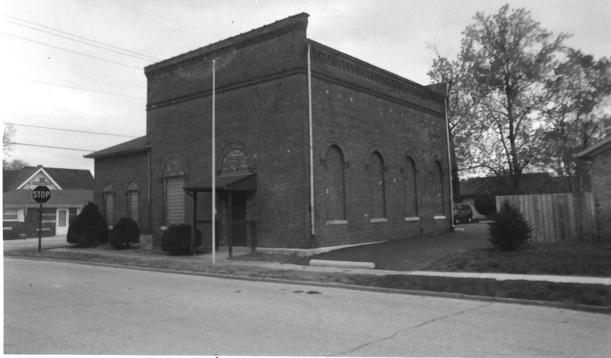
T.H.I. & E. INTERURBAN DEPOT/SUBSTATION HENDRICKS COUNTY, INDIANA
