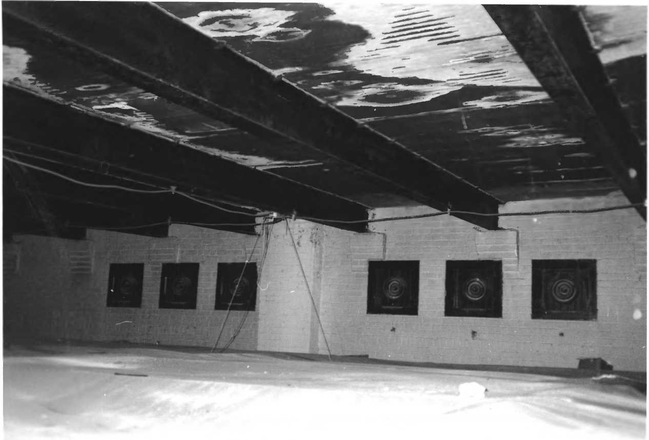
T.H.I. & E. INTERURBAN DEPOT/SUBSTATION
