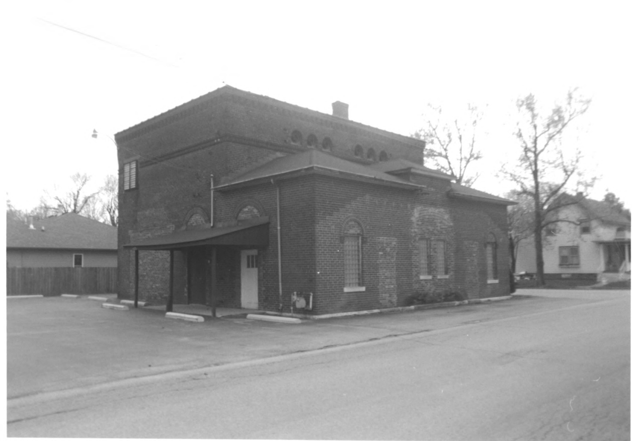
T.H.I. & E. INTERURBAN DEPT / SUBSTATION HENDRICKS COUNTY, INDIANA #4
