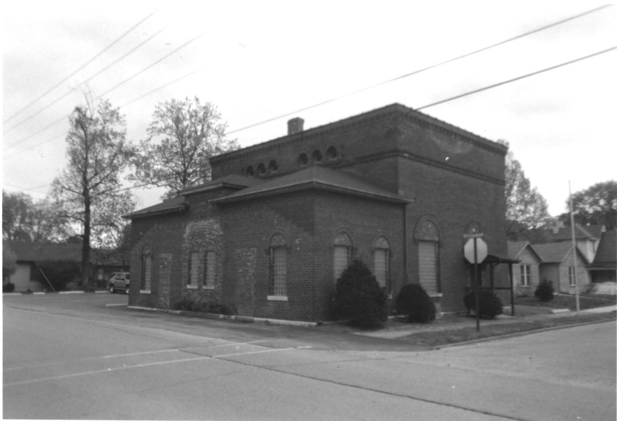
T.H.I. & E. INTERURBAN DEPT/SUBSTATION, HENDRICKS COUNTY, INDIANA #1
