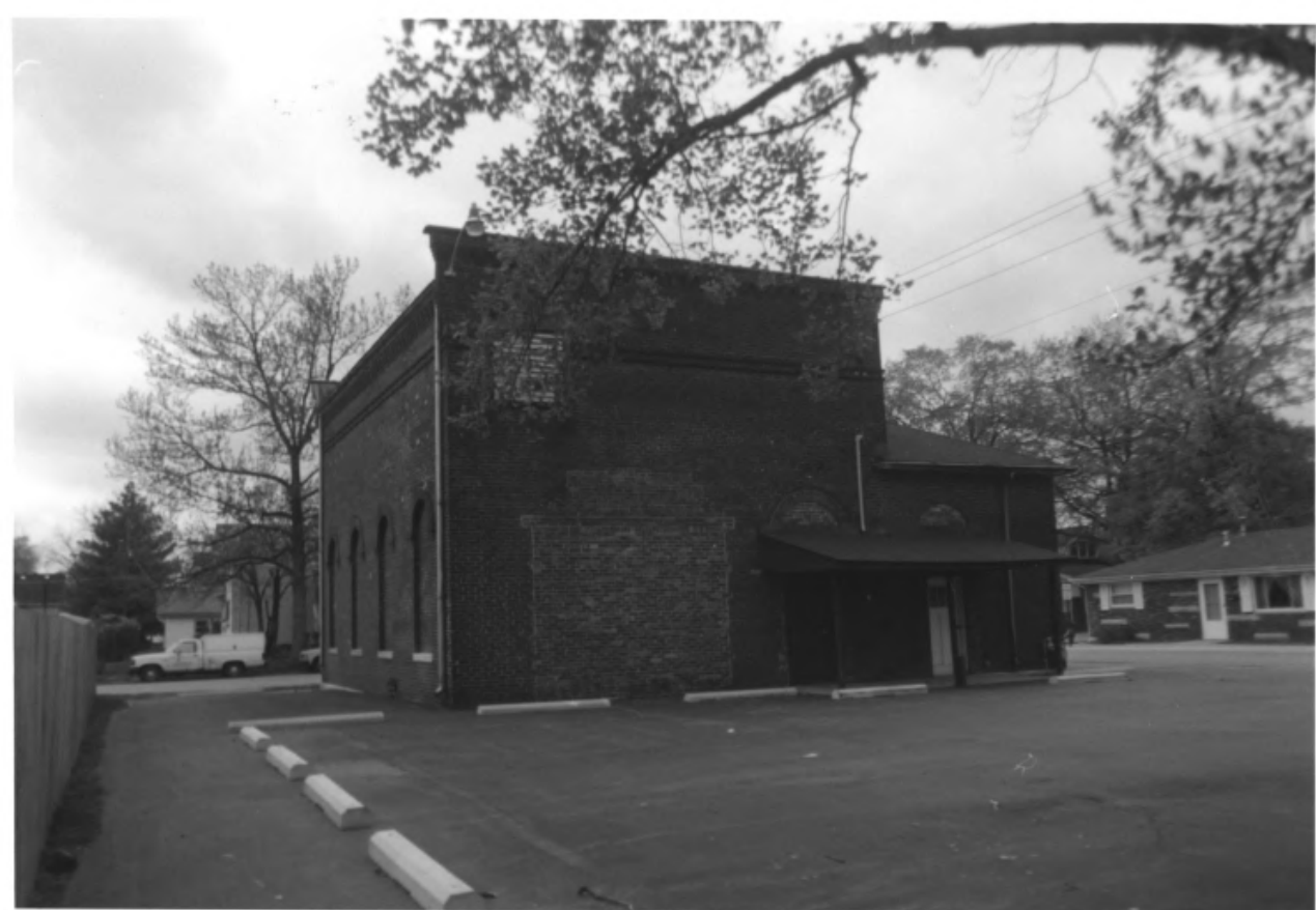
T.H.I. & E. INTERURBAN DEPOT/SUBSTATION, HENDRICKS COUNTY, INDIANA
