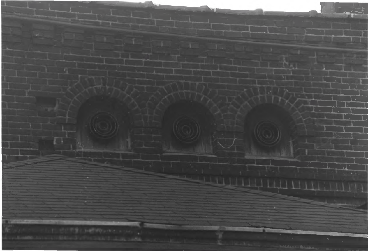
T.H.I. & E. INTERURBAN Depot/SUBSTATION HENDRICKS COUNTY, INDIANA #5
