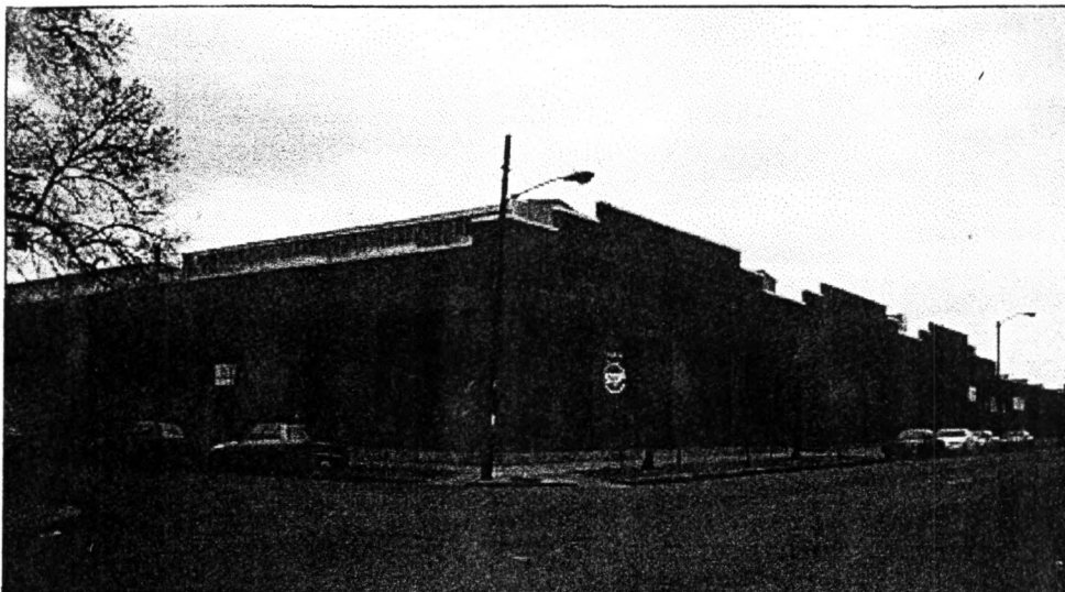
Taken from 36th Avenue and Franklin Street, this view shows the three bays of the 1947 addition connecting along Franklin with the 1937 addition. Photographer: Nancy L. Widmann.
