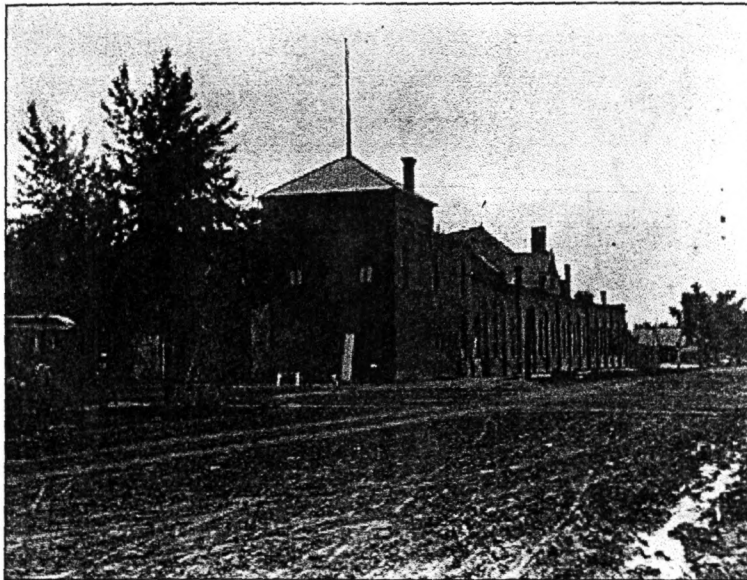
The East Division Car Barn, 35th and Gilpin Street, on 15 May 1904. Dirt streets held the tracks. The roof of Hyde Park School, now Wyatt School, is seen above the barn. A streetcar is leaving the barn at the left of the photograph. Source: Denver Tramway Collection, Colorado Railroad Museum, Golden, Colorado.
