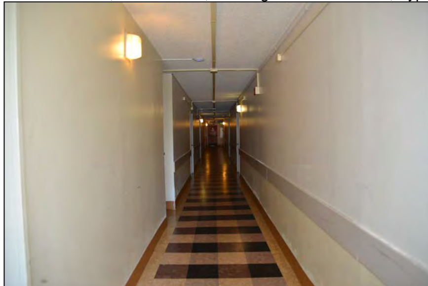
Photo 10. Interior, Fourth Floor, Looking West at Corridor, Typical
