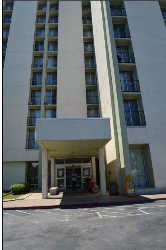
Photo 5. Exterior, North Elevation, Looking South at Entrance
