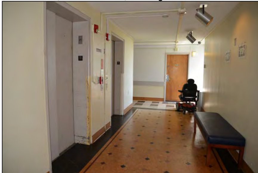
Photo 16. Interior View, Eleventh Floor, Looking North at Elevator Lobby, Typical
