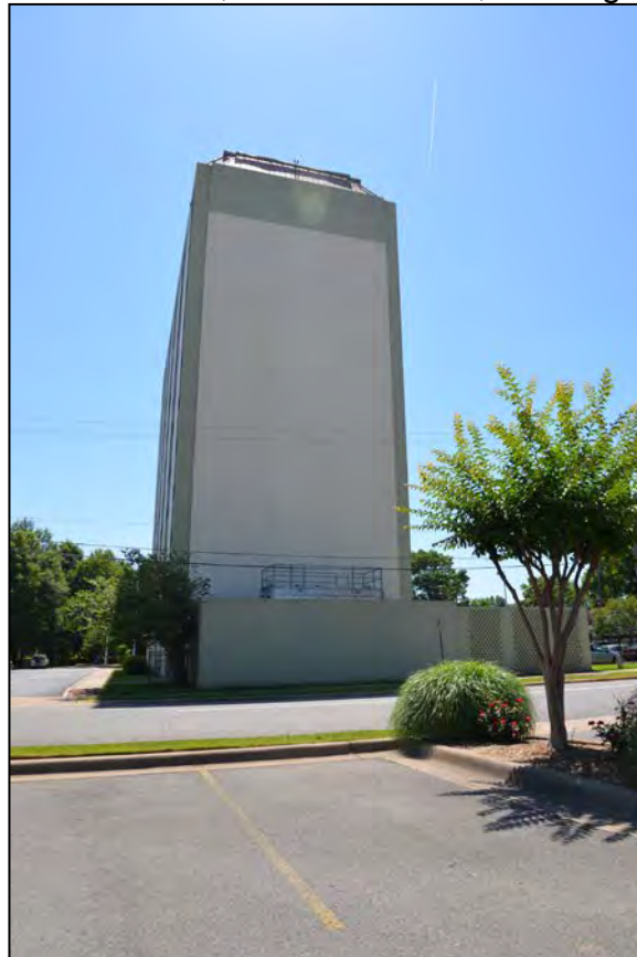
Photo 2. Exterior, West Elevation, Looking East
