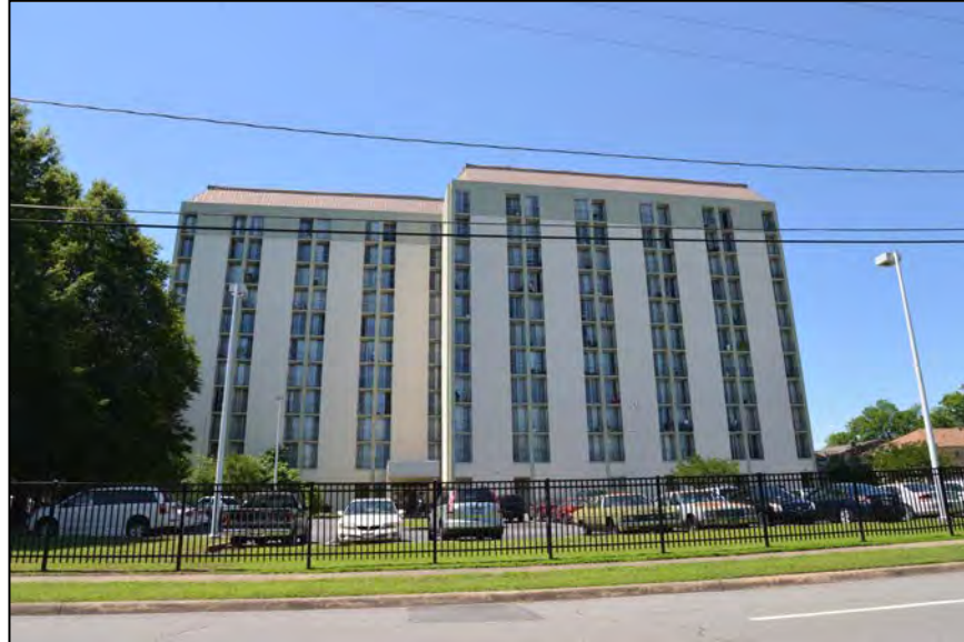
Photo 1. Exterior, North Elevation, Looking South
