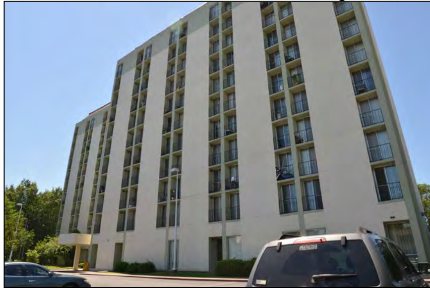
Photo 3. Exterior, North Elevation, Looking South
